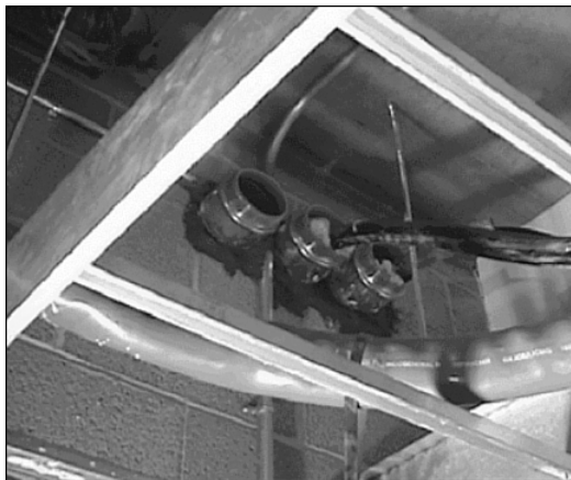
Figure A-36 Typical Firewall Penetration
