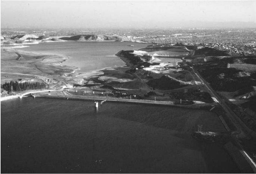
FIGURE 2.23 Aerial view of Lower San Fernando Dam and San Fernando Valley. (Photograph courtesy of Steinbrugge Collection, Earthquake Engineering Research Center, University of California, Berkeley.)
