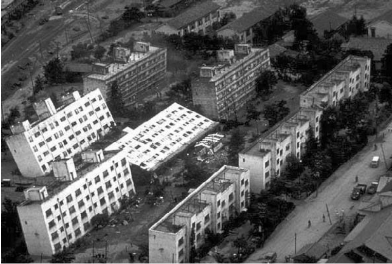
FIGURE 2.4 Liquefaction caused building failure in Niigata, Japan. (Photo by Joseph Penzien; photo courtesy of Steinbrugge Collection, Earthquake Engineering Research Center, University of California, Berkeley.)
