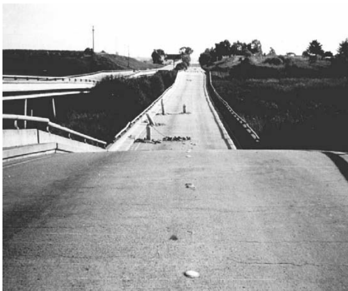
FIGURE 2.26 Piles penetrating bridge deck.
