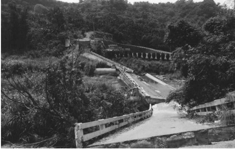
FIGURE 2.33 Three-span bridge rocked over during the 1999 Ji Ji, Taiwan, earthquake.
