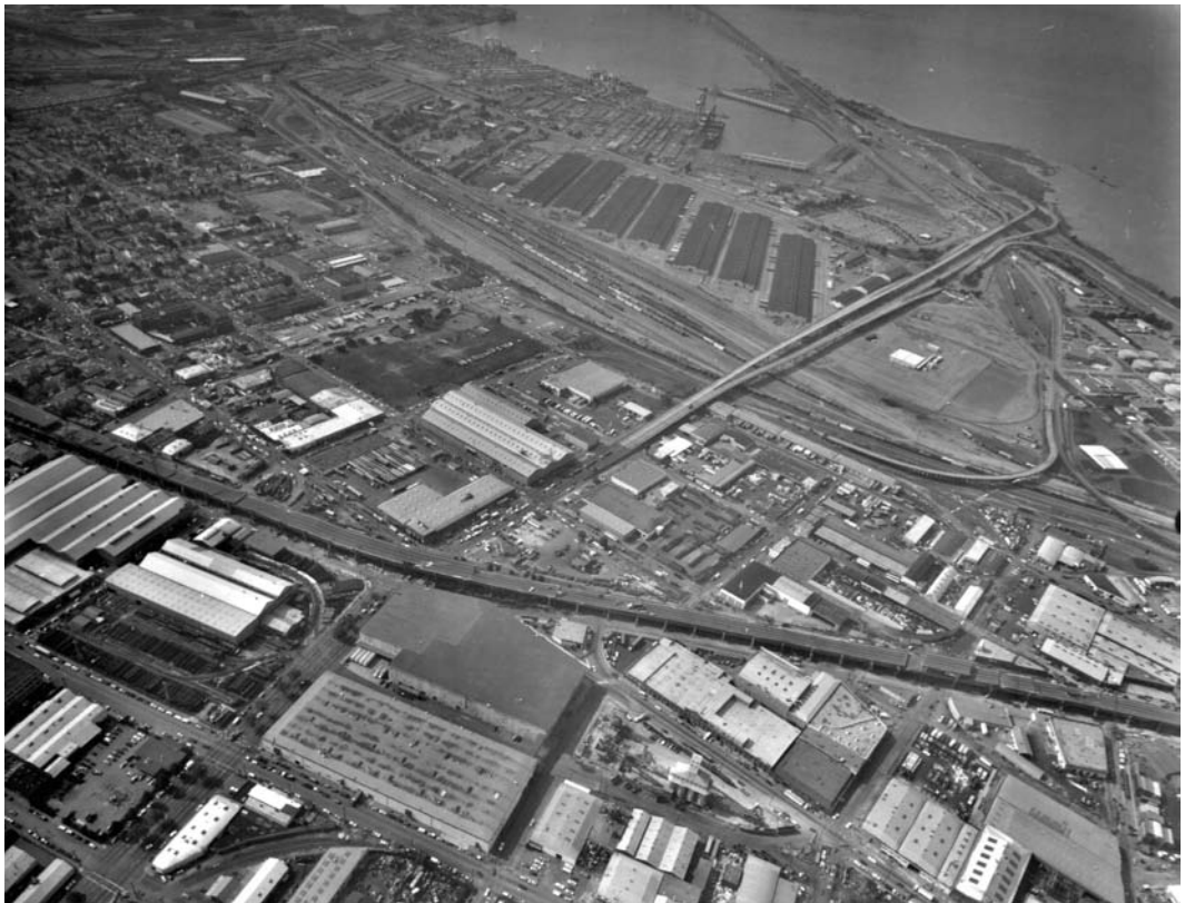
FIGURE 2.29 Aerial view of Cypress Viaduct showing collapse where the structure crossed over Bay mud.
