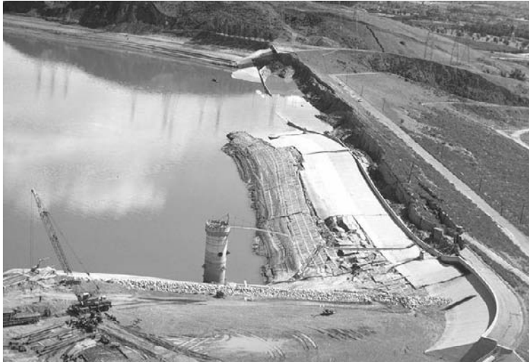
FIGURE 2.21 Damage to the Lower San Fernando Dam. (Photograph courtesy of Steinbrugge Collection, Earthquake Engineering Research Center, University of California, Berkeley.)
