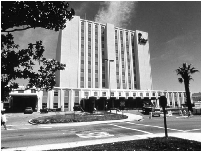
FIGURE 2.84 The existing Long Beach VA Hospital was seismically retrofit with lead-rubber bearings. (Photo courtesy of Dynamic Isolation Systems, Inc.)
