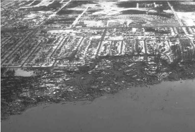
FIGURE 2.17 Aerial view of Turnagain Slide. (Photograph courtesy of Steinbrugge Collection, Earthquake Engineering Research Center, University of California, Berkeley.)
