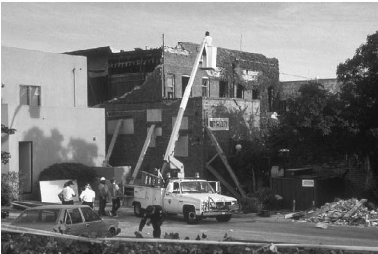
FIGURE 2.61 Rear view of damaged unreinforced masonry (URM) building facing Pacific Garden Mall, Santa Cruz Area, California. (Photo by James R. Blacklock, Loma Prieta Collection, Earthquake Engineering Research Center, University of California, Berkeley.)
