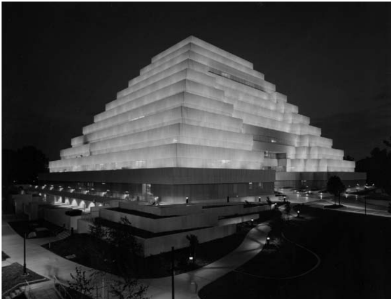
FIGURE 2.81 The uniquely shaped "Money Store" was designed with fluid viscous dampers to improve its seismic behavior. (Photo courtesy of Marr-Shaffer & Miyamoto, Structural Engineers.)
