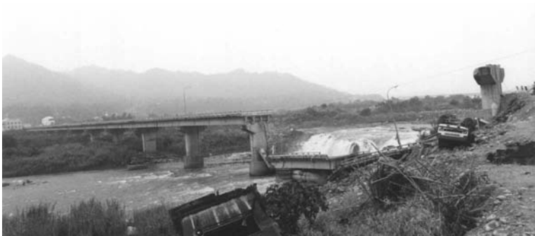
FIGURE 2.67 The Dajia River bridge and 6-m fault scarp.
