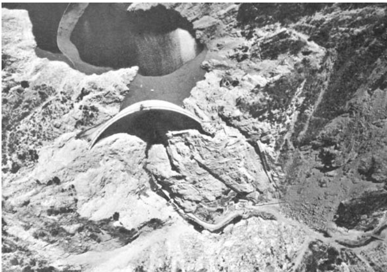
FIGURE 2.20 Landslides at Pacoima Dam following the 1971 San Fernando Earthquake. (Photograph courtesy of Steinbrugge Collection, Earthquake Engineering Research Center, University of California, Berkeley.)
