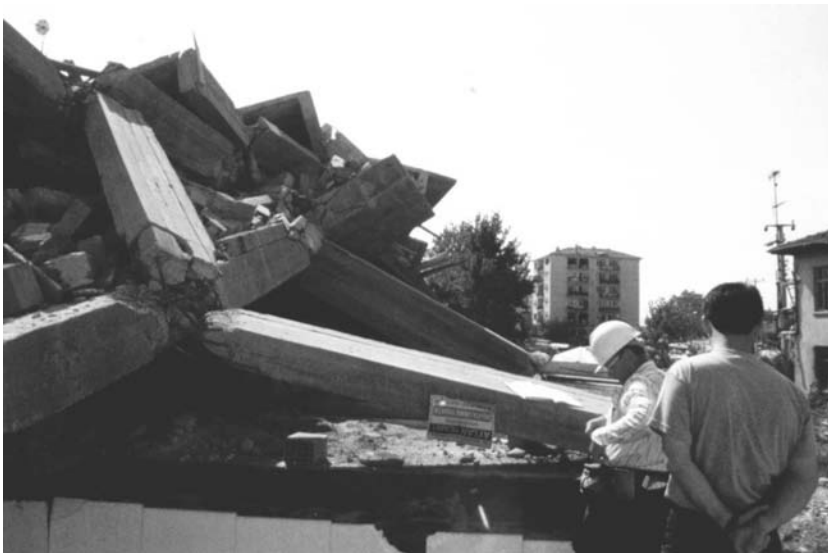
FIGURE 2.59 Collapsed reinforced concrete building during the 1999 Kocaeli Earthquake.
