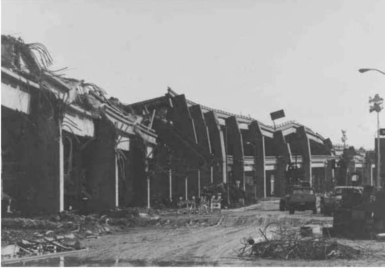
FIGURE 4.4 Collapse of Cypress Viaduct, California, in the 1989 Loma Prieta Earthquake.
