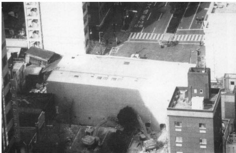
FIGURE 2.42 Eventual collapse of nine-story SRC building after the Kobe Earthquake. (Photo courtesy of NIST; NIST, The January 17, 1995 Hyogoken-Nanbu (Kobe) Earthquake, U.S. NIST, Gaithersburg, MD, 1996.)
