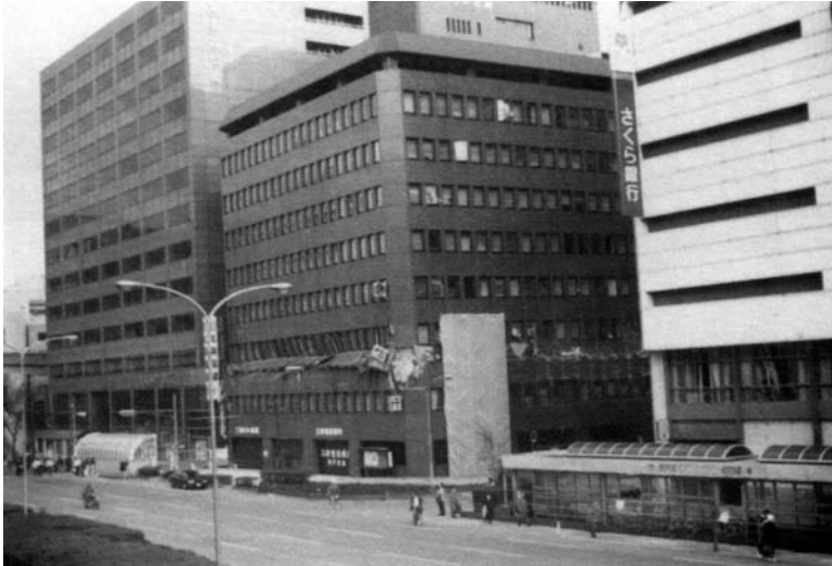
FIGURE 2.39 Ten-story SRC building with third floor collapse during the Kobe Earthquake. (Photo courtesy of NIST; NIST, The January 17, 1995 Hyogoken (Kobe) Earthquake, U.S. NIST, Gaithersburg, MD, 1969.)
