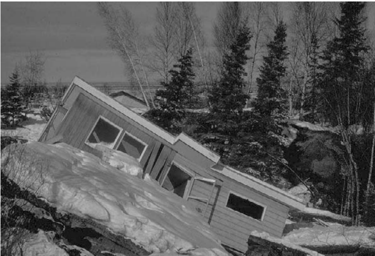
FIGURE 2.18 About 75 homes were damaged as a result of the Turnagain Heights Slide. (Photograph courtesy of Steinbrugge Collection, Earthquake Engineering Research Center, University of California, Berkeley.)
