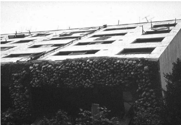
FIGURE 2.5 Liquefaction caused building failure in Niigata, Japan. (Photo by Joseph Penzien; photo courtesy of Steinbrugge Collection, Earthquake Engineering Research Center, University of California, Berkeley.)
