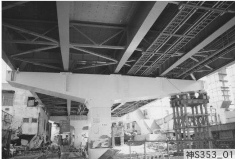
FIGURE 2.68 Collapsed building leaning against the Kobe Route 3 Expressway. (Photo courtesy of Hanshin Expressway Public Corporation.)
