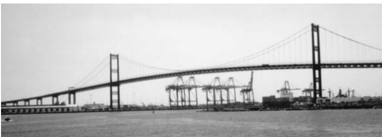
FIGURE 2.87 The Vincent Thomas Bridge is a three-span suspension structure built over the port of Los Angeles.
