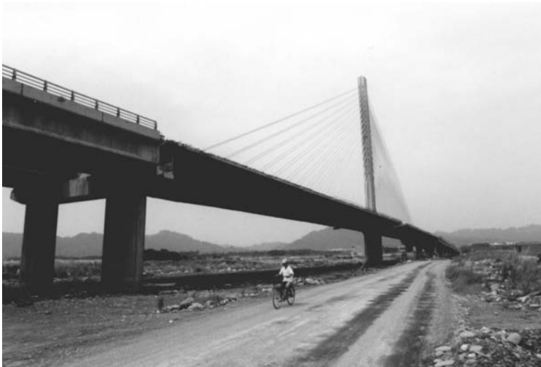
FIGURE 2.44 The Ji Lu cable-stayed bridge after the 1999 Ji Ji, Taiwan, earthquake.
