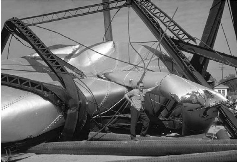
FIGURE 2.62 California Water Service 150,000-gal tank on six legs; the typical failure of tanks is upside down, with riser on top (Bakersfield, California, photo by Karl V. Steinbrugge, Steinbrugge Collection, slide/image No. S64, photo date July 25, 1952, Kern County, California, earthquake, July 21, 1952, magnitude 7.69; courtesy of Steinbrugge Collection, Earthquake Engineering Research Center, University of California, Berkeley).
