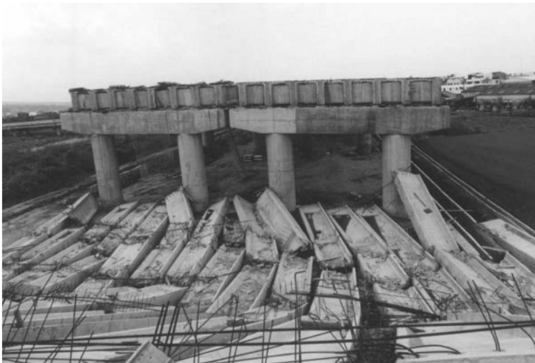
FIGURE 2.63 Collapsed precast, prestressed “I” girders during construction of new expressway in Taiwan due to the 1999 Ji Ji, Taiwan, earthquake.
