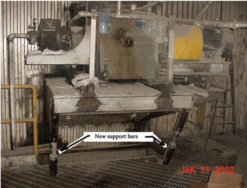
FIGURE 12.7 Air preheater drive/platform with overhang support bars.
