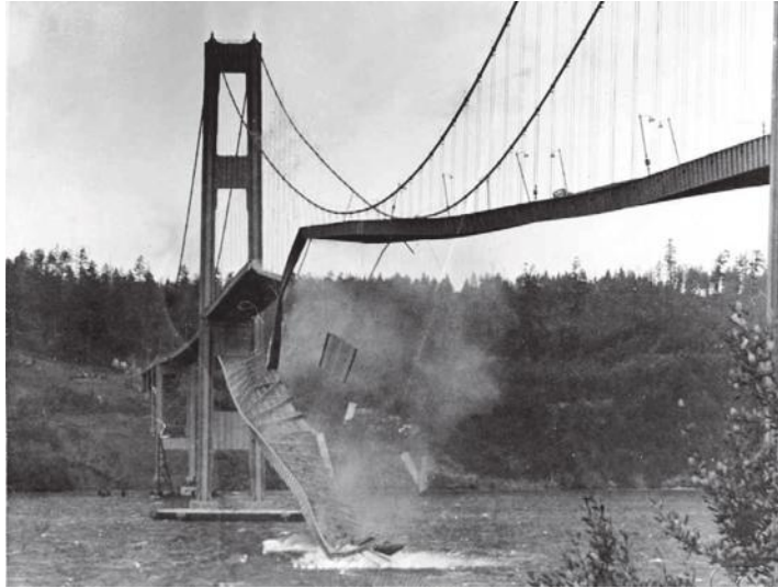
FIGURE 18.1 Tacoma Narrows Bridge collapse. Source: University of Washington Libraries, Special Collections, UW 21422.
