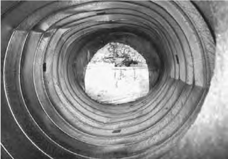
Figure 6.17 Inside pipe at completion of test 3. The cover height is 110 ft.
