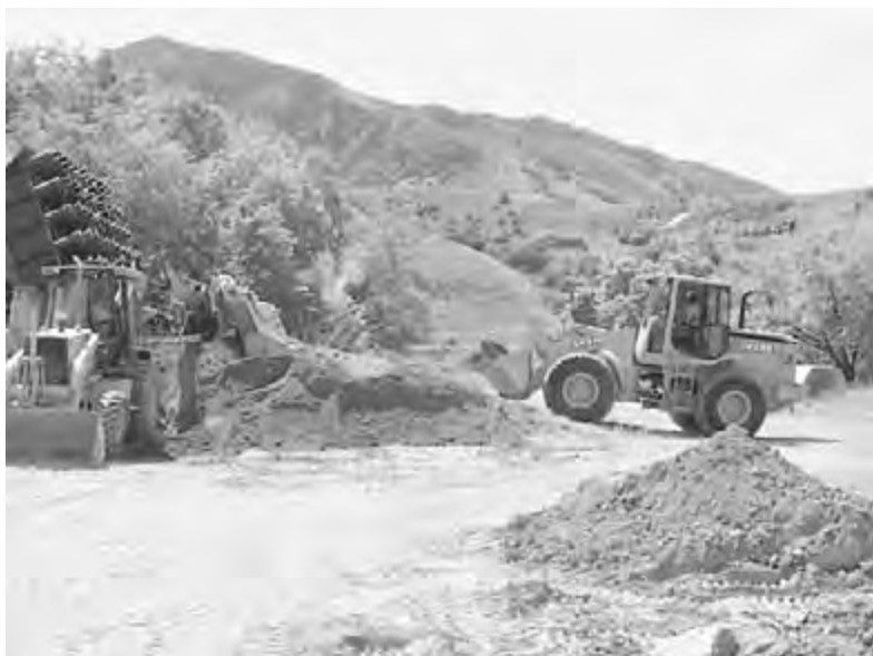
Figure 7.59 Soil placement process.
