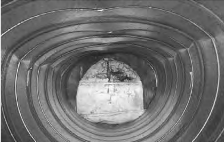
Figure 6.14 Inside the pipe after completion of test (40 ft of cover).
