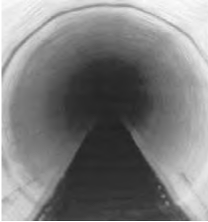
Figure 8.14 A 24-in-diameter pipe after relining. (Courtesy of Ultraliner.)
