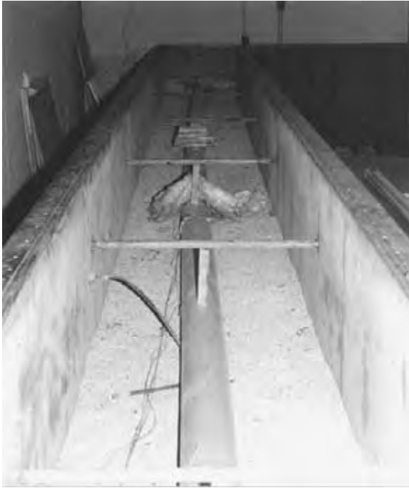
Figure 6.66 Condensate pipe in test cell.
