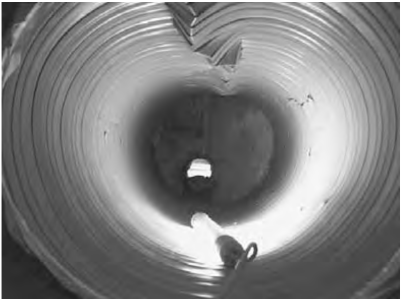
Figure 6.33 Steel-ribbed pipe (18-in diameter) at 75 ft of cover in silty-sand soil at 95 percent density.
