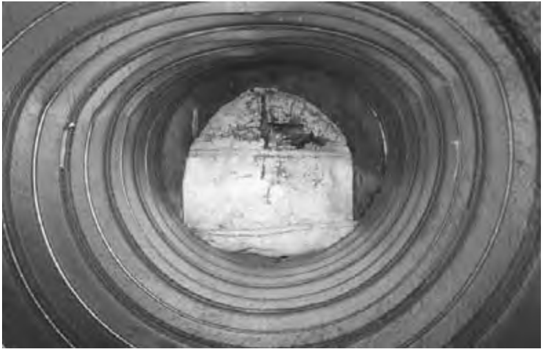
Figure 6.13 Inside the pipe at 35 ft of cover.
