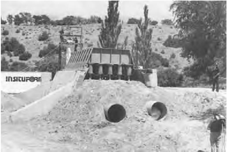
Figure 8.1 The testing of Insituform pipe in the USU large test cell.
