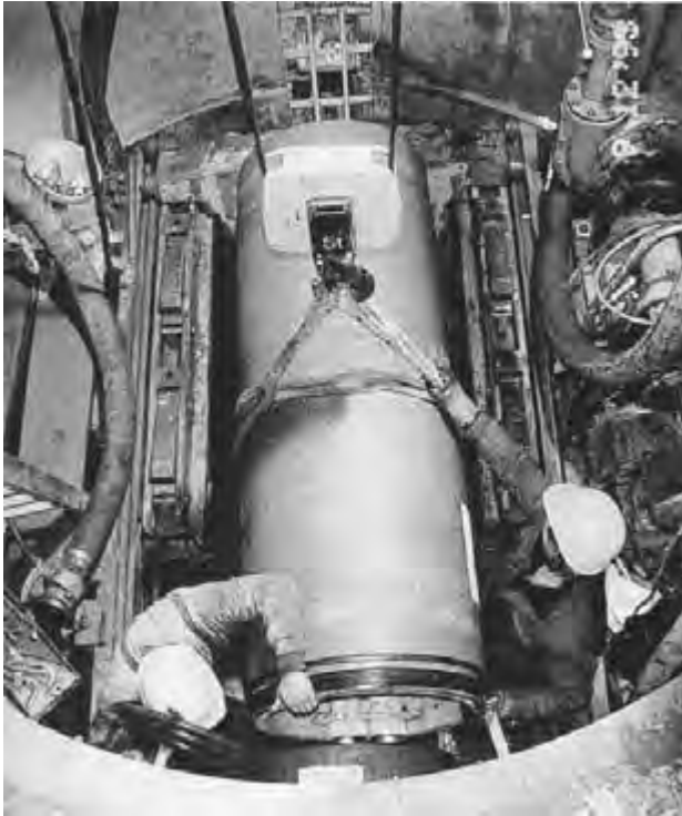
Figure 8.17 Polycrete pipe in jacking pit. (Courtesy of Meyer-Polycrete.)
