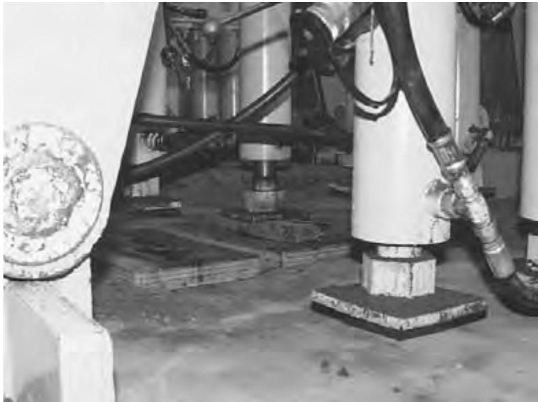
Figure 6.27 Application of 16,000 lb.
