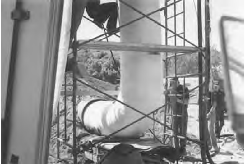
Figure 8.5 Process of inverting the Insitutube.
