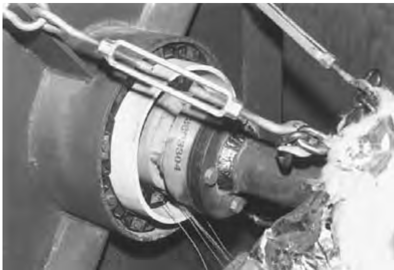
Figure 6.65 External connection and thrust restraint.
