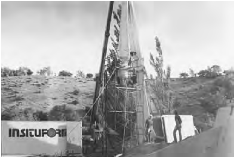
Figure 8.4 Equipment for inverting the Insitutube.
