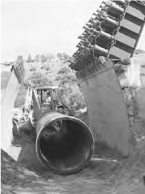
Figure 7.55 A 60-in HDPE pipe being placed in the test cell.
