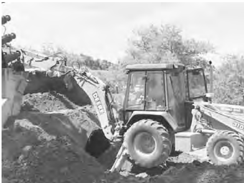
Figure 7.58 Backhoe loading soil in test cell.
