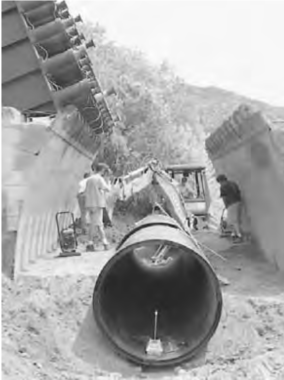
Figure 7.57 Soil placement, compaction, and density measurement.
