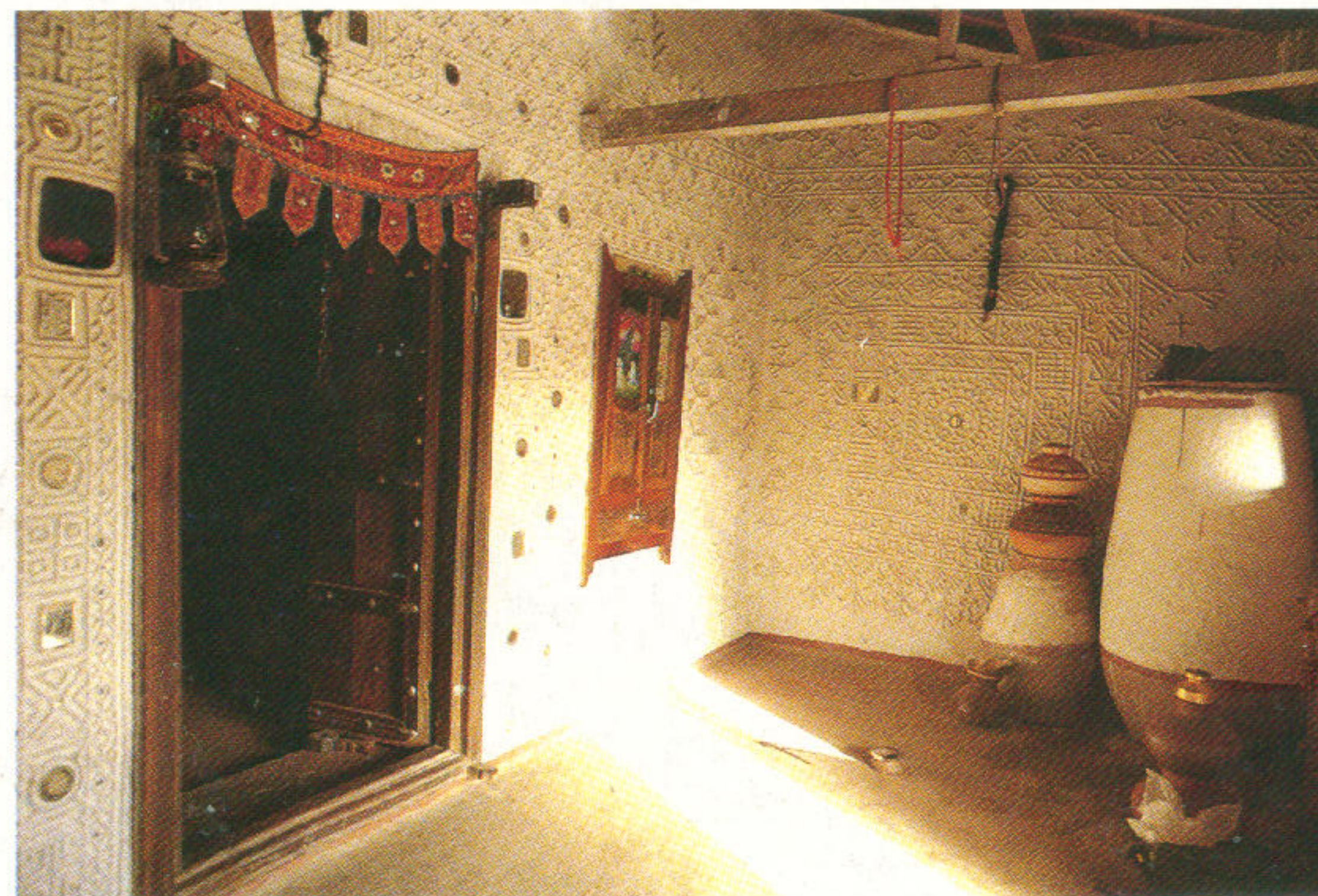
Pl. 20, 21, figs. 4-7. In Gujarat state, India, interior walls are delicately embossed with mud tracery. The artists are women of the Harijan and Rabari castes. Using no molds, they work the mud by hand into a wide variety of forms, from benches strong enough to support thirty heavy blankets to delicately faced shelves for brass utensils.
