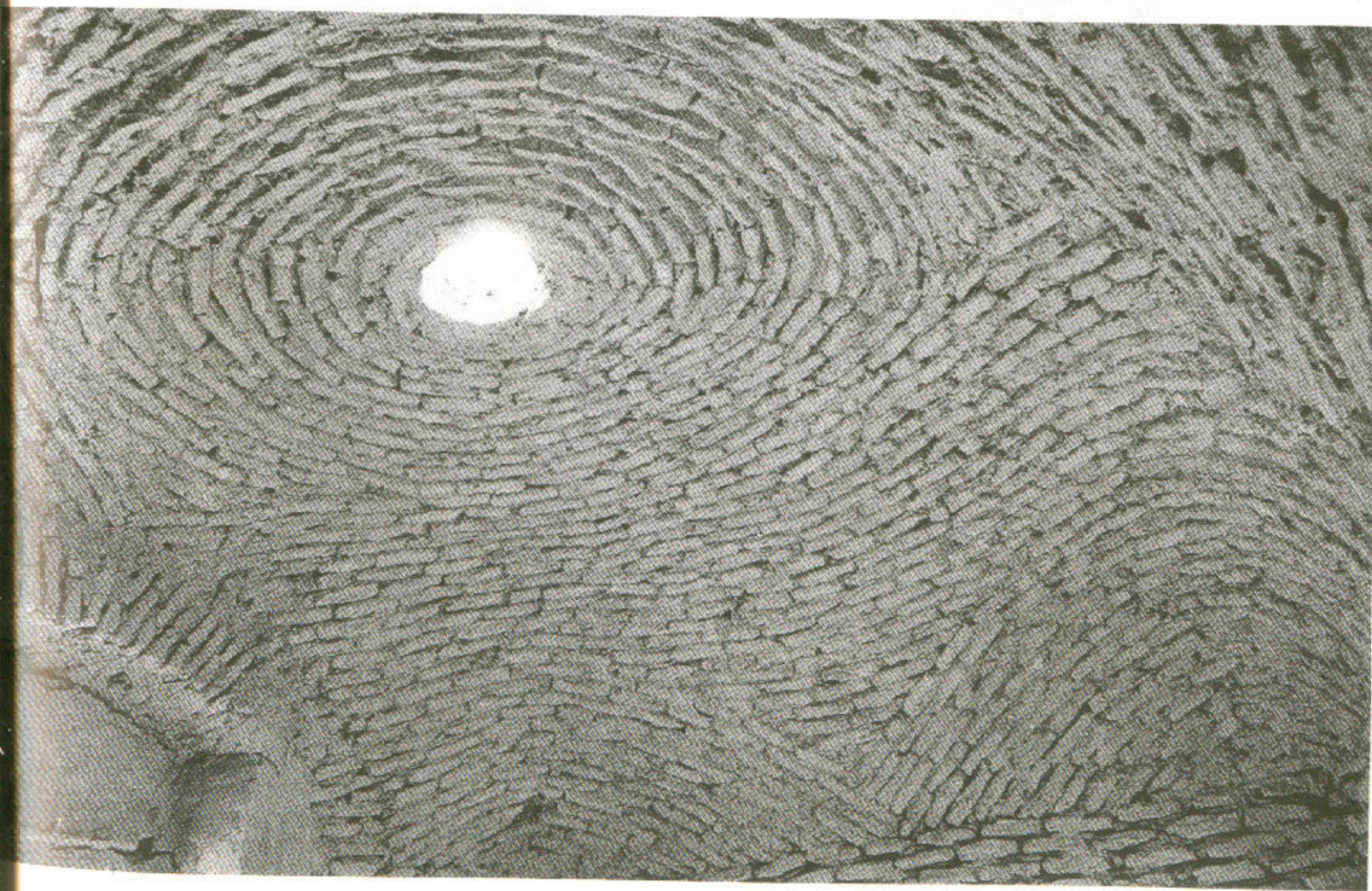
Figs. 45, 46. Ribless vaults and domes are found throughout the Middle East.
