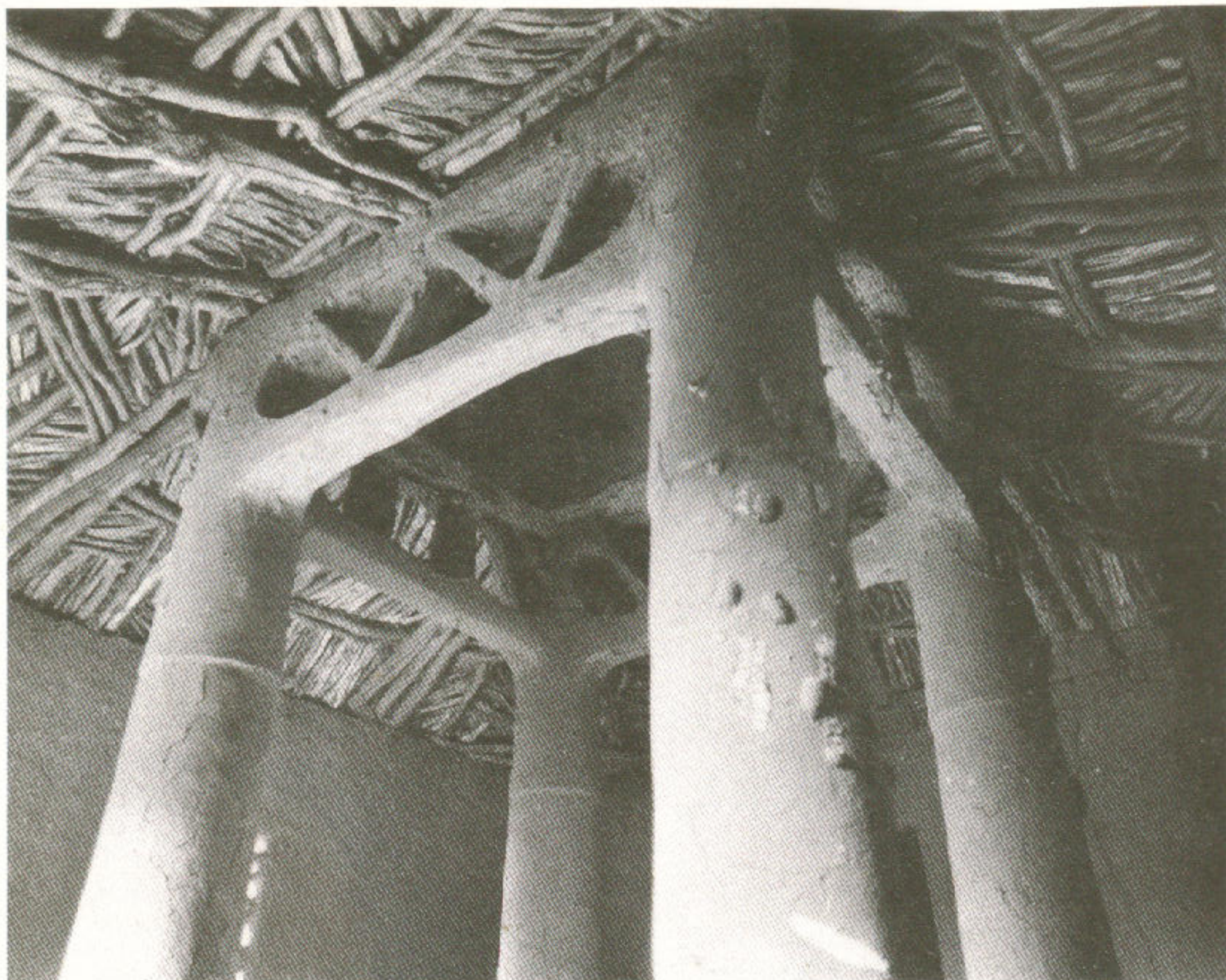
Figs. 42-44. In areas where there are few trees to provide long beams, interior space is spanned by many methods. In a small mosque in Niger, a set of columns supports the central lantern roof. An entry house's single central pillar is made of solid mud. And another entry house has a "Hausa dome" with saplings for ribs, a system adapted from the tents used years ago, when the Hausas were nomads.
