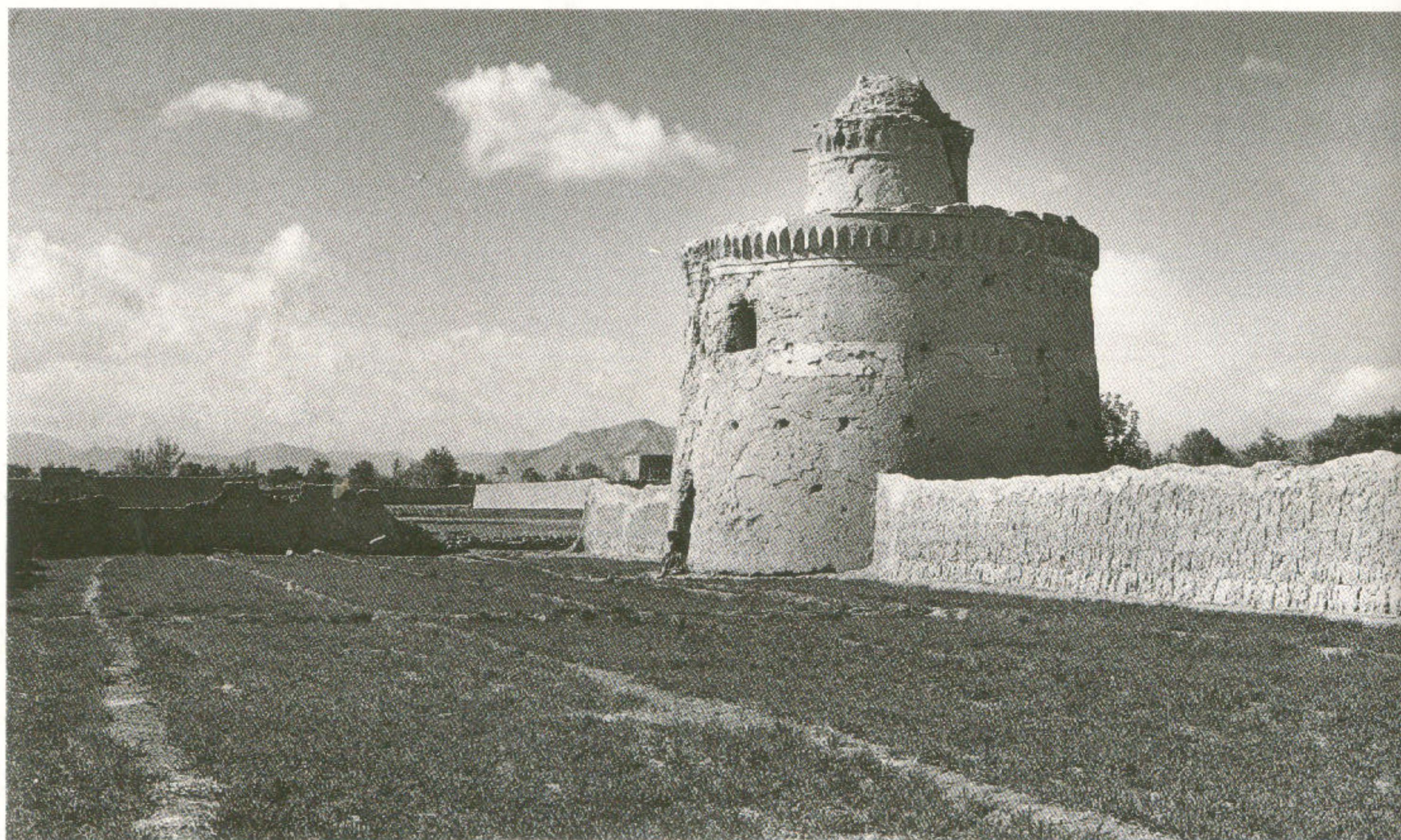
Figs. 8, 9. Iranian pigeon towers were built to collect pigeon droppings for fertilizer. Each pigeon-hole is furnished with its own perch.
