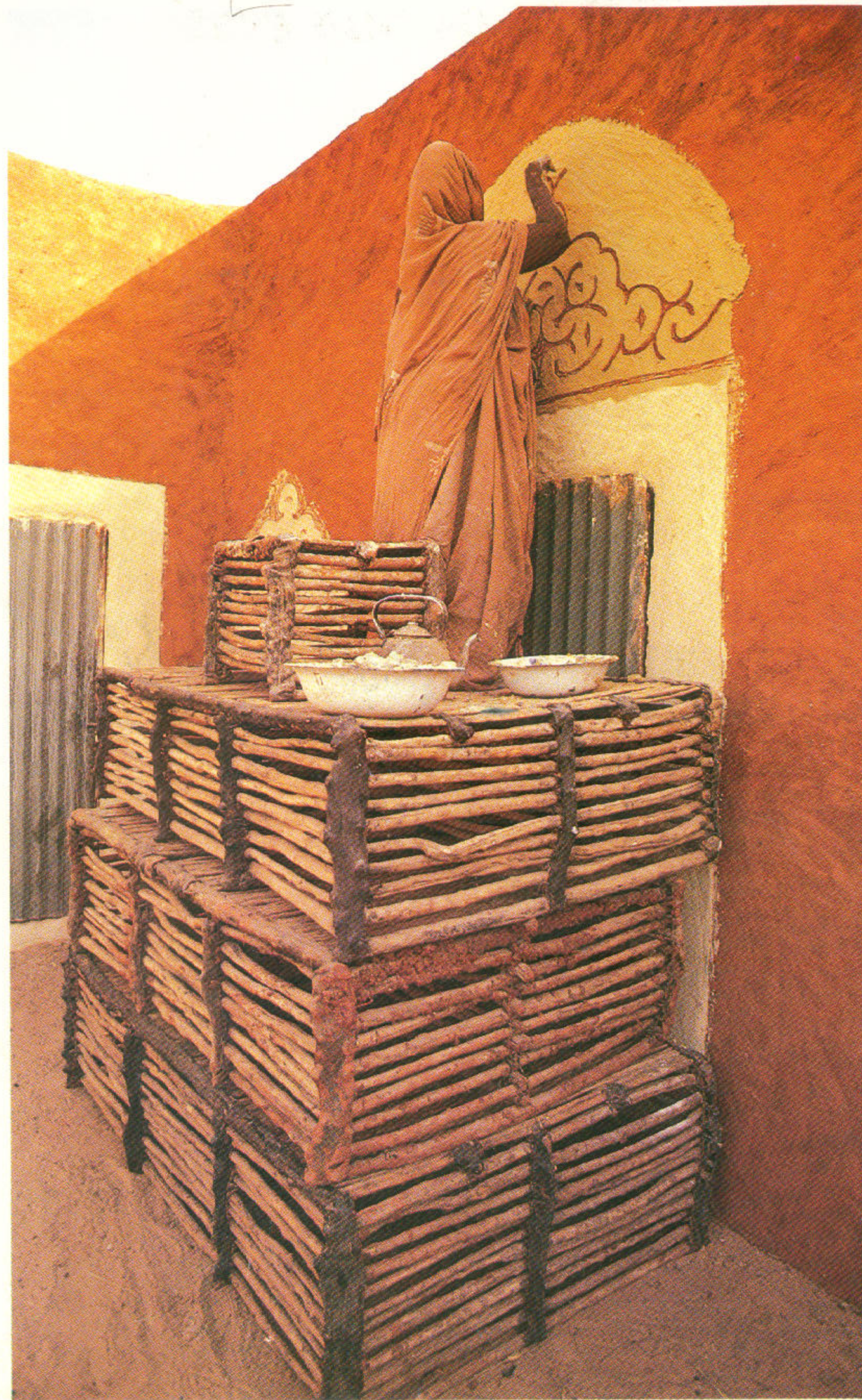
Pl. 10. After a wall is plastered, decoration may be applied. Standing on a stack of beds, a woman incises a pattern.
