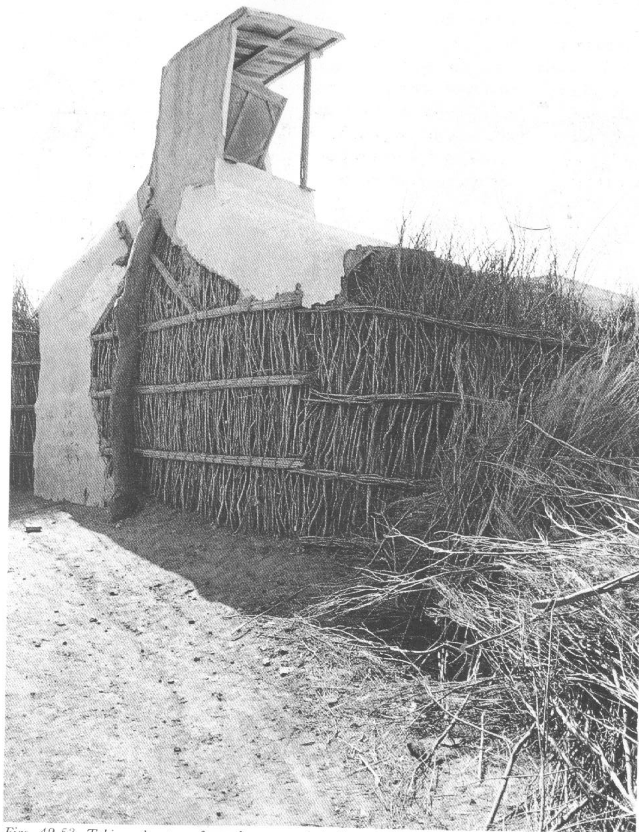
Figs. 49-53. Taking advantage of a cool summer wind, Sindis in southern Pakistan build wind-catchers to channel the breeze down into their houses.
