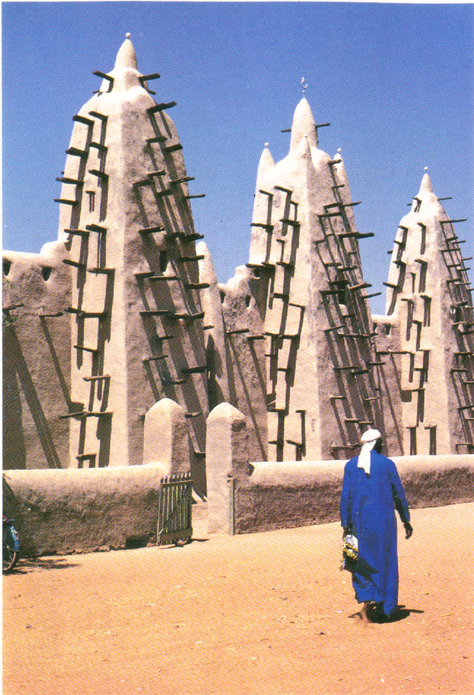
Pl. 23. Sticks bristle from walls and towers, providing permanent scaffolding for maintenance. Pinnacles are often topped by ostrich eggs, symbols of fertility.
