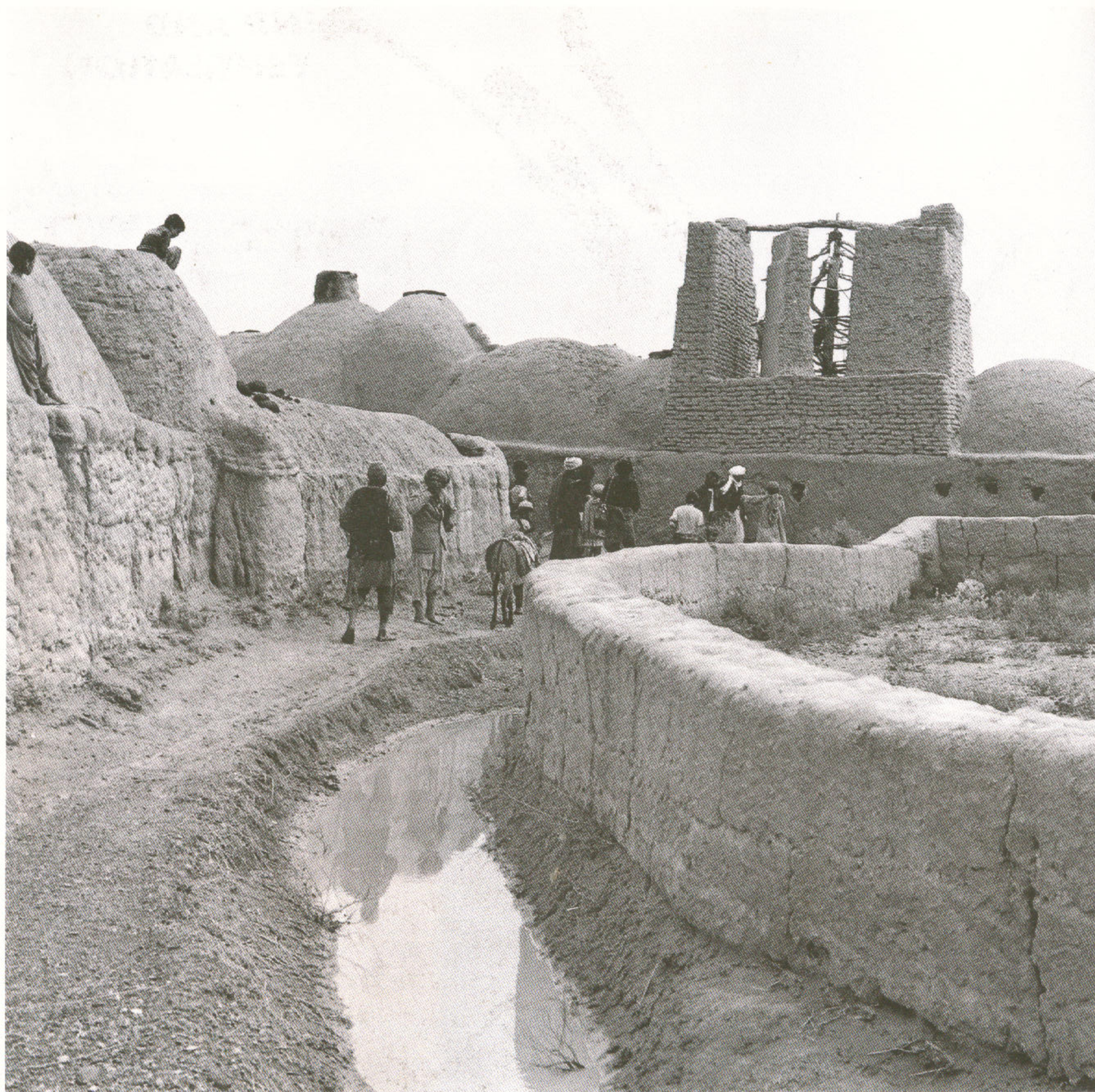
Figs. 47, 48. Built to grind grain, an Afghan windmill with horizontally rotating sails recalls the world's earliest, invented in the region more than one thousand years ago.
