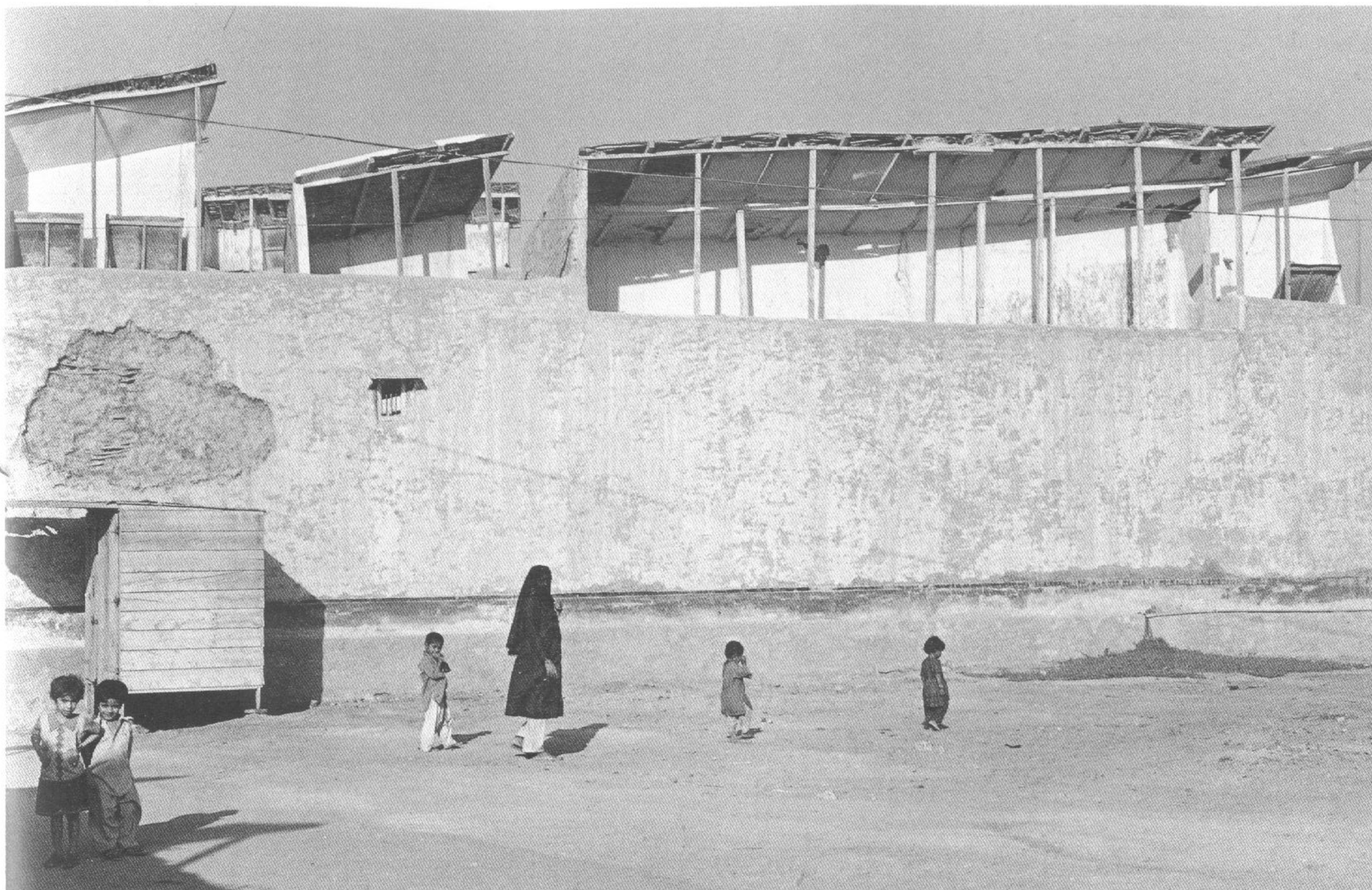
Figs. 52, 53, drawings A, B. A twenty-year-old house in the town of Tatta boasts a wind-catcher twenty-eight feet long. Below it, a wind-room has four windows and two doors which can be opened in any combination to regulate air flow.
