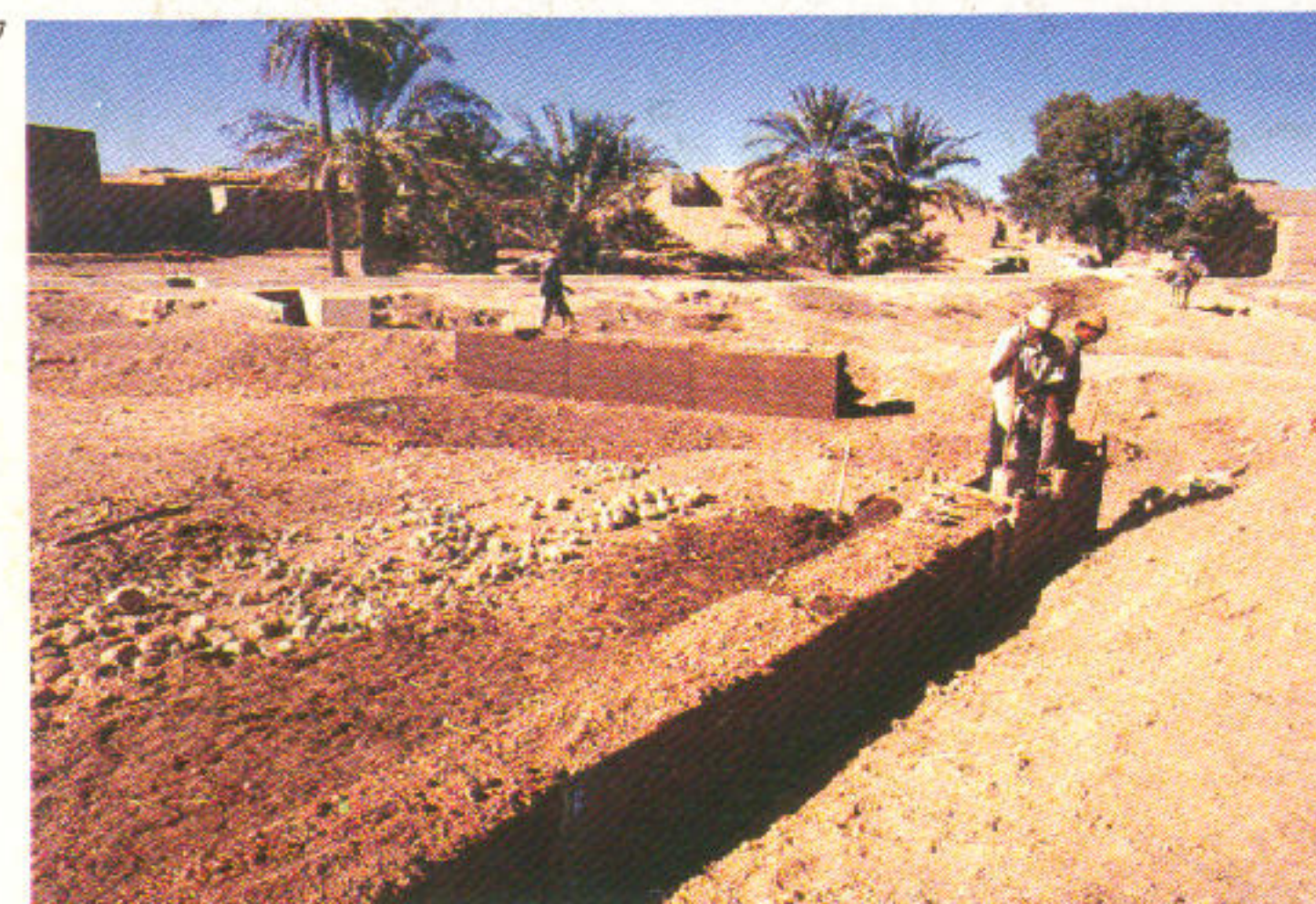
Pl. 6. Mud bricks drying in the sun.
