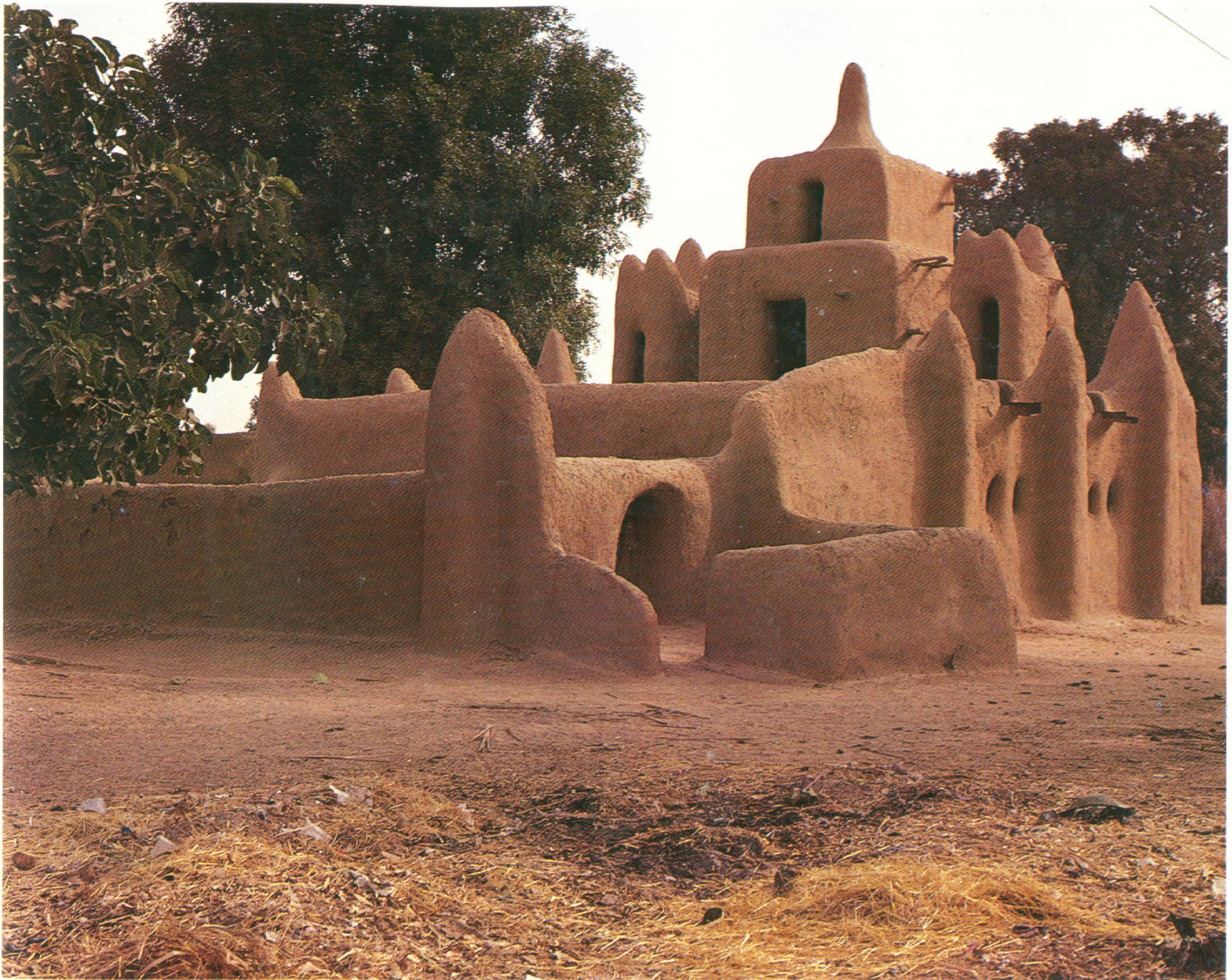
Pl. 22-39. The dry savannah south of the Sahara features a unique style of mosque. The sculpted look of the older and more rural mosques is not due to weathering; molded contours are part of the original design.
