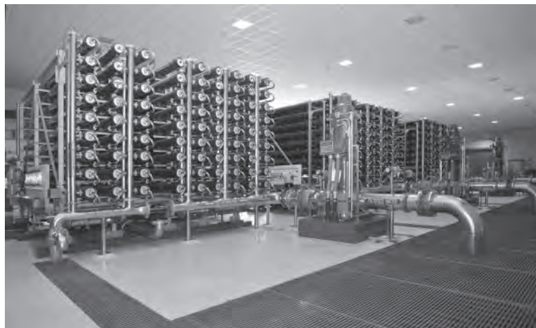
Figure 9-2 Typical reverse osmosis facility.
