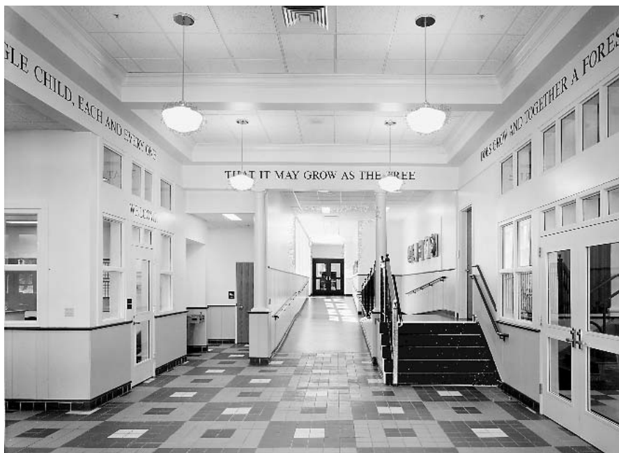
◀ Barrier-free design often involves incorporating ramps into a school's circulation. Carrie Ricker Middle School, Litchfield, Maine. Harriman Associates.
