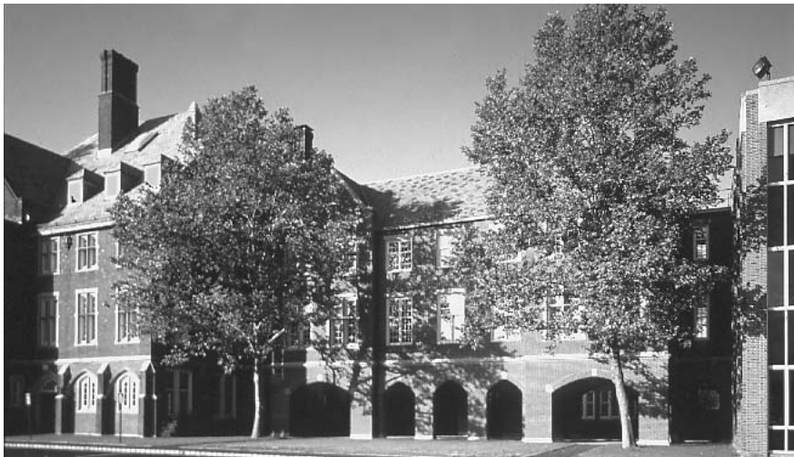
◀ The Scarsdale, New York, school system initially used unattractive brown replacement windows in the older Georgian and Collegiate Gothic style schools and, because of community reaction, replaced them several years later with more architecturally appropriate units with superior energy conservation and operating characteristics. Peter Gisolfi Associates. (Photograph by Norman McGrath.)
