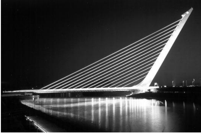
FIGURE 3.9 Alamillo Bridge, Seville, Spain.
