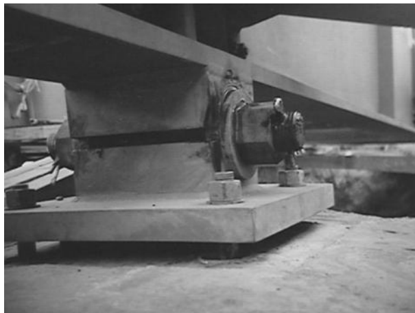
FIGURE 1.6 Steel pin bearing application.
