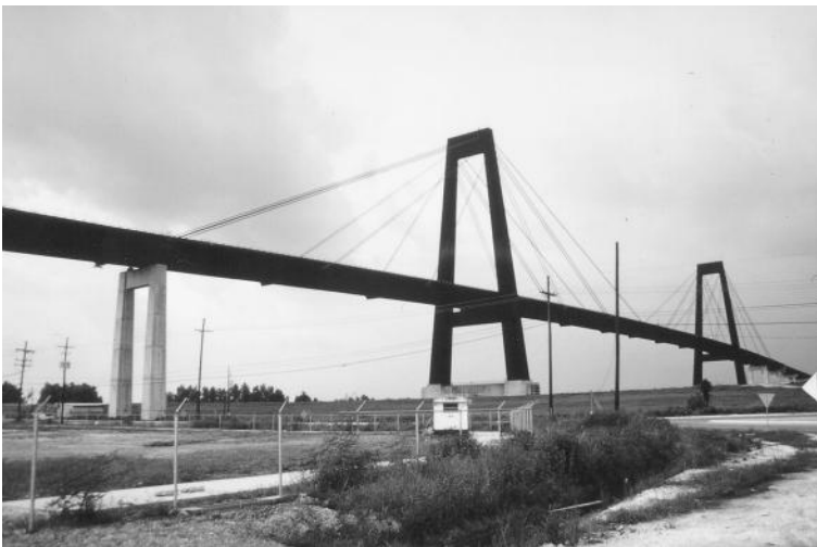
FIGURE 3.16 Luling Bridge, New Orleans, Louisiana. (Courtesy of Charles Seim.)
