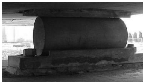
FIGURE 1.7 Steel rocker bearing application.
