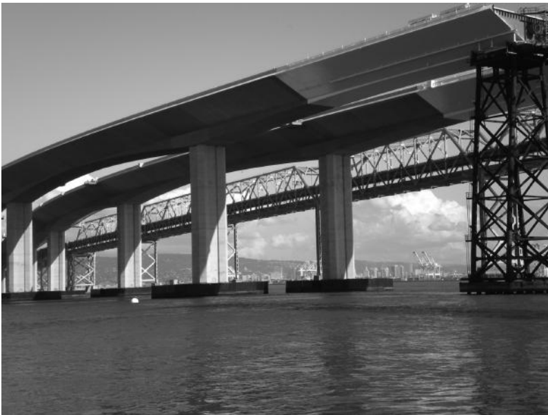
FIGURE 2.2 Columns in Skyway structure of San Francisco–Oakland Bay Bridge.
