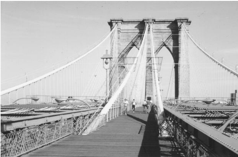
FIGURE 3.4 Brooklyn Bridge, New York. (Courtesy of Charles Seim.)
