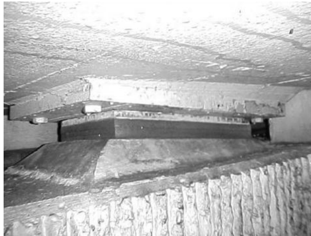
FIGURE 1.4 Fabric pad sliding bearing application.
