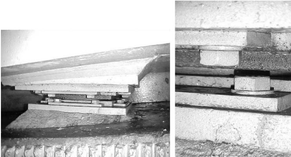
FIGURE 1.13 Disc bearing application.
