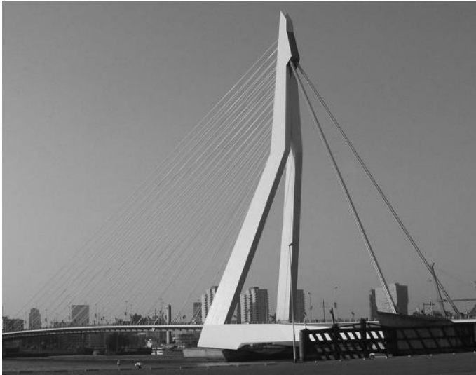
FIGURE 3.10 Erasmus Bridge in Rotterdam, the Netherlands. (Courtesy of Charles Seim.)
