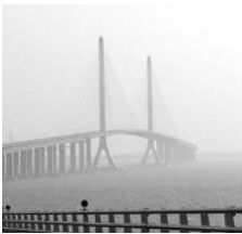
FIGURE 3.19 Distinctive towers for cable-stayed and suspension bridges.
