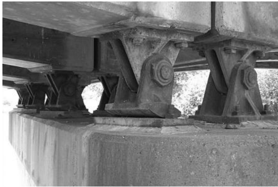
FIGURE 1.7 Steel rocker bearing application.
