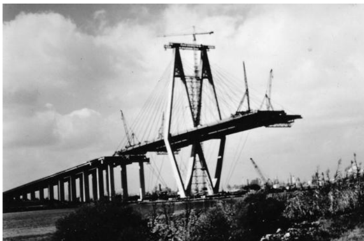
FIGURE 3.21 Baytown Bridge, Texas. (Courtesy of T. Y. Lin International.)
