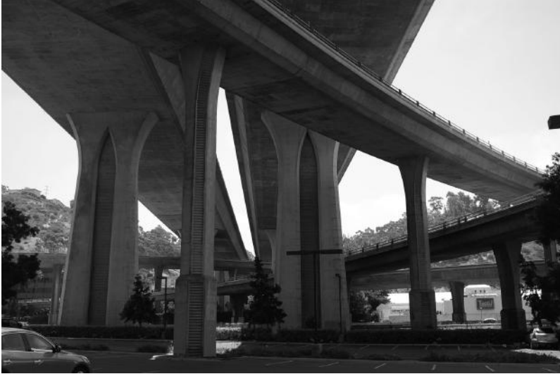
FIGURE 2.1 Columns in a typical urban interchange.
