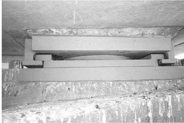
FIGURE 1.11 Pot bearing application.
