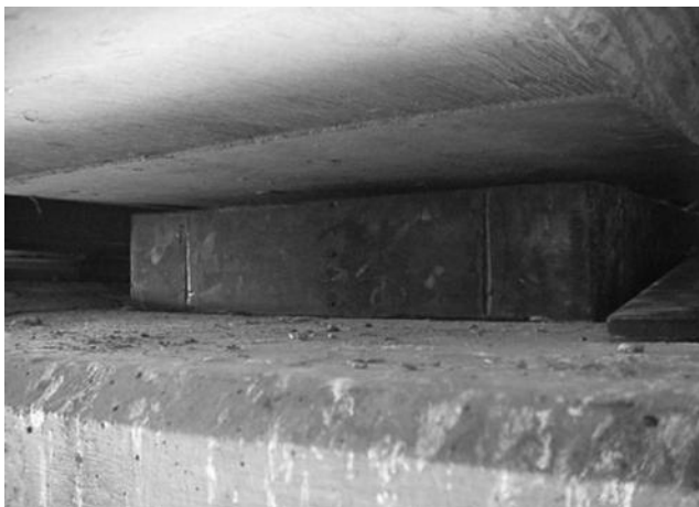
FIGURE 1.1 Steel reinforced elastomeric bearing (concrete bridge) application.
