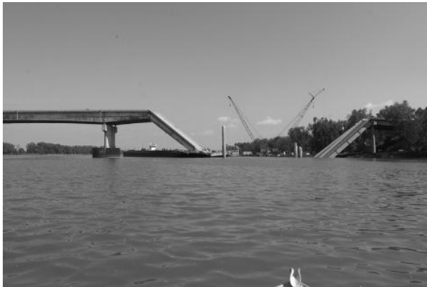
FIGURE 4.2 I-40 Bridge over Arkansas River, OK (2002).
