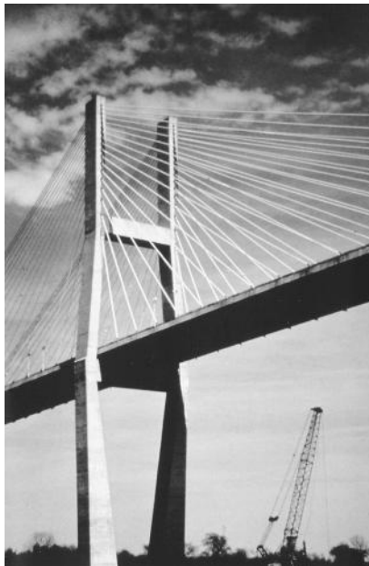
FIGURE 3.20 Talmadge Bridge, Georgia. (Courtesy of T. Y. Lin International.)
