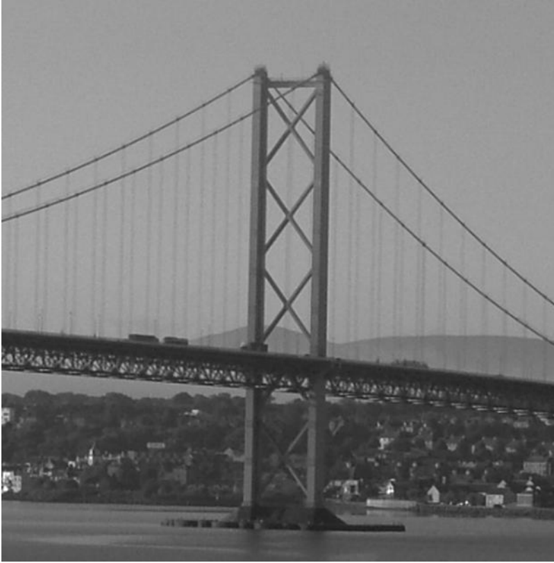
FIGURE 3.3 Firth of Forth Suspension Bridge. (Courtesy of Charles Seim.)
