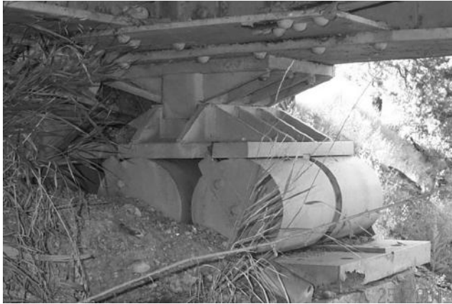
FIGURE 1.9 Nested roller bearing application.
