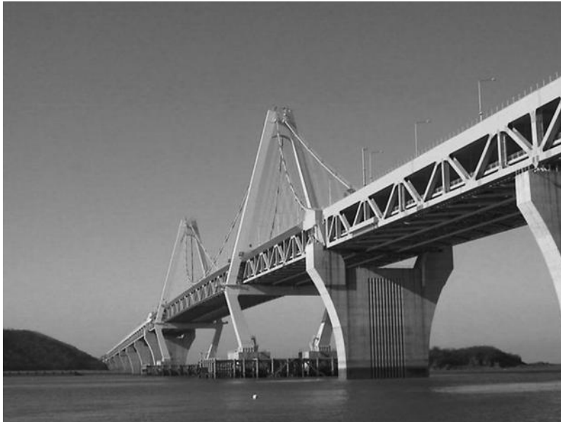
FIGURE 3.6 Yeongjong Grand Bridge, Incheon, South Korea.
