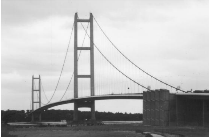
FIGURE 3.22 Humber Bridge, England. (Courtesy of Charles Seim.)
