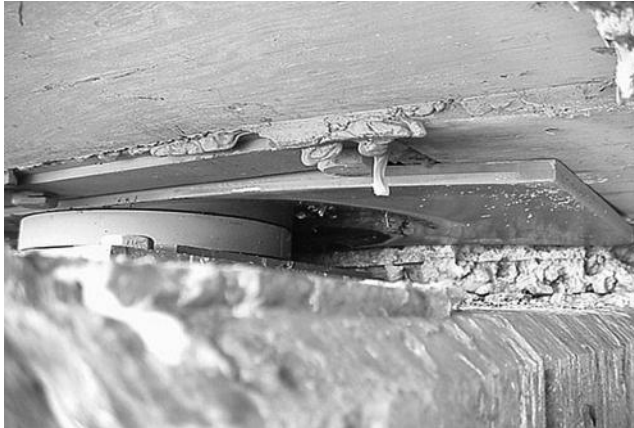
FIGURE 1.15 Spherical bearing application.
