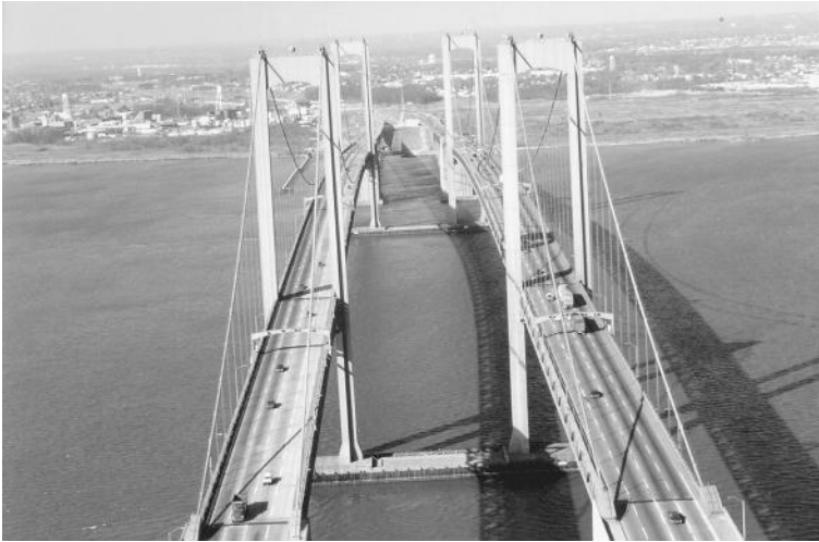
FIGURE 3.15 Delaware Memorial Bridges. (Courtesy of D. Sailors.)
