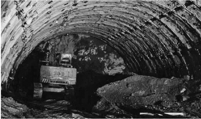
Figure 4-9 Outer support layer with deformation slots.
