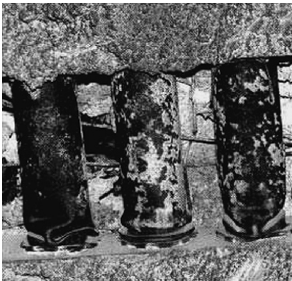
Figure 4-10 Dilatation tube element in the Galgenberg Tunnel [324].
