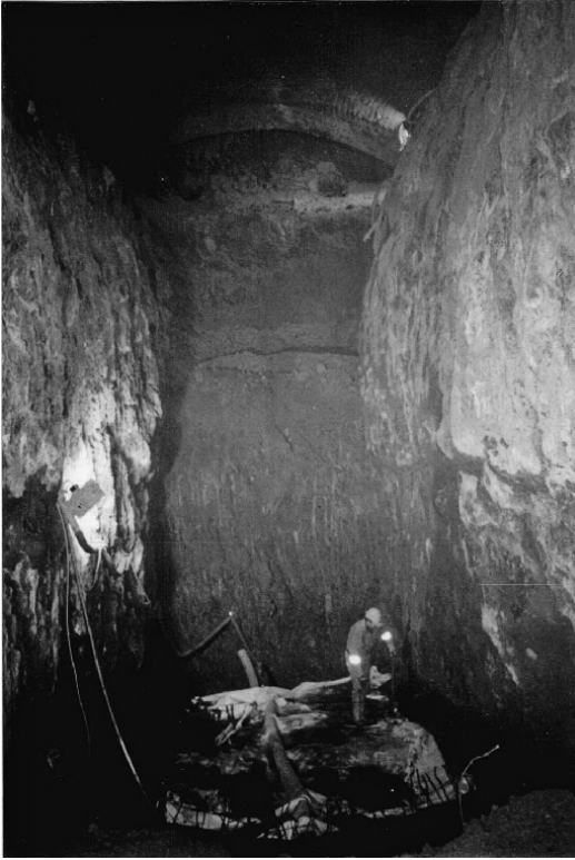
Figure 4-12 Core excavation in the Himmelberg Tunnel.
