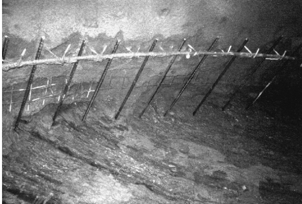
Figure 2-23 Use of spiles in the Euerwang Tunnel
