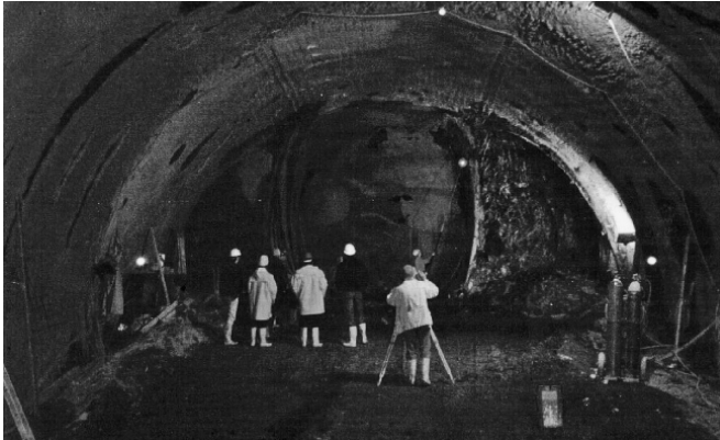
Figure 4-7 Crown pilot heading method in the Schulwald Tunnel.
