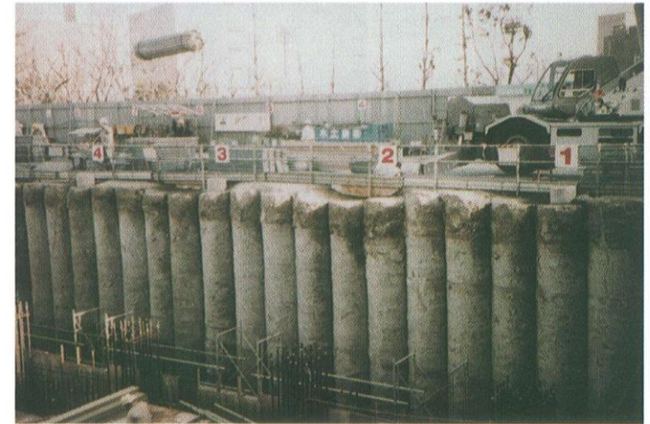
Excavated surface of Retaining Wall by Deep Mixing columns
