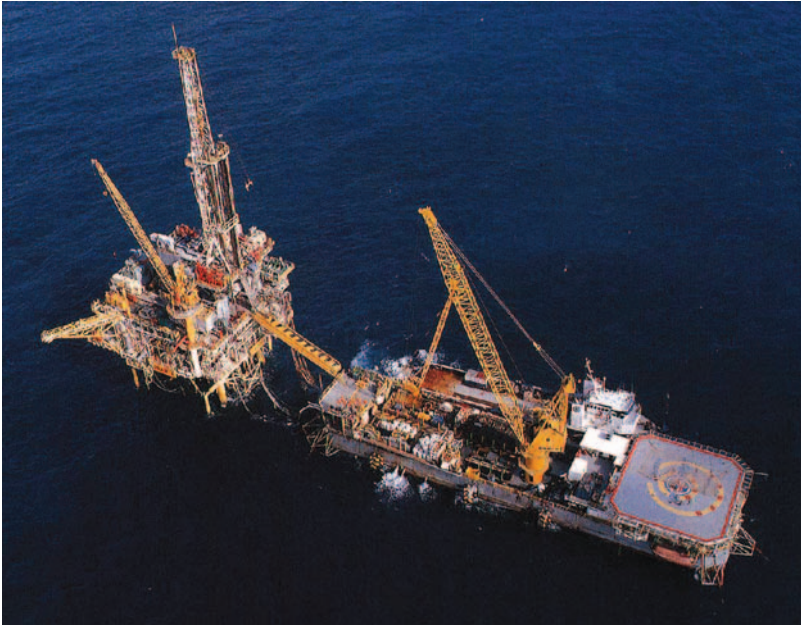
Figure 4.5 Tender-assisted drilling.
