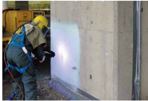
Fig. 11A Activated Arc Sprayed Zinc Anode Installation
