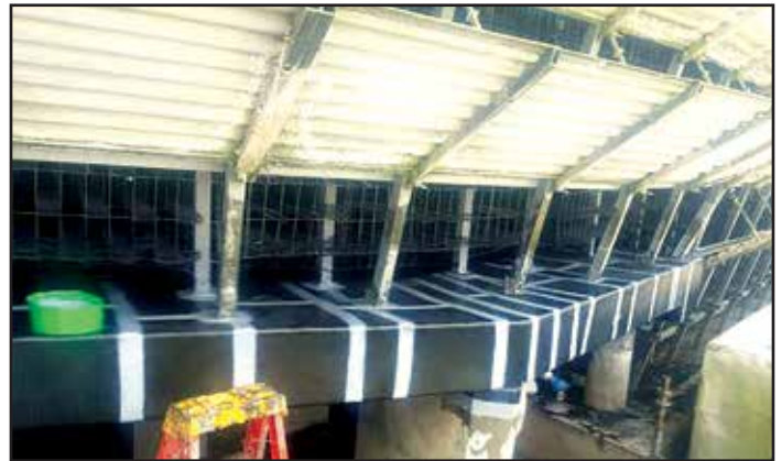
Fig. 45 Previously repaired beams strengthened with CFRP.
