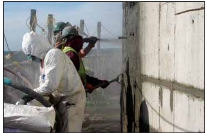
Fig. 18 Shotcrete installation.
