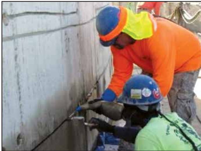
Fig. 20 Grouting ribbon anode in continuous saw-cut slot at shell exterior.
