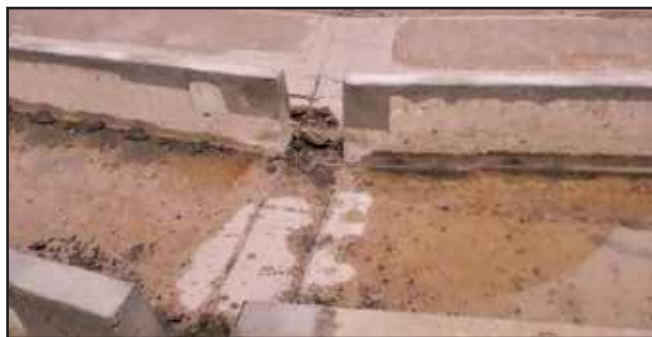
Fig. 41 Concrete fins repaired, prior to protective coating application.
