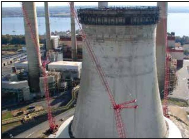
Fig. 15 Rebuild of the upper third of the tower, in progress.
