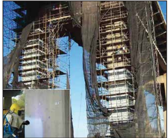
Fig. 12 Activated Arc Sprayed Zinc Project Installation
