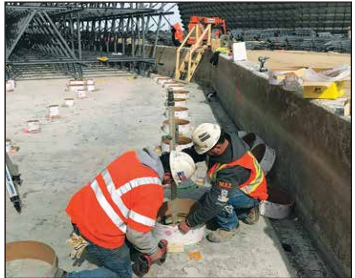
Fig. 49 Concrete pedestals installed to support new FRP cooling tower framing.
