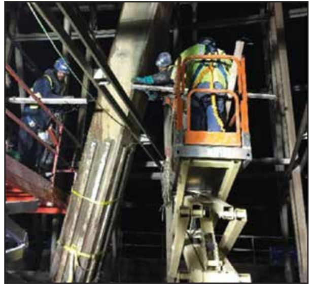
Fig. 7 Connecting Anode to Reinforcing Steel
