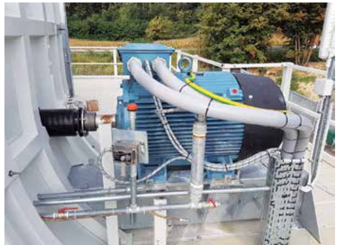
Fig. 2.3: ABB Electric Motor (EM) and Carbon Shaft (CS)
