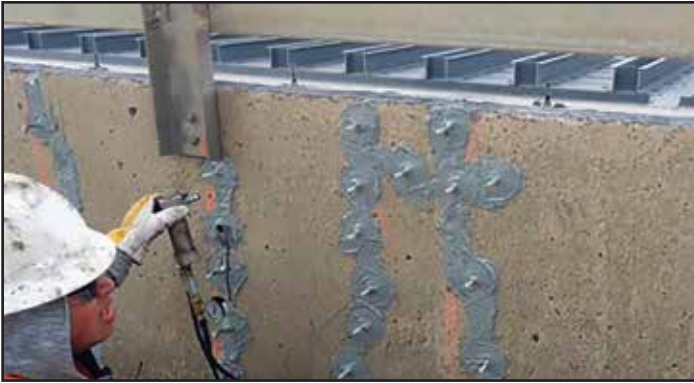
Fig. 42 Epoxy adhesive injected to seal fine cracks in the basin walls
