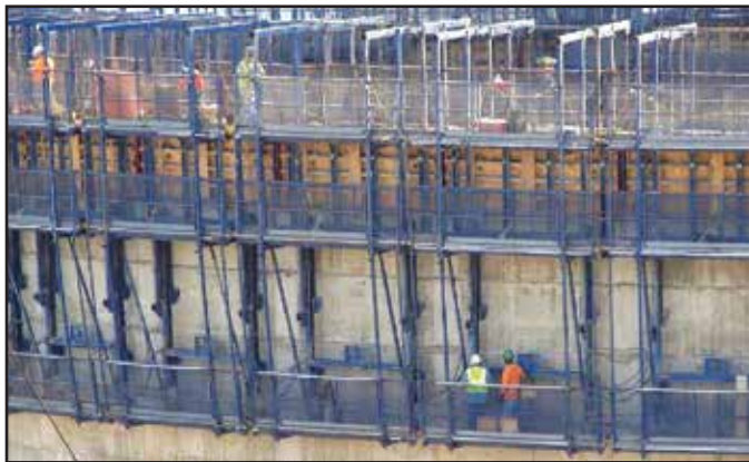
Fig. 16 Three-level self-climbing work platform
