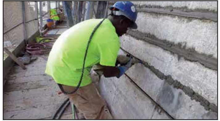
Fig. 27 Grouting slots after ribbon anode installed
