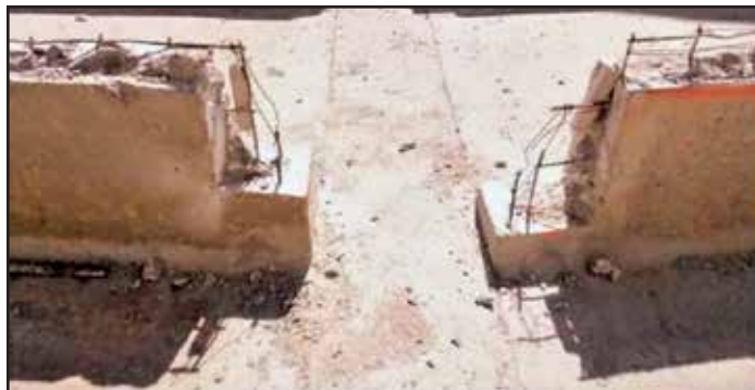
Fig. 40 Prepared precast fins with galvanic anodes awaiting new high performance concrete.
