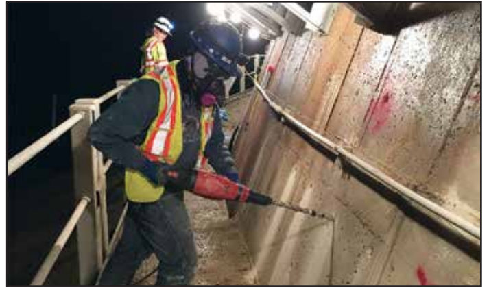
Fig. 28 Drilling for Ebonex Discrete Anodes
