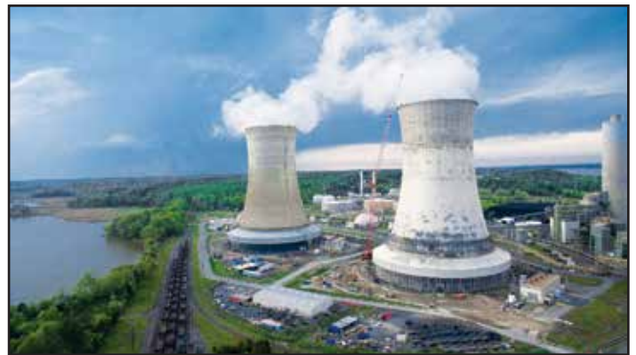
Fig. 1 Mid-Atlantic Generating Station Cooling Tower
