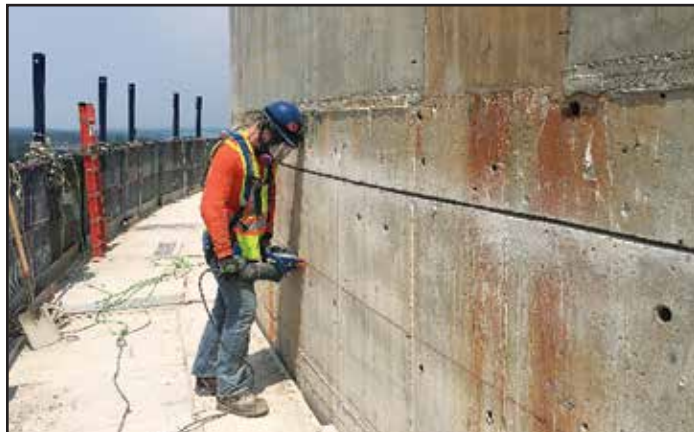
Fig. 26 Sawcutting slots for ribbon anode
