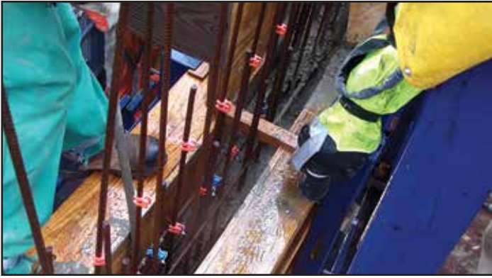
Fig. 24 Ribbon anode installed in new concrete
