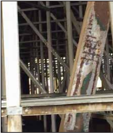
Fig. 4 Remove Delaminated Concrete
