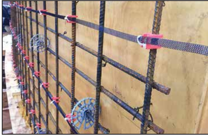
Fig.25 Ribbon anode ready for new concrete
