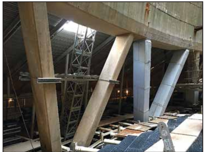
Fig. 8 Completed Jacket
