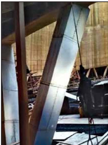
Fig. 6 Install and Grout Jacket Sequence of X-column galvanic jacket installation.
