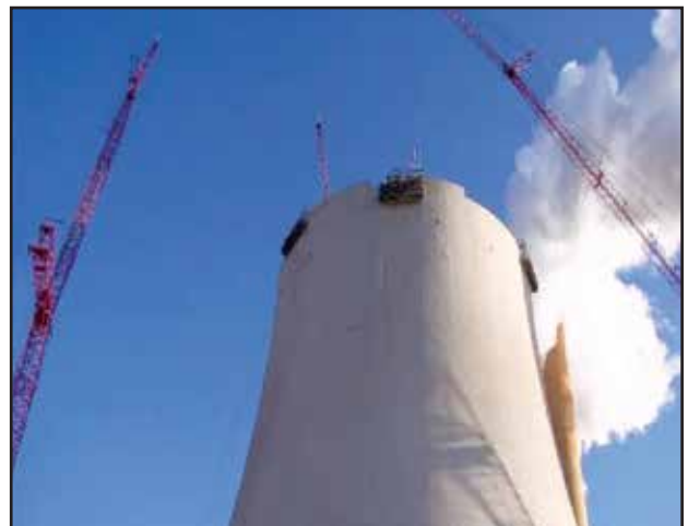
Fig. 13 Demolition of upper third of the tower in progress.
