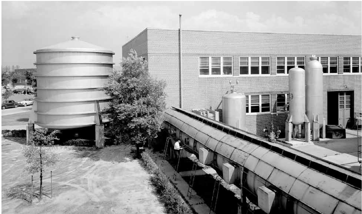
View of the Physical Research Laboratory at Langley in 1949 showing the ill-fated Langley Free-Flight Facility in the foreground. The 100-foot-long, 8-foot-diameter facility was equipped with viewing windows but suffered poor flow characteristics during model flights and was closed before meaningful research results were obtained.
