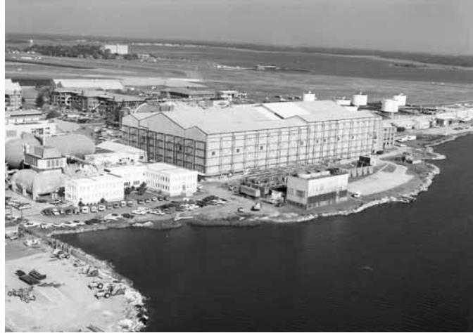
The huge Langley Full-Scale Tunnel has been the focal point of NASA's free-flight model studies. The large test section and open-throat design permit flight-testing of relatively large sophisticated models of aerospace vehicles.
