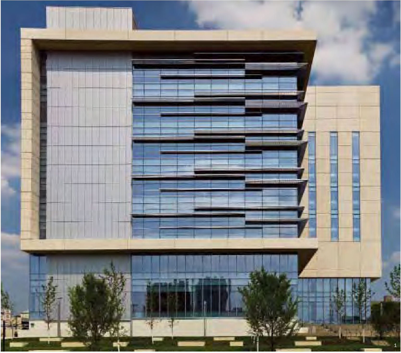
1. Side view of the building 2. Sun shading devices to minimize solar gain and maximize views
