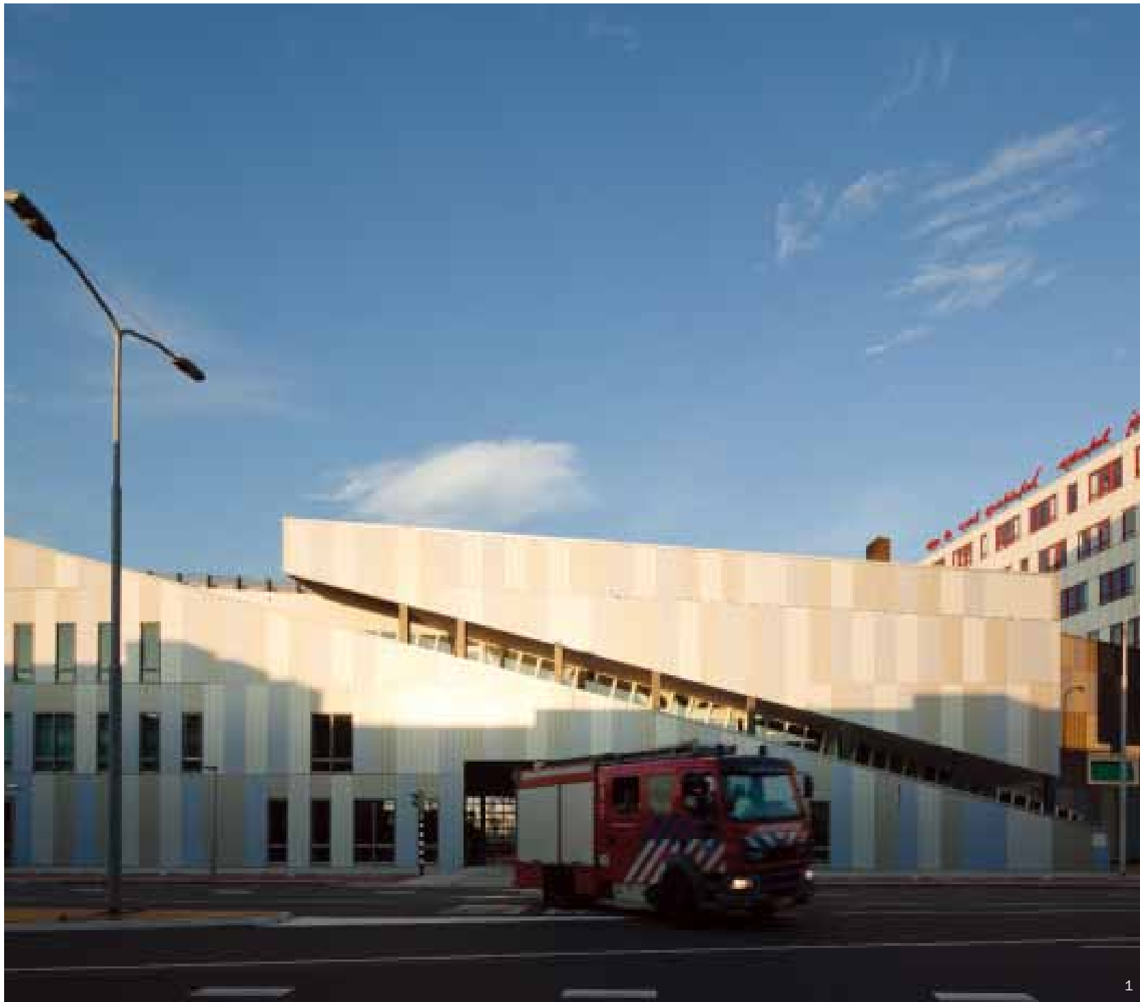
1. The visible strong slanting line on the front and back of the building forms the access ramp for the parking on the roof 2. Details of the fire engine garage
