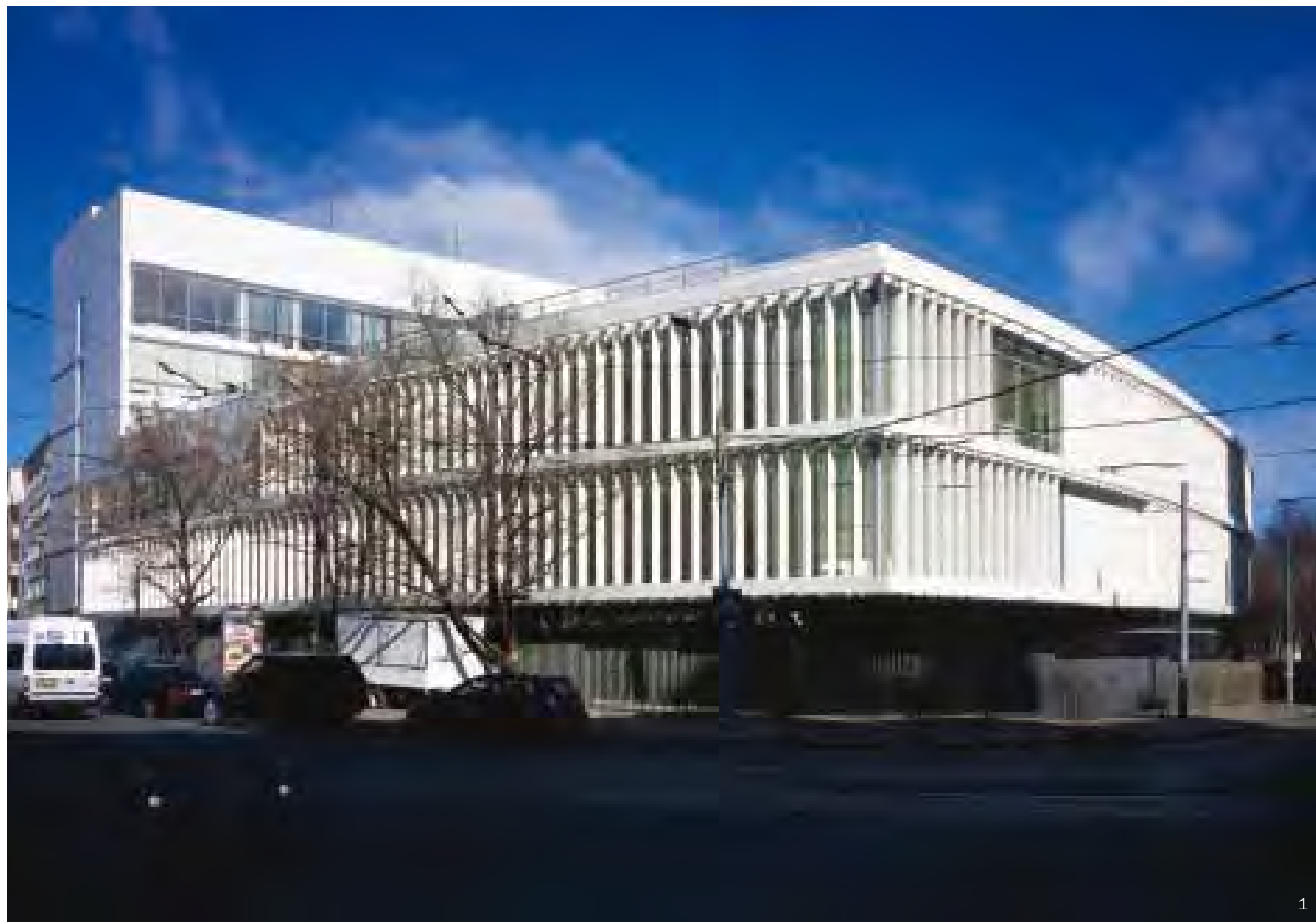
1. The sweeping shutters installed on the public building could effectively filter the strong sunlight, and also give a sense of grace 2. A seven-storey accessory building locates at the back of the building
