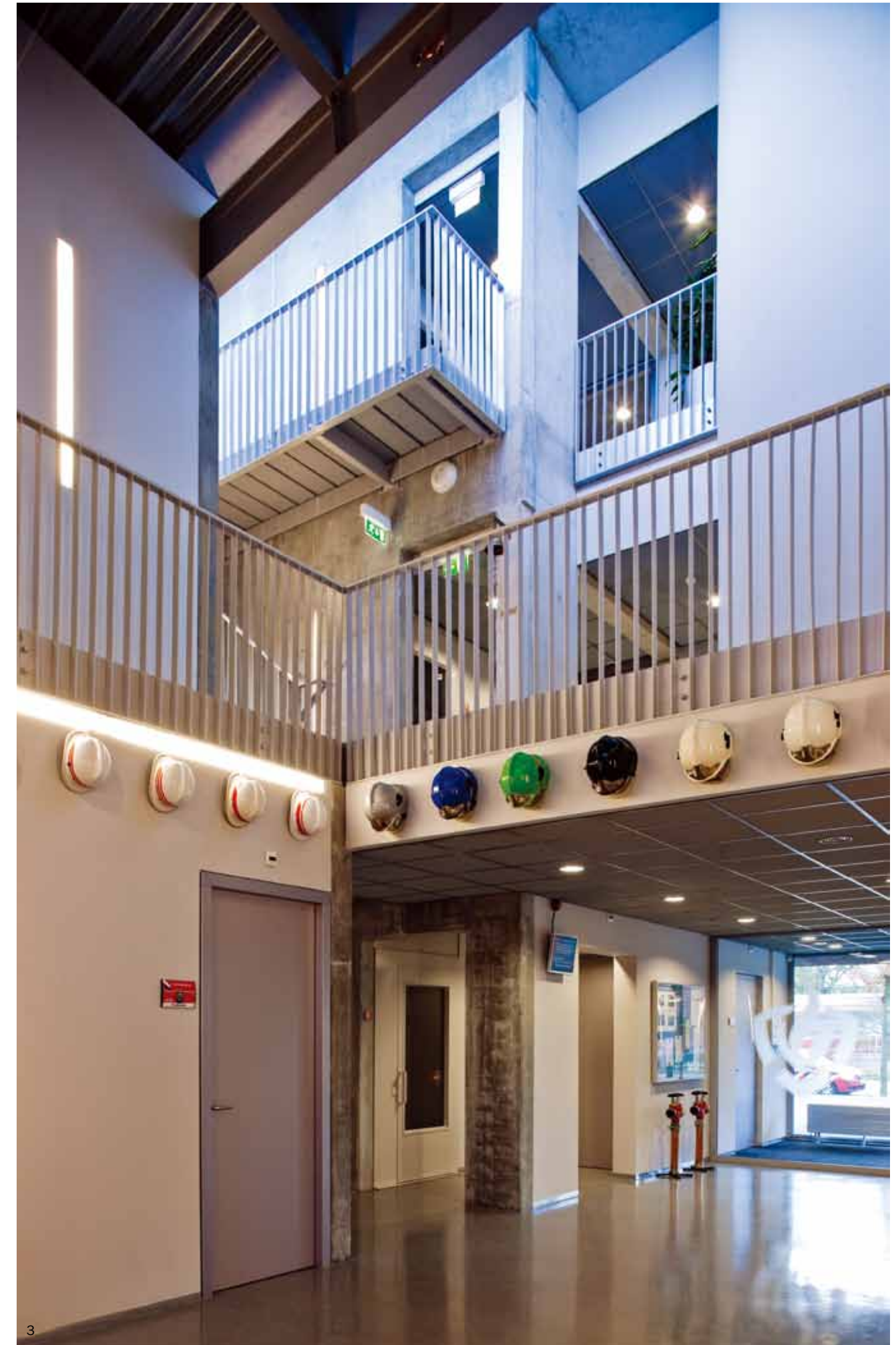
1. Overlooking the entrance hall from the corridor at the first floor 2. Details of the inner structure
