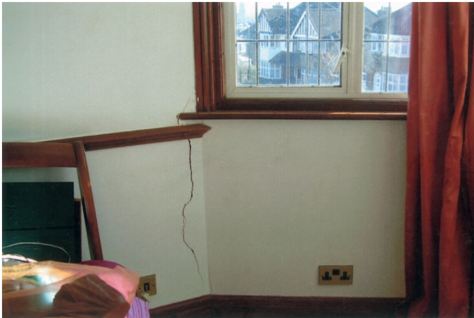
FIG 4.1 A number of problems may be found when sealed unit double glazing is installed in existing buildings. Condensation between the glass in sealed units is very common necessitating replacement of the glass. When double glazing is installed in bay windows, it is important to check whether the construction above is fully cantilevered or whether the ground floor window frames support the window, wall and gable above. In this case the bedroom bay is cracking and pulling out because the support provided by the original, more substantial, window frame below has been removed.
