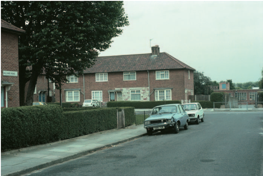
FIG 2.3 Artificial stone cladding generally reduces the value of the property to which it is applied, and in this case by cladding only at ground floor level the owner has left a ledge for driving rain to penetrate behind the cladding resulting in a damp problem inside.
