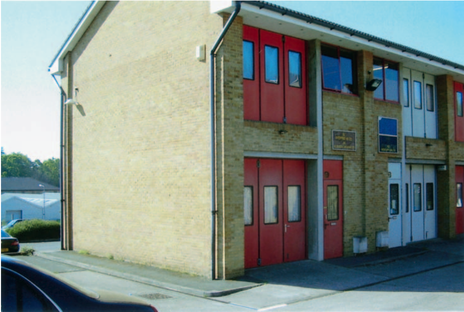
FIG 12.2 A simple low-rise industrial building. A Building Survey here follows the same principles as for a residential property. Buildings of this type are often built on brownfield sites or disturbed ground, so look out for signs of movement. Also will the floors take the weight? access and loading heights? services including three-phase electricity? adequate heating, lavatory and washing facilities?
