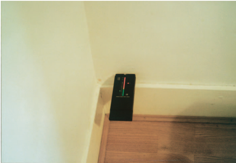
FIG 18.2 Testing No. 1 Suburban Road for damp. The green light on the left indicates that the wall is dry. If the light moves up into the red sector it would indicate increasing levels of moisture in the wall plaster. This would not necessarily indicate rising damp due to failure of damp-proof courses however; there are many other reasons why wall plaster could be damp.
