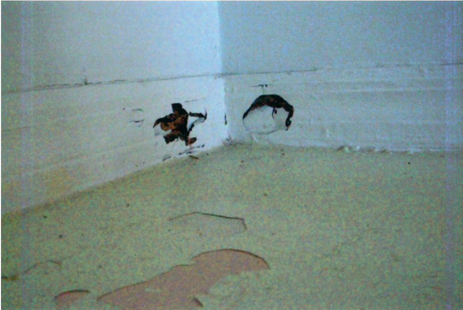
FIG 5.1 A solid concrete floor and masonry walls. The damp-proof membrane in the floor is not contiguous with the damp-proof course in the walls, allowing dampness to rise up behind the skirting boards resulting in rot. Look out for rusting nail heads showing through skirting board paintwork – a sure sign of dampness behind. Fortunately, in this case there is no adjacent timberwork, so the remedy is to deal with the damp and replace the skirtings. If this were a timber floor then more extensive investigation would be needed to establish how far the rot had travelled beneath and whether the true dry rot fungus – Serpula lacrymans – may be active.
