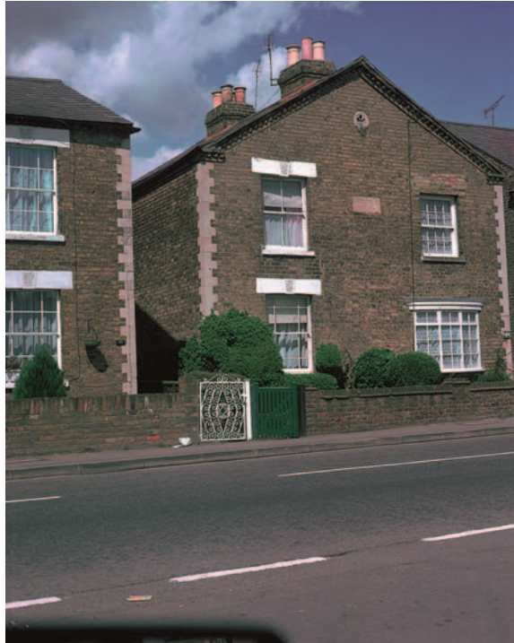
FIG 21.4 The arch over first floor window has spread and the lintel has dropped. This section of wall will need to be rebuilt.
