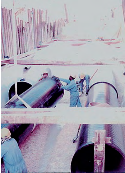
(a) Twin 1000 mm diameter ductile iron pipe laying in Middle East. (Black & Veatch)
