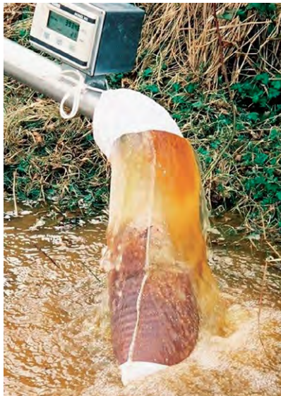
(b) Flushing a 100 mm diameter cast iron main. Debris collects in net for grading and analysis. Flow meter records the quantity of water used. (Black & Veatch)
