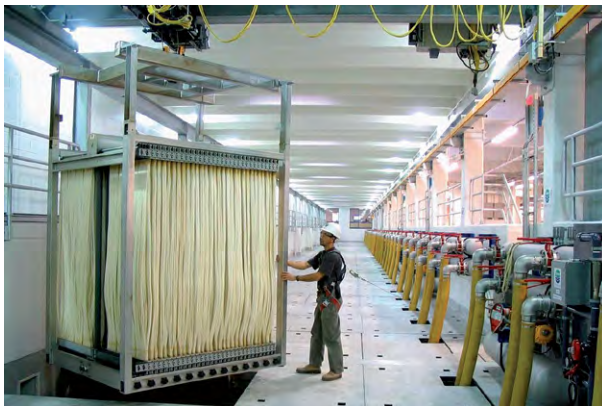
(b) Zenon ZeeWeed® 500d immersed membrane cassette being lowered into a tank. (Photo: GE Water and Process Technologies, Canada)
