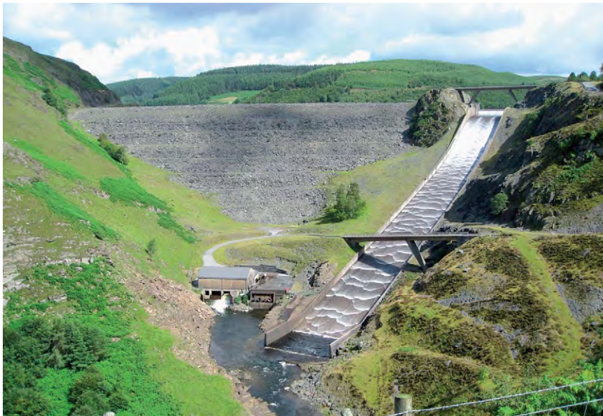
(b) Llyn Brianne 91 m high rockfill dam, Wales; side spillway: capacity 850 m 3 /s. (Courtesy of Aled Hughes) (Engineer: Binnie & Partners)
