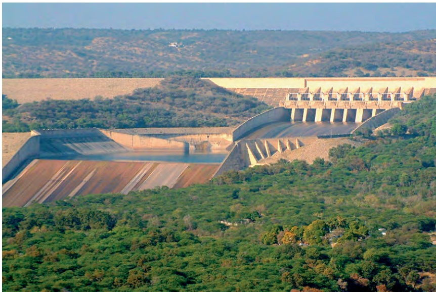
(b) Main spillway of 138 m high earth dam at Mangla, Pakistan—capacity 25 000 m 3 /s. (Engineer: Binnie & Partners) (Courtesy of O J Berthelsen)
