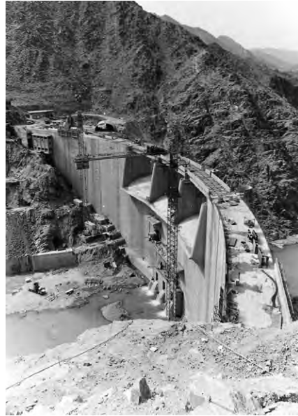
(b) Mudhiq concrete arch dam, 73 m high, Saudi Arabia. (Engineer: Binnie & Partners)
