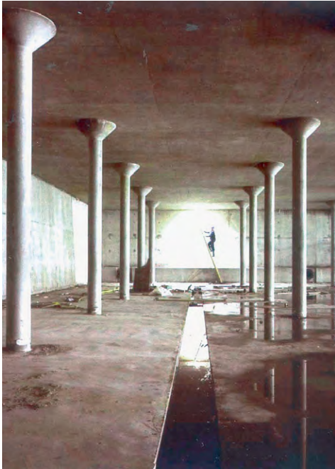
(a) Rectangular reinforced concrete monolithic service reservoir under construction in UK. (Engineer: Binnie & Partners)
