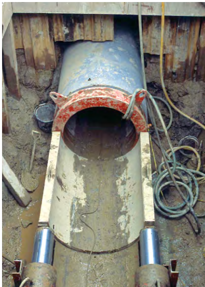
(c) Pipe jack under railway line for sleeve for 300 mm diameter trunk main. (Black & Veatch)
