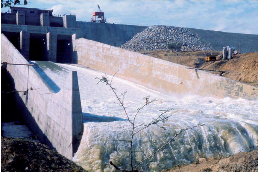
(a) Main spillway of 50 m high earth dam at Poechos, Peru—capacity 7200 m 3 /s.
