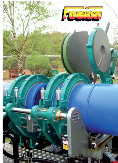
(d) Automatic butt fusion jointing of PE pipe. (Courtesy of The Fusion Group, Chesterfield, UK)
