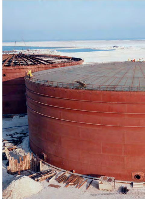
(b) 45 000 m 3 circular steel plate ground storage tanks under construction in the Middle East. (Engineer: Binnie & Partners).
