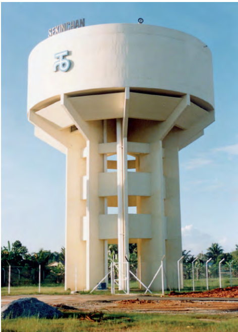
(c) 2270 m 3 reinforced concrete water tower, Malaysia. (Engineer: Binnie & Partners in association with SMHB)
