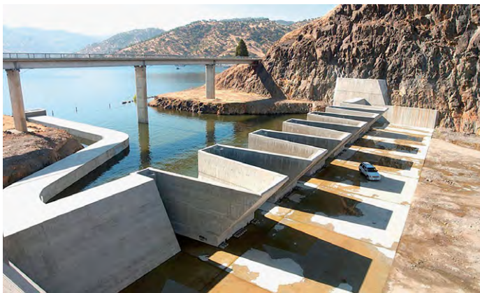
(c) Reinforced concrete labyrinth fusegates at Terminus Dam, California. Capacity 7545 m 3 /s after tipping of all gates. (Courtesy of Hydroplus, Inc, VA)
