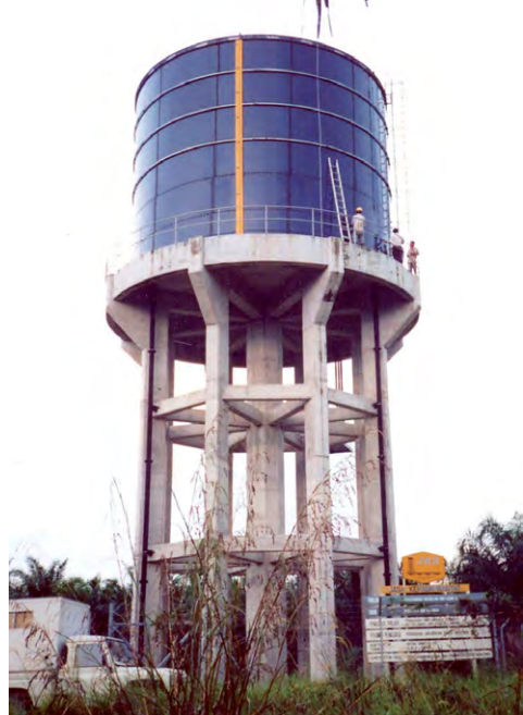
(d) 700 m 3 welded steel water tank on reinforced concrete tower, Malaysia. (Engineer: Binnie & Partners in association with SMHB)
