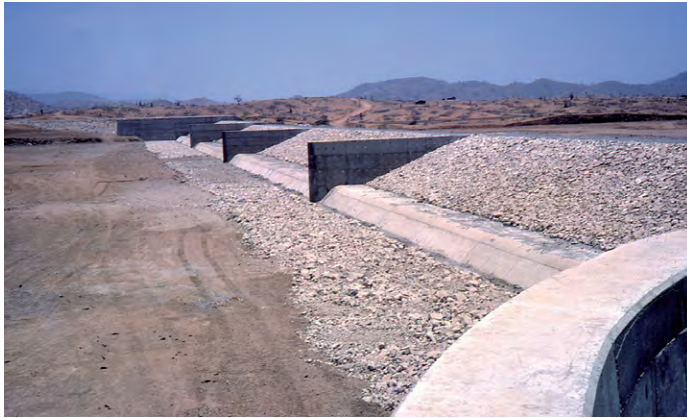
(a) 14 000 m 3 /s capacity fuse plug emergency spillway at Poechos Dam, Peru.
