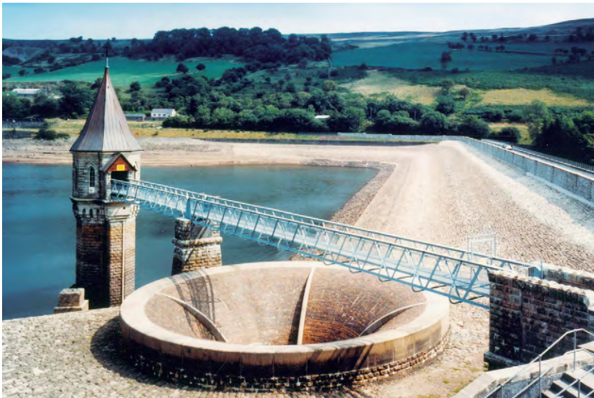
(b) Taf Fechan dam drawoff tower and bellmouth spillway, Wales. (Engineer: Sir Alex Binnie, Son & Deacon)
