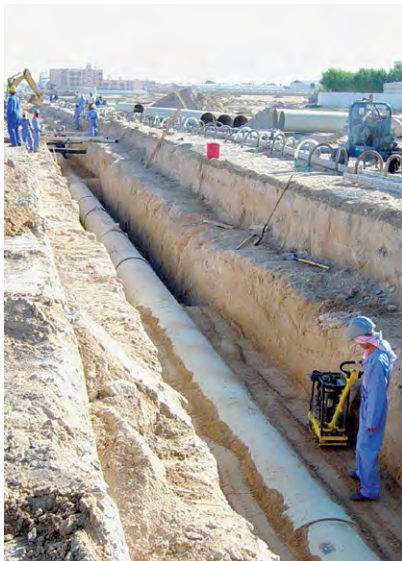
(c) 900 mm diameter GRP pipeline installation in Middle East—note attention to sidefill compaction. (Binnie Black & Veatch)
