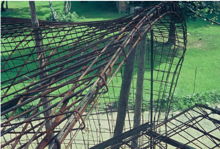
Figure 3: Steel 'girders' at the edge.
