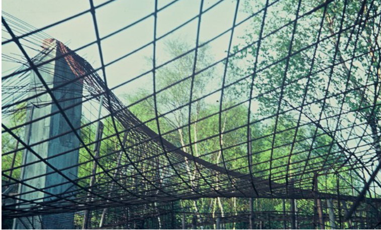
Figure 2: Steel lattice attached to the chimney.
