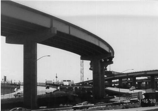
FIGURE 4.2 Steel–concrete composite I-girder bridge (I-880 Replacement, Oakland, California).
