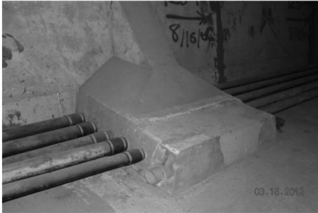
FIGURE 3.6 External tendons at deviator.
