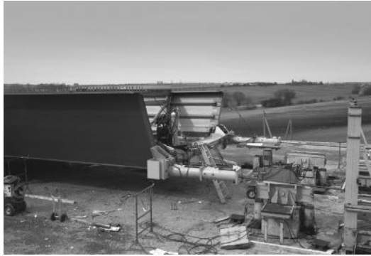
FIGURE 5.23 Short stroke hydraulic systems for lightweight superstructures in the Schrotetal Bridge (1995–1997).
