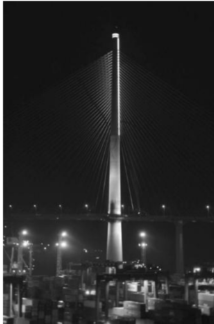
FIGURE 10.35 Stonecutters Bridge, Hong Kong S.A.R., China. Night view showing the architectural lighting on the pylon. (Courtesy of M. R. Larsen.)
