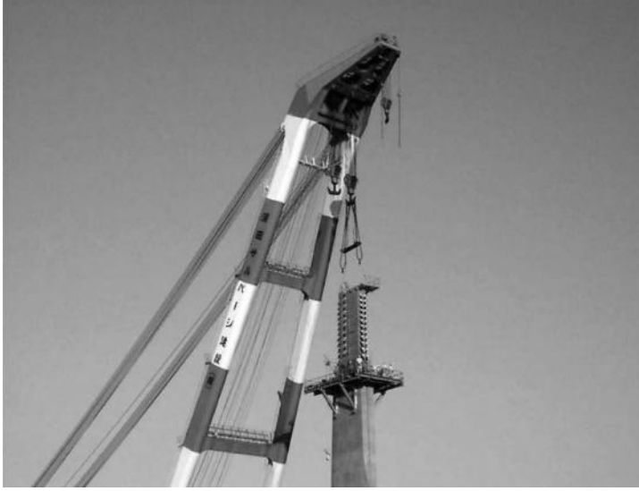
FIGURE 11.26 Anchorage box erection (Ibi River Bridge).
