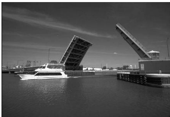
FIGURE 13.5 Nitschke (Main Street) Bridge, Green Bay, Wisconsin. (Courtesy of David Sailors.)
