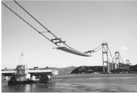
FIGURE 9.33 Block erection method on the Kurushima Bridge.
