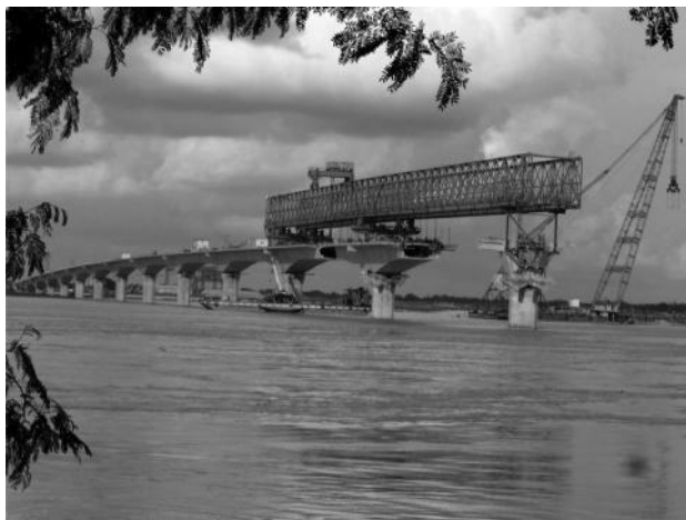
FIGURE 3.19 Segment erection with overhead launching gantry.
