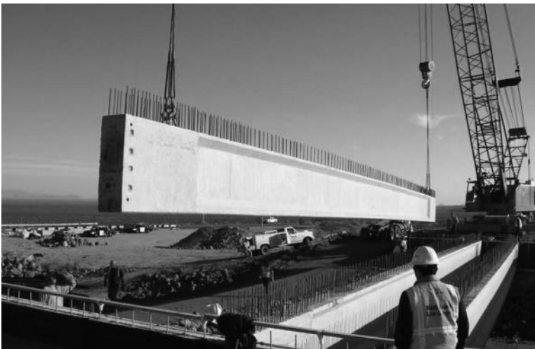
FIGURE 1.7 Single-span I beam lowered onto abutments at bridge site.
