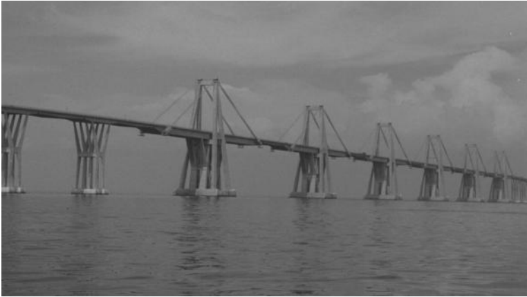
FIGURE 10.5 Maracaibo Bridge in Venezuela (General Rafael Urdaneta Bridge), completed in 1962, is an all-concrete multi-span cable-stayed bridge with five main spans of 235 m. (Courtesy of C. Añez.)
