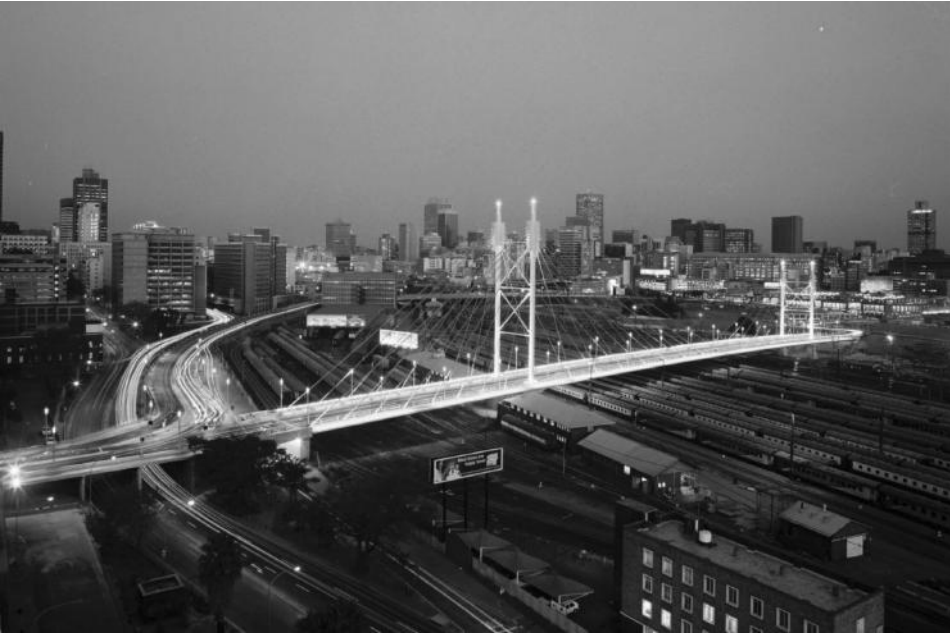
FIGURE 10.11 Nelson Mandela Bridge in Johannesburg, South Africa, completed in 2003. (Courtesy of J. Jung.)
