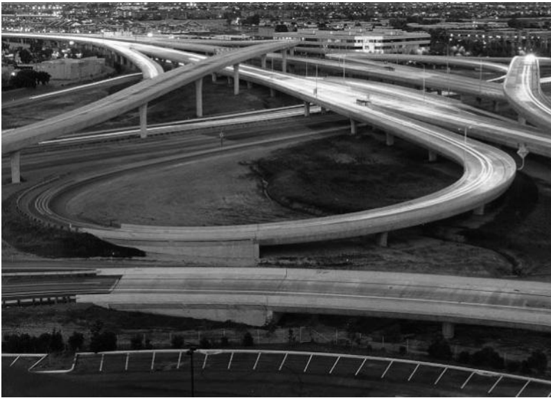
FIGURE 6.6 Curved Concrete Box Girder Bridges—Route 92/101 Interchange, San Mateo, CA.
