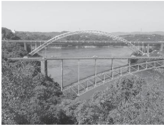
FIGURE 8.70 New Saikai Bridge, Japan: (a) elevation, (b) cross-section, and (c) completed bridge.
