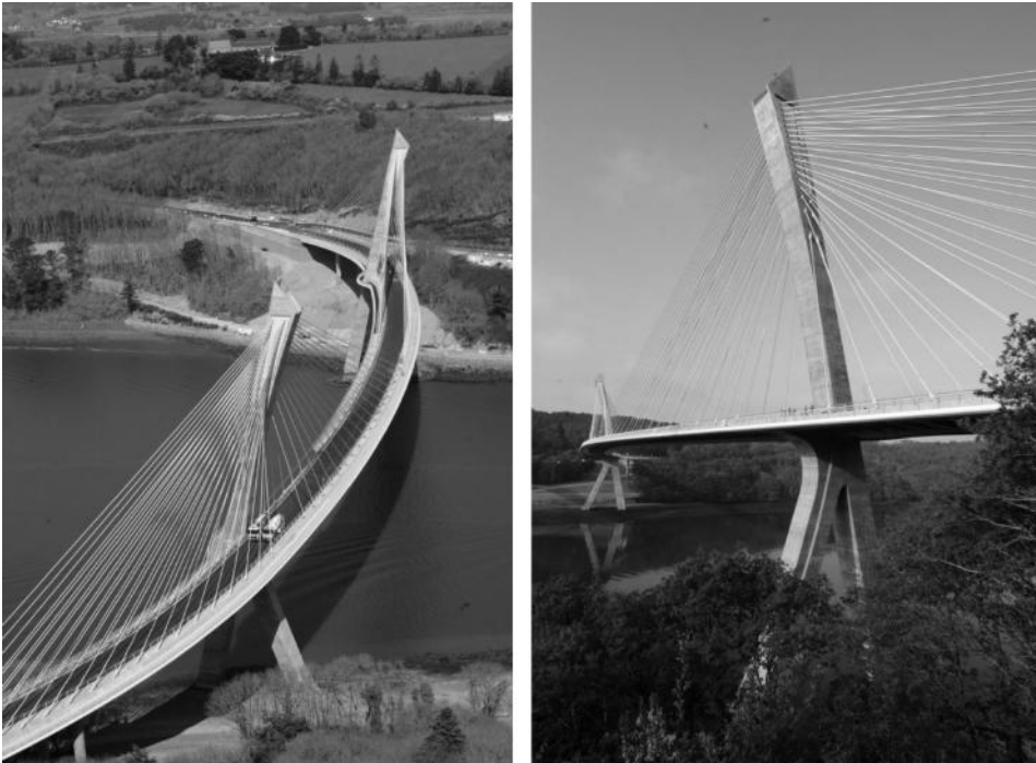
FIGURE 10.19 Térénez Bridge in France, completed in 2010. The bridge has a horizontally curved alignment with a main span of 285 m (935 ft) and carries road traffic. (Courtesy of Photothèque VINCI [F. Vigouroux].)
