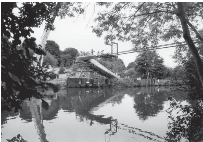
FIGURE 12.22 Bridge across the Medway River, Maidstone, Kent, UK—erection of a segment.
