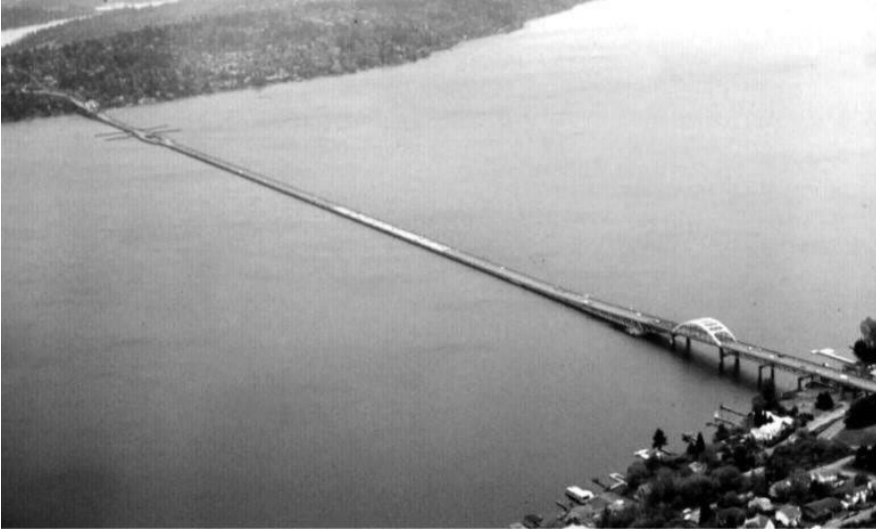
FIGURE 14.1 First Lake Washington Floating Bridge. (Courtesy of Washington State DOT.)
