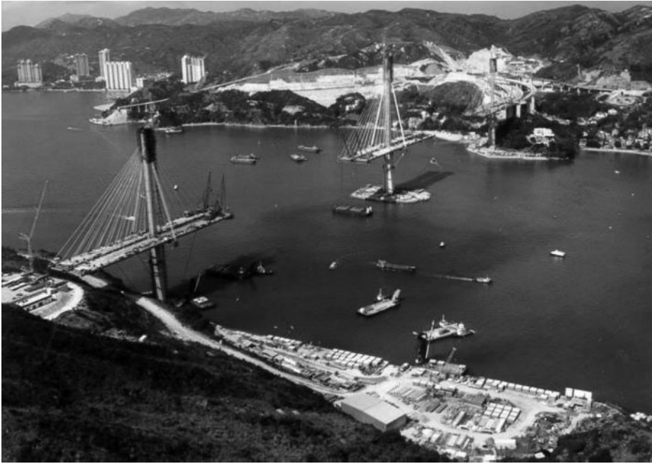
FIGURE 10.30 Ting Kau Bridge in Hong Kong S.A.R., China. The bridge has two main spans of 475 m (1558 ft) and 448 m (1470 ft), respectively. The superstructure consists of a twin deck supported by four cable planes. The bridge was completed in 1998. (Courtesy of Buckland & Taylor Ltd.)
