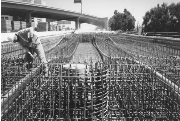
FIGURE 2.1 A posttensioned box girder bridge under construction.
