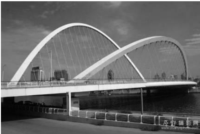
FIGURE 8.24 Dagou Bridge in Tianjin, China. (Courtesy of Zhendong Ma.)
