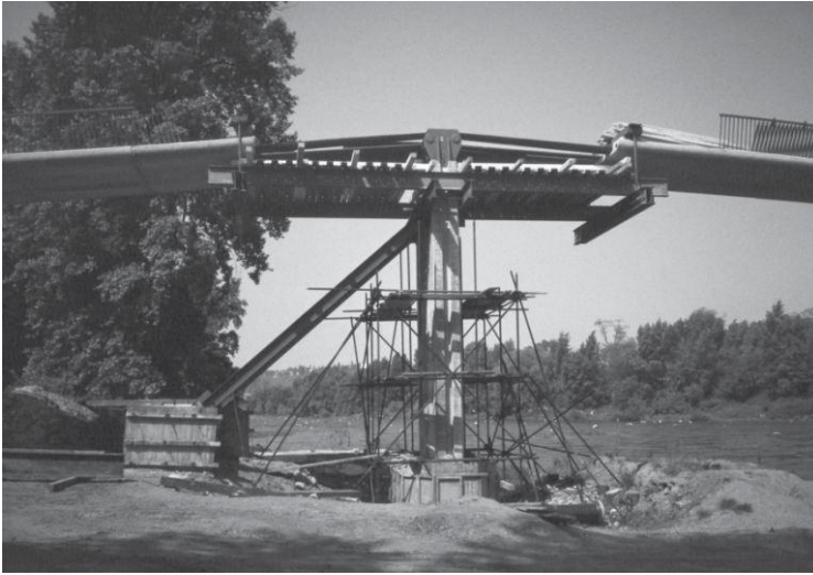
FIGURE 12.15 Prague-Troja Bridge—intermediate pier during the erection.
