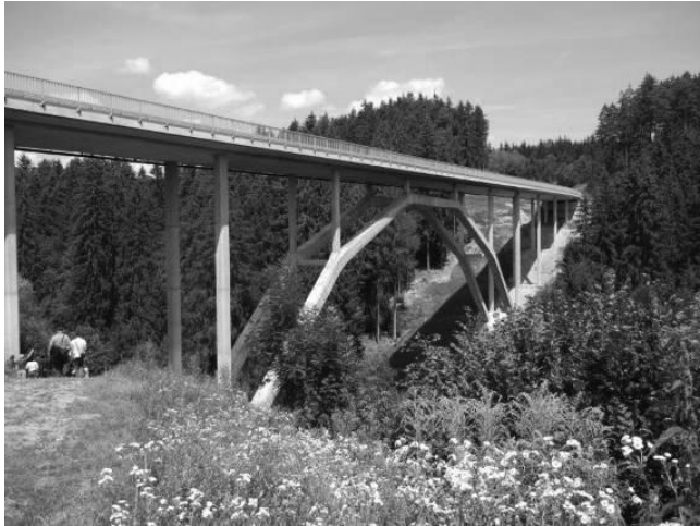
FIGURE 8.11 Wild Bridge, Austria.
