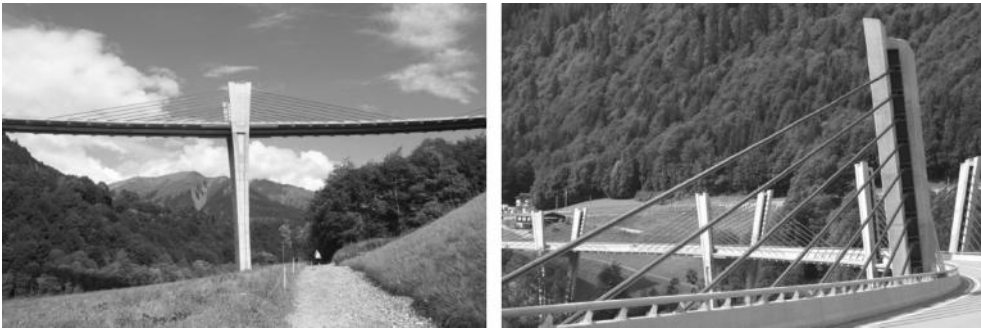
FIGURE 10.15 Sunniberg Bridge near Klosters in Switzerland was completed in 1998. The bridge is a multi-span extradosed bridge with a curved alignment. The curved alignment is clearly visible from the bridge deck (right). One of the pylons with the array of flat cables (left). (Courtesy of www.structurae.de [N. Janberg].)
