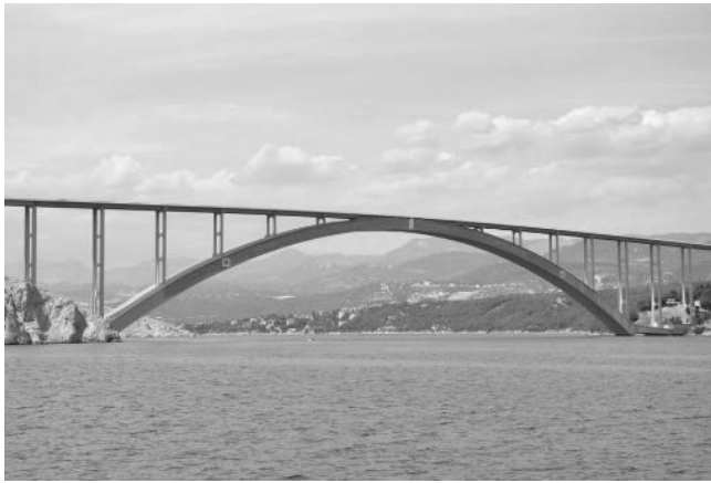
FIGURE 8.7 Krk I Bridges, Croatia. (Courtesy of Qingwei Huang.)
