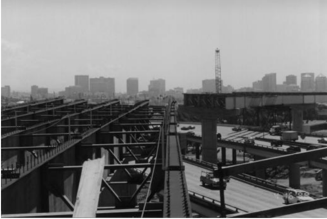
FIGURE 4.1 Steel–concrete composite I-girder bridge under construction (I-880 Replacement, Oakland, California).
