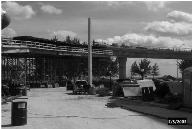
FIGURE 3.21 Cast-in-place on falsework.
