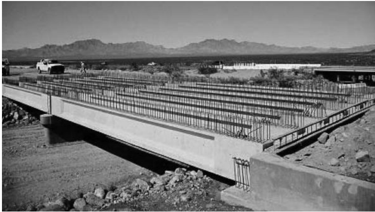
FIGURE 1.8 A typical drop cap for highway bridges.
