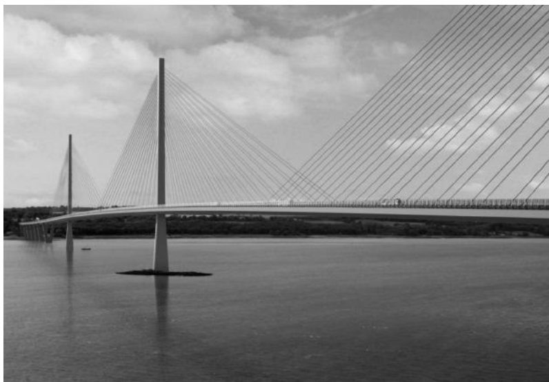
FIGURE 10.32 New Forth Crossing near Edinburgh, Scotland, scheduled for completion in 2016. Rendering showing the crossover stay cables in the two main spans. (Visualization by Knight Architects, courtesy of Forthspan and Transport Scotland.)
