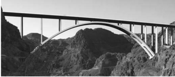
FIGURE 8.54 Mike O'Callaghan-Pat Tillman Memorial Bridge, Nevada. (Courtesy of T. Y. Lin International.)
