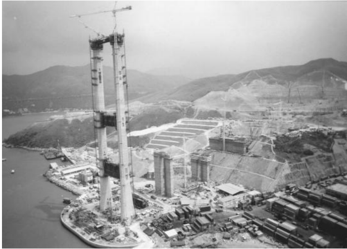
FIGURE 9.29 Tower erection for the Tsing Ma Bridge.
