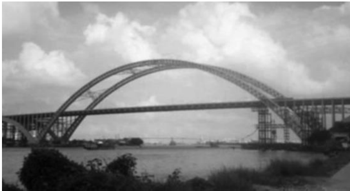
FIGURE 8.74 Ya-ji-sha Bridge in Guangzhou, China.
