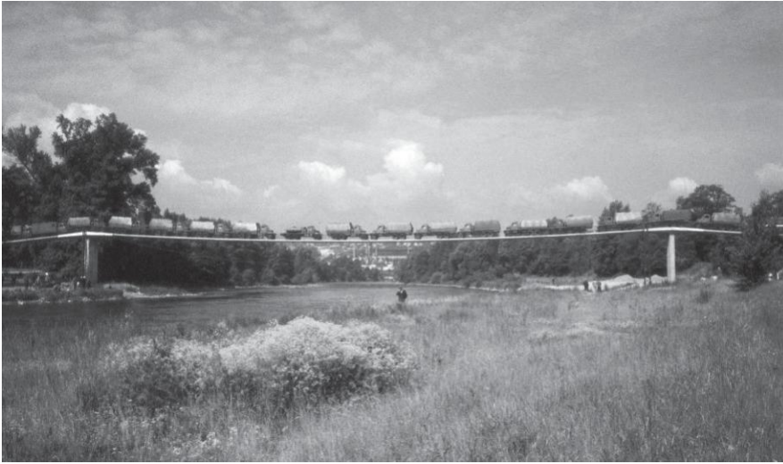
FIGURE 12.4 Loading test of the bridge across the Vltava River in Prague-Troja, Czech Republic.
