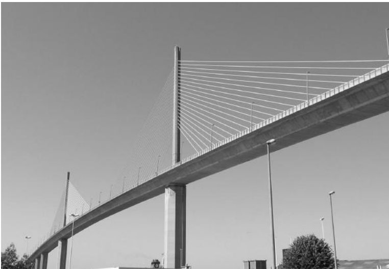
FIGURE 10.6 Brotonne Bridge across the river Seine, France, completed in 1977. The main span is 320 m and the bridge is an all-concrete structure. (Courtesy of P. Bourret.)
