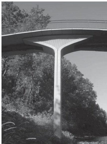
FIGURE 12.14 Grants Pass Pedestrian Bridge—intermediate pier.
