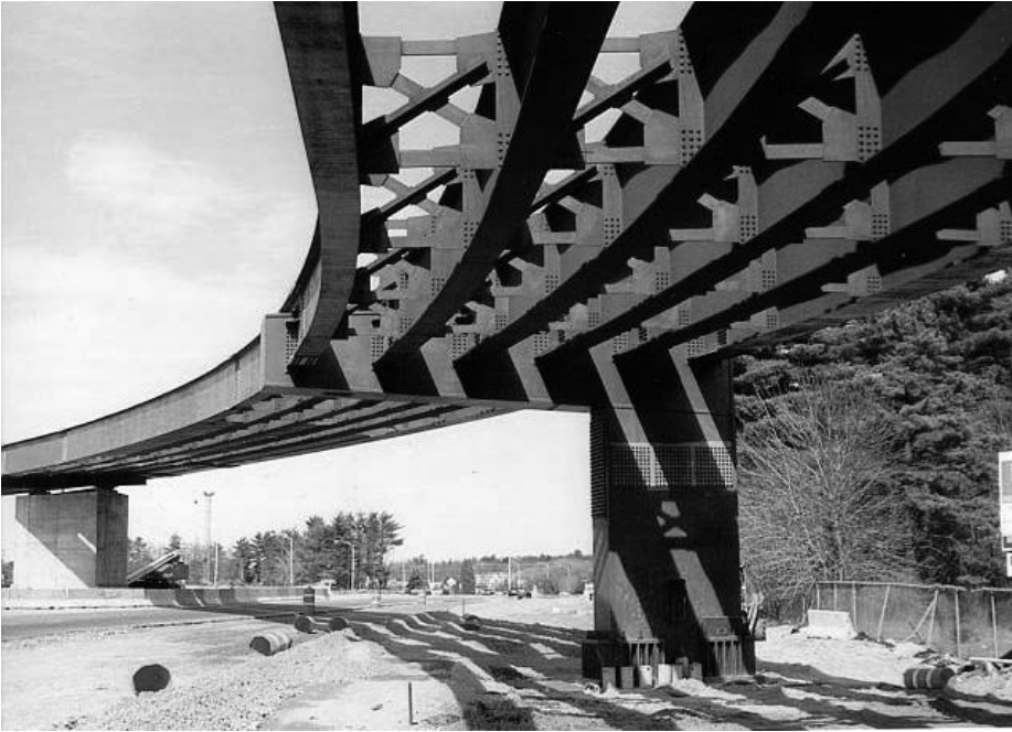
FIGURE 6.1 Curved I-girder bridge under construction—20th Street HOV, Denver, CO.
