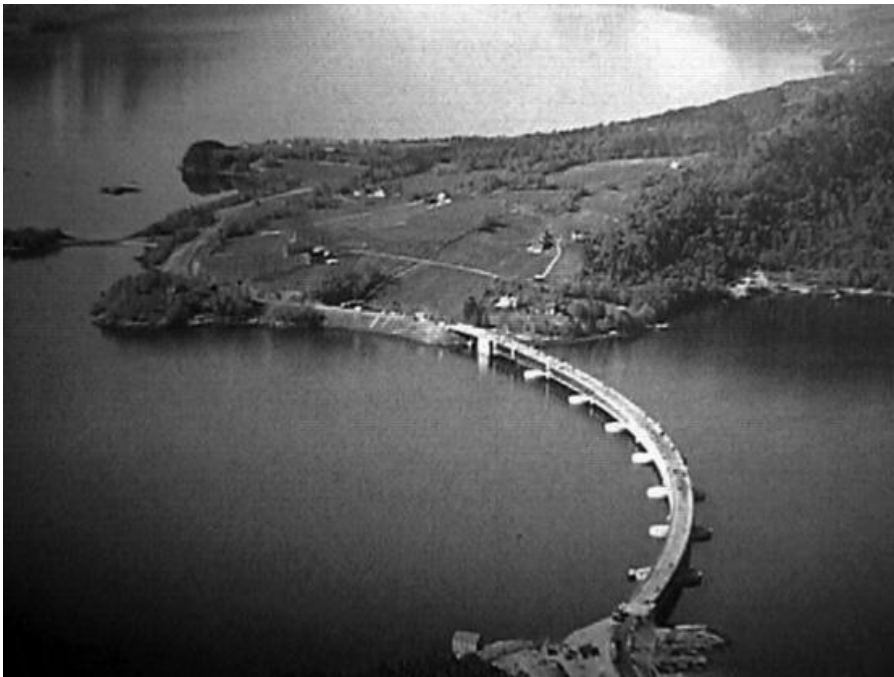
FIGURE 14.2 The Bergsoysund Floating Bridge.
