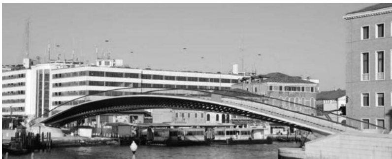
FIGURE 8.22 Fourth Grand Canal Bridge in Venice, Italy.
