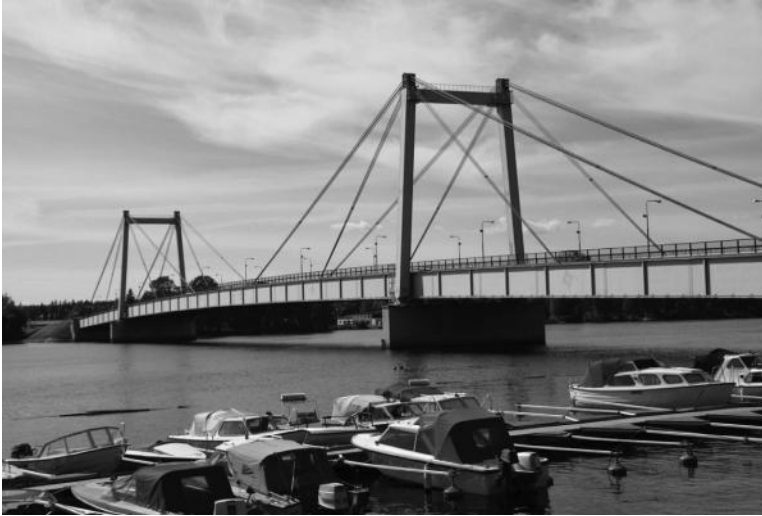
FIGURE 10.2 Strömsund Bridge, Sweden, completed in 1955. The main span is 182.6 m (599 ft) and the stay cables are arranged in a pure fan system. Pylons and stiffening girders are in steel. (Courtesy of www.pwpeics.se [P. Wählin].)
