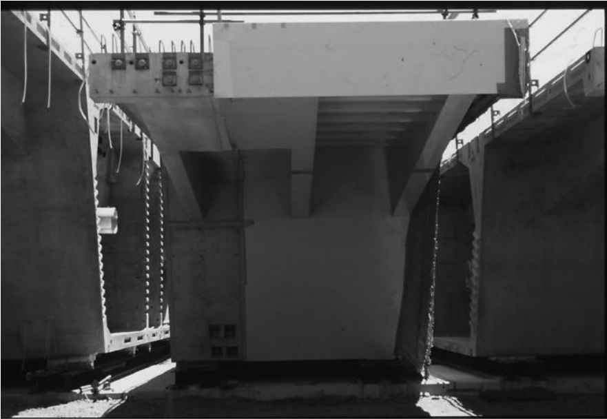
FIGURE 11.11 Connection segment (Ibi River Bridge).
