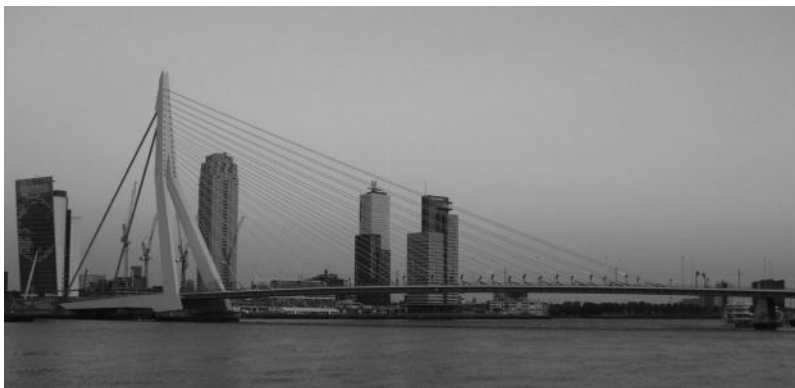
FIGURE 10.23 The Erasmus Bridge in Rotterdam, the Netherlands, completed in 1996. The bridge features a single, kinked pylon with a height of 139 m (456 ft). (Courtesy of COWI A/S [M. B. Jensen].)
