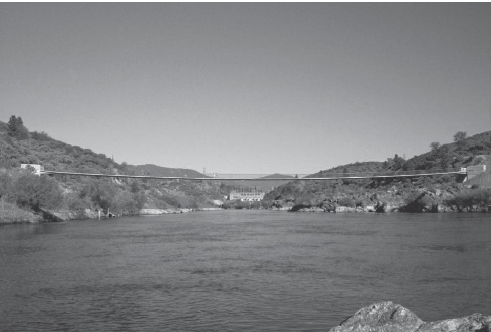
FIGURE 12.2 Bridge across the Sacramento River in Redding, CA.
