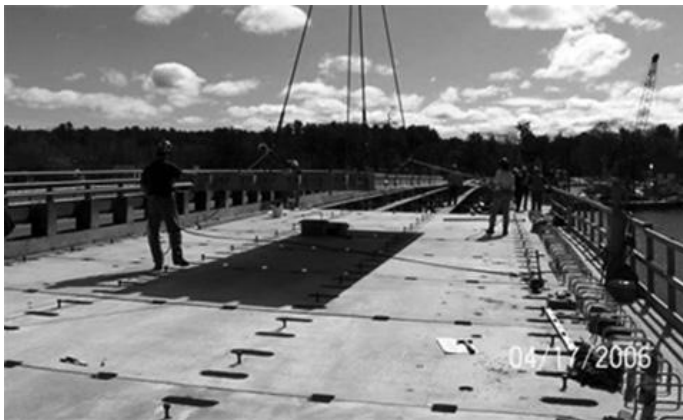
FIGURE 15.4 Full-depth precast concrete deck panels under construction. (Courtesy of FHWA.)
