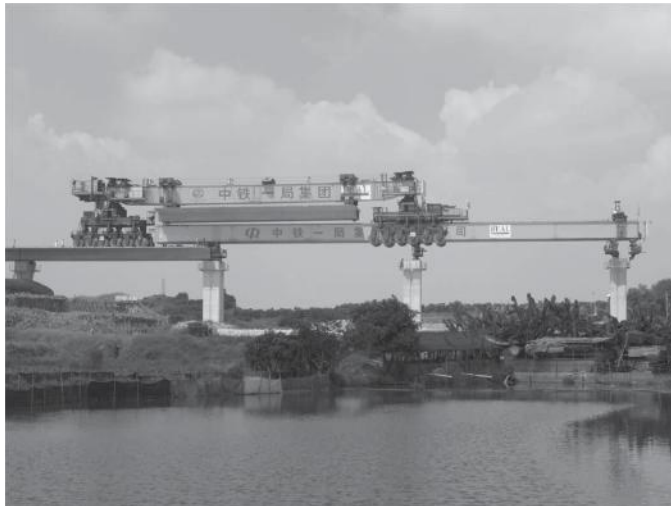
FIGURE 3.30 Full-span girder erection. (Courtesy of DEAL.)
