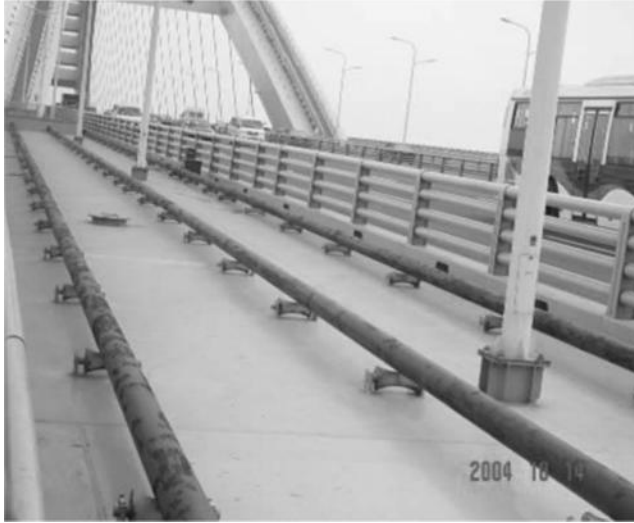
FIGURE 8.69 Tie bars on Lupu Bridge deck.
