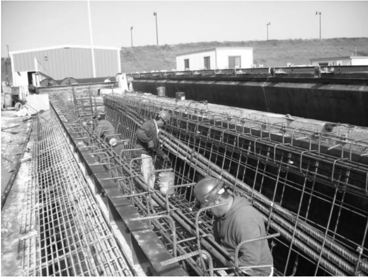
FIGURE 1.1 Precast bathtub girder (with posttensioned ducts) in pretensioning bed.
