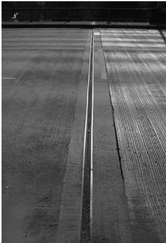
FIGURE 18.13 Elastomeric strip seal application.
