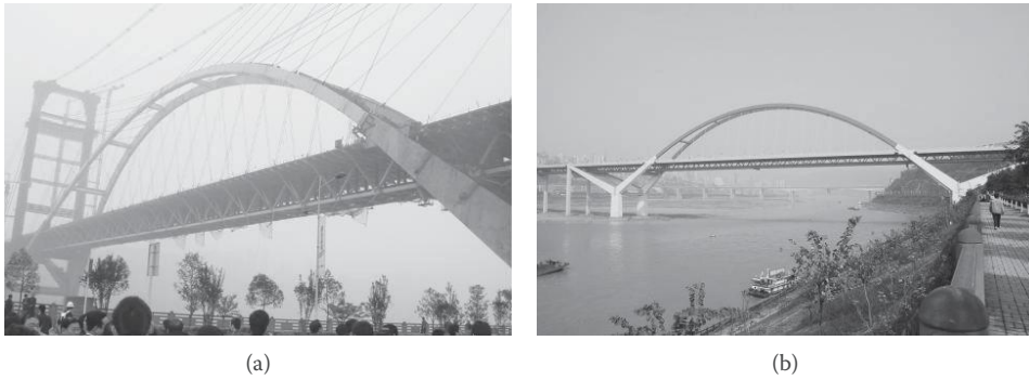
FIGURE 8.44 Caiyuanba Yangtze River Bridge in Chongqing, China: (a) in construction (Courtesy of Qingxiang WU) and (b) completed bridge.
