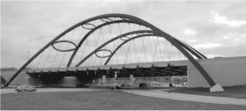
FIGURE 8.66 Gateway Bridge in Michigan. (Courtesy of M. Kasi.)
