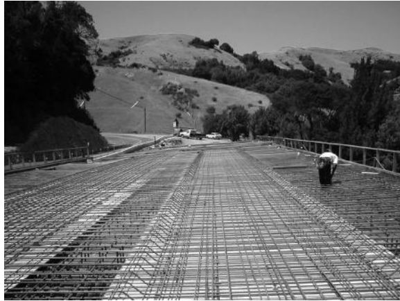
FIGURE 15.1 Reinforcement layout in a cast-in-place concrete deck.
