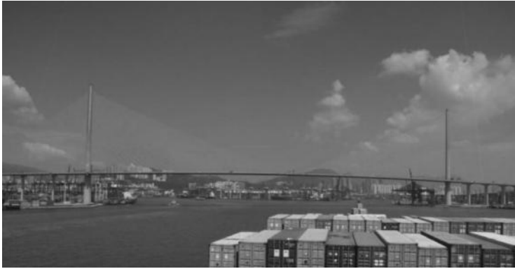
FIGURE 10.26 Stonecutters Bridge, Hong Kong S.A.R., China. The bridge with a main span of 1018 m (3340 ft) was completed in 2009. (Courtesy of M. R. Larsen.)
