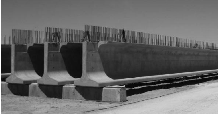
FIGURE 1.2 California wide-flange girder.
