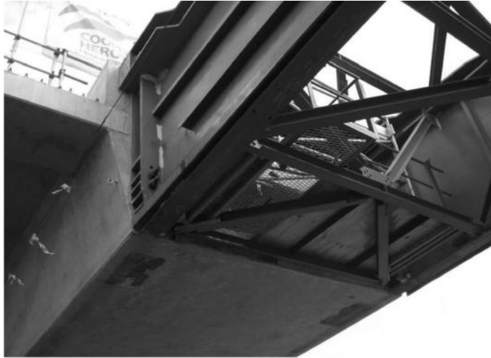
FIGURE 3.26 Launching nose and segment connection. (Courtesy of C2HC Alliance, Australia.)
