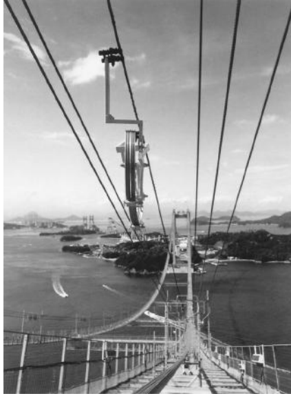
FIGURE 9.32 Aerial spinning for the Shimotsui-Seto Bridge.
