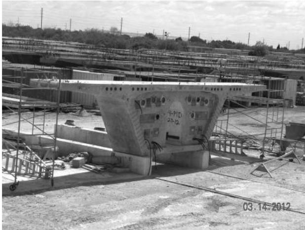
FIGURE 3.17 Segments storage site.
