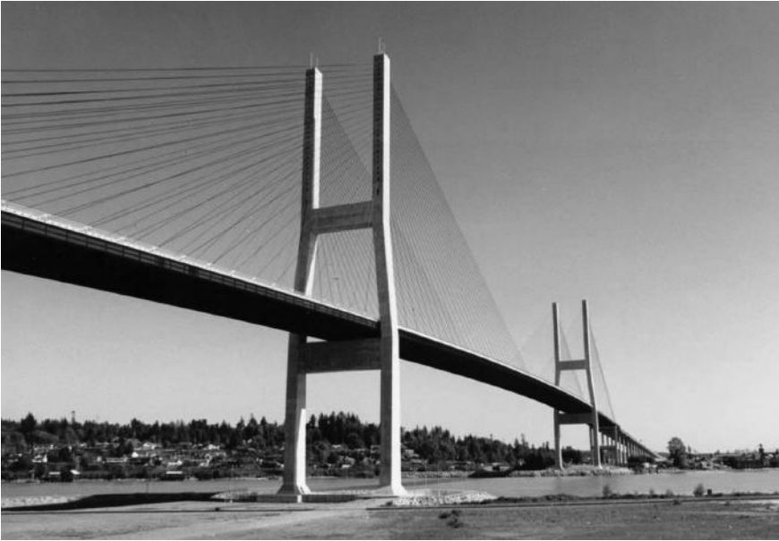
FIGURE 10.7 Alex Fraser Bridge in Vancouver, Canada, has a composite main span of 465 m (1526 ft). The bridge was completed in 1986. (Courtesy of Buckland & Taylor Ltd.)
