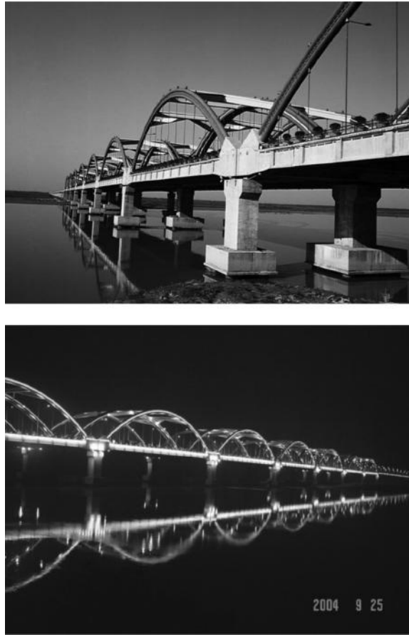
FIGURE 8.71 Second Yellow River Highway Bridge in Zhengzhou, China.
