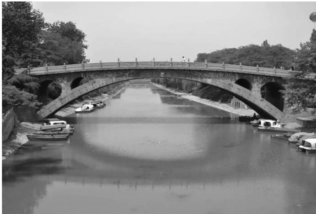
FIGURE 8.3 Zhaozhou Bridge, China.
