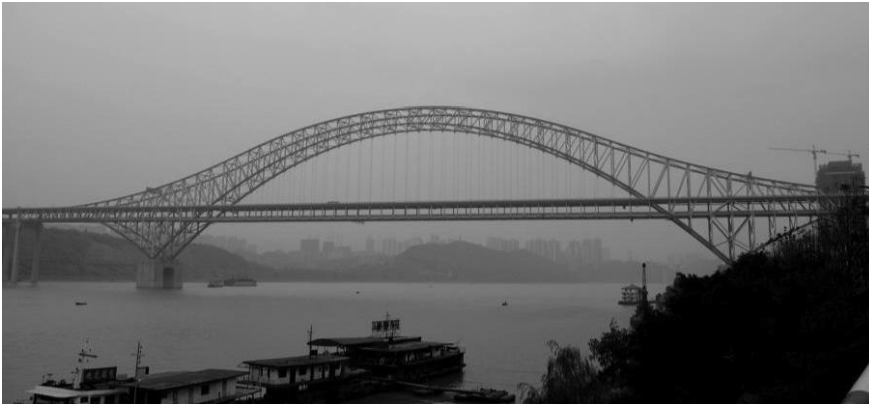
FIGURE 8.9 Chaotianmen Bridge, China. (Courtesy of Zhongfu Xiang.)
