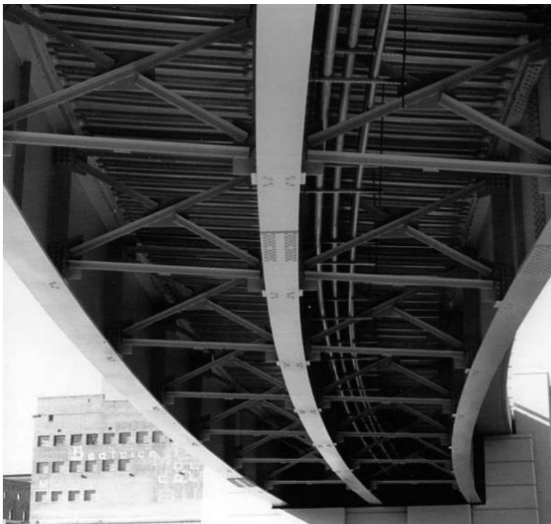
FIGURE 6.2 Bottom view of curved I-girder bridge.
