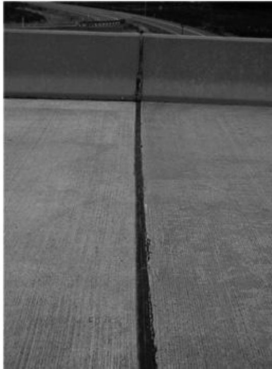
FIGURE 18.4 Elastomeric compression seal application.
