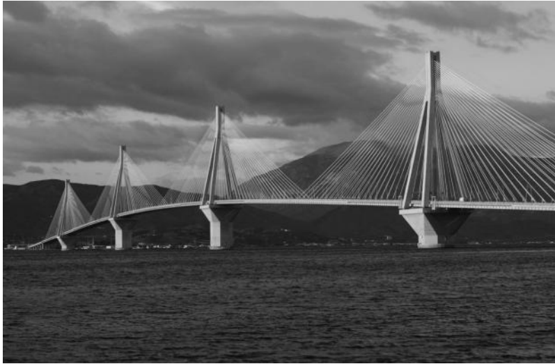
FIGURE 10.28 The Rion-Antirion Bridge in Greece, completed in 2004. The bridge has three main spans of 560 m (1837 ft). (Courtesy Photothèque VINCI [C. Dupont].)
