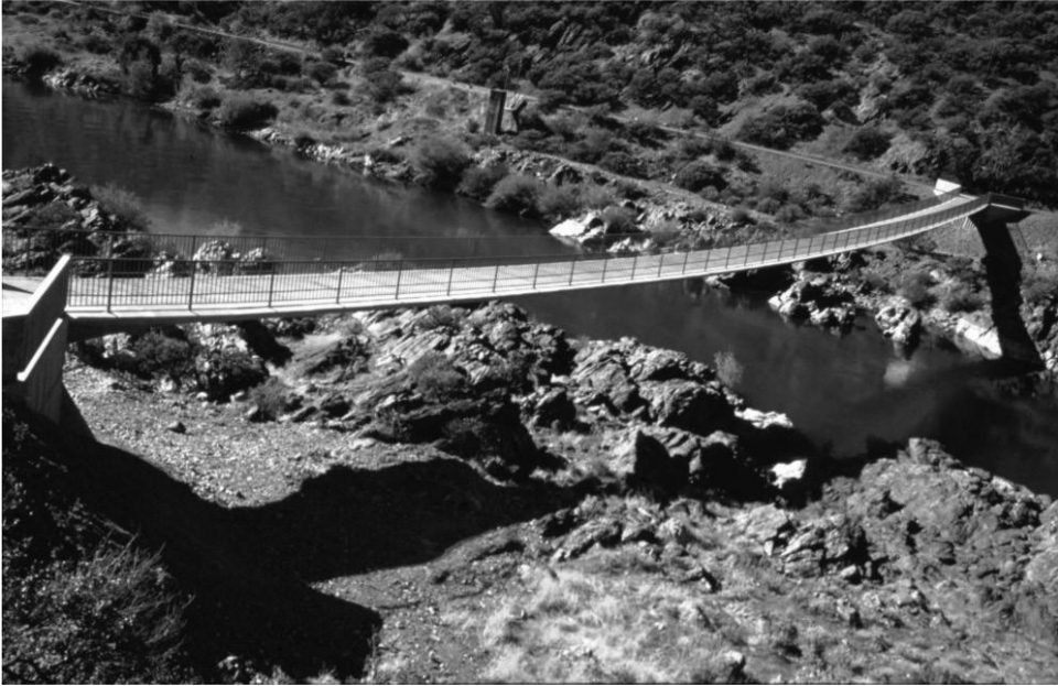
FIGURE 12.41 Redding Bridge—completed structure (slide).
