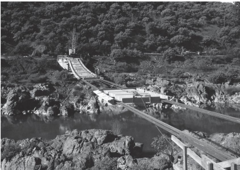
FIGURE 12.3 Erection of the bridge across the Sacramento River in Redding, CA.
