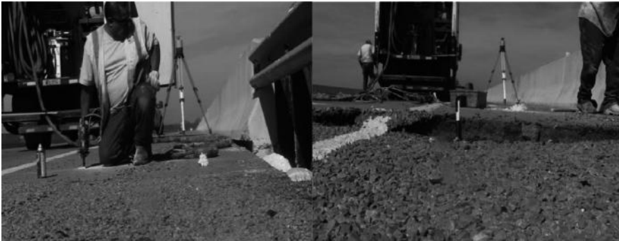
FIGURE 17.11 Position of approach slab during and after the urethane injection process.
