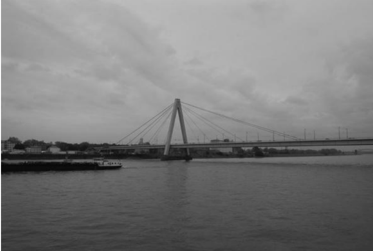
FIGURE 10.4 Severins Bridge across the Rhine River in Cologne, Germany, completed in 1961. Main span 302 m (991 ft). (Courtesy of S. Prinzler.)
