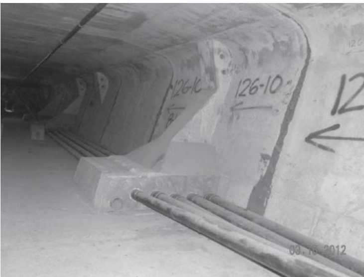
FIGURE 3.23 Typical deviator.
