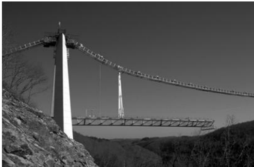
FIGURE 5.23 Short stroke hydraulic systems for lightweight superstructures in the Schrotetal Bridge (1995–1997).
