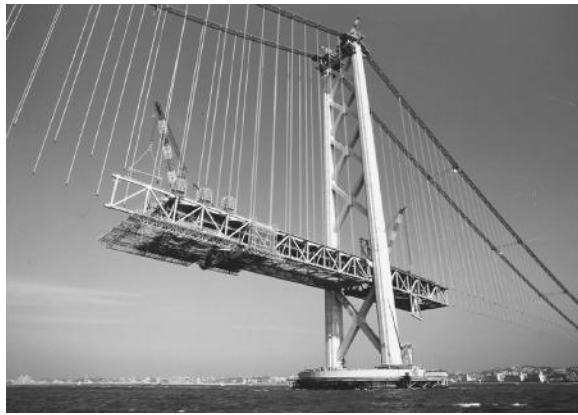
FIGURE 9.34 Cantilevering method in the Akashi Kaikyo Bridge.
