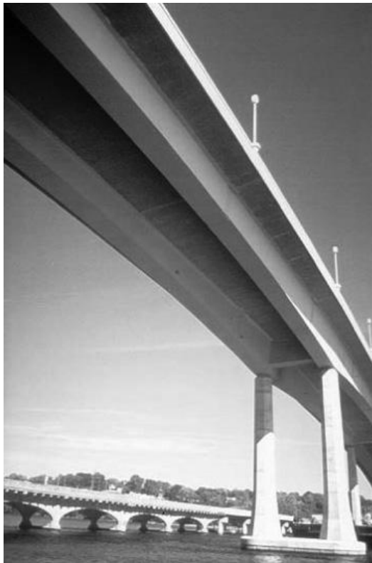
FIGURE 6.4 Twin box girder bridge—United States Naval Academy Bridge, Annapolis, MD.
