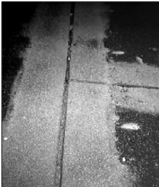
FIGURE 18.9 Poured sealant application.
