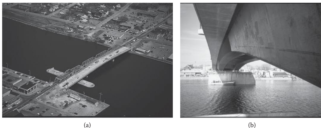
FIGURE 5.25 Trenton, Ontario 1993. (a) Aerial view of bridge. (b) Bottom view of bridge.
