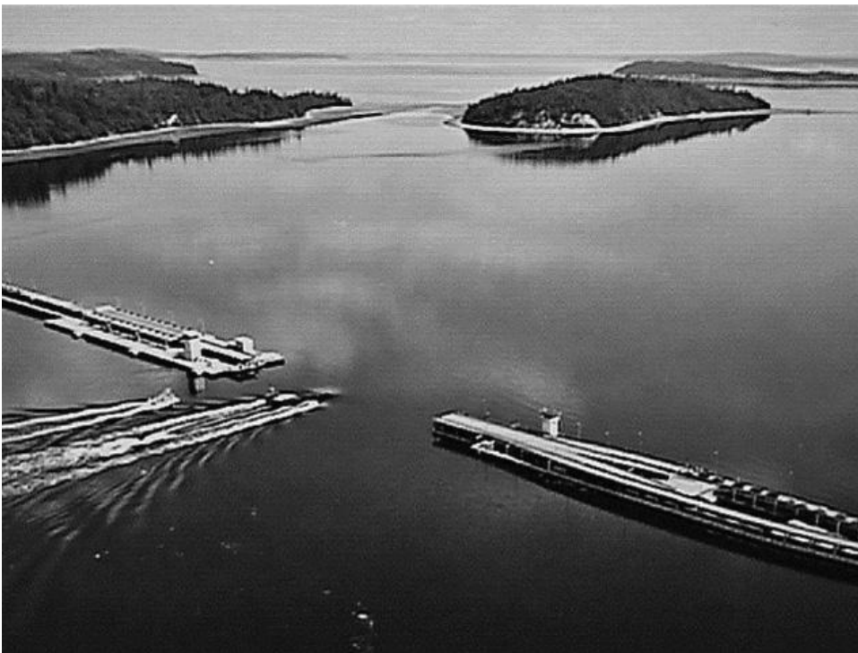
FIGURE 14.3 Movable spans for large vessels.
