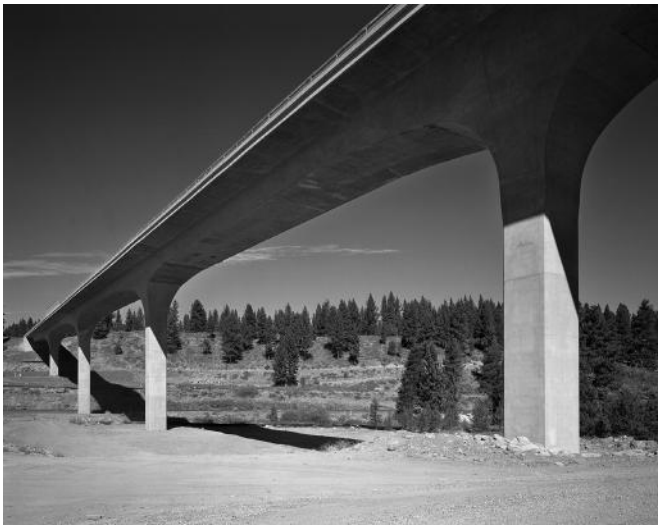
FIGURE 2.7 Truckee River Bridge, California. (Courtesy of California Department of Transportation.)
