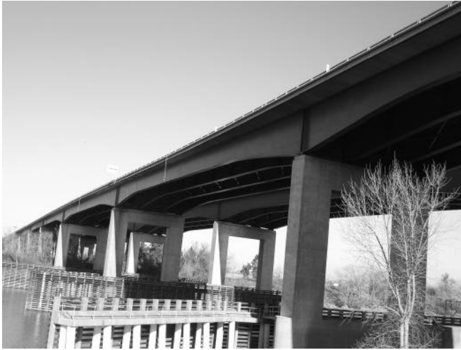
FIGURE 4.7 A haunched steel continuous girder bridge (U.S. 50 Bridge over Sacramento River).
