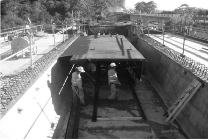
FIGURE 3.25 Casting form. (Courtesy of C2HC Alliance, Australia.)
