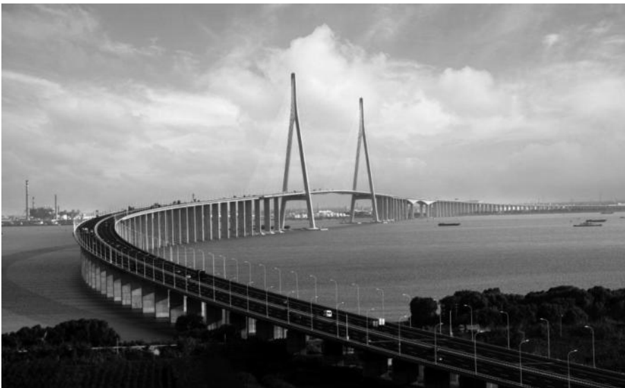
FIGURE 10.25 Sutong Bridge over the Yangtze River, China, completed in 2008. The main span is 1088 m (3570 ft). (Courtesy of Sutong Bridge Co. Ltd.)
