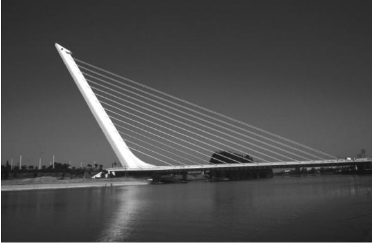
FIGURE 10.9 Alamillo Bridge in Seville, Spain. Arranged with a main span of 200 m (656 ft) and no side span or backstays. Completed in 1991. (Courtesy of www.pwpeics.se [P. Wählin].)
