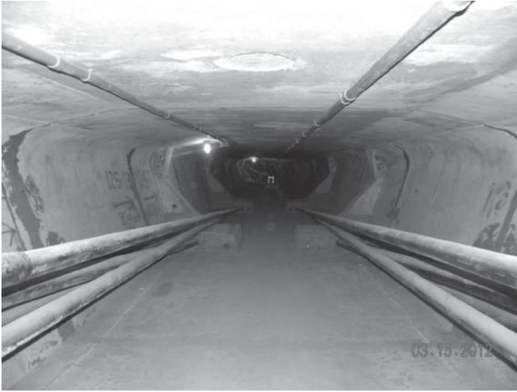
FIGURE 3.22 External tendons inside a box girder.
