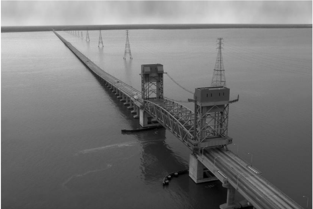
FIGURE 13.13 James River Bridge, Virginia (photo). (Courtesy of David Sailors.)
