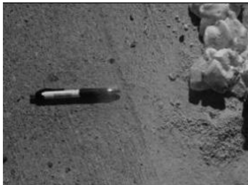
FIGURE 17.12 Hairline crack observed on the approach slab during the urethane injection.
