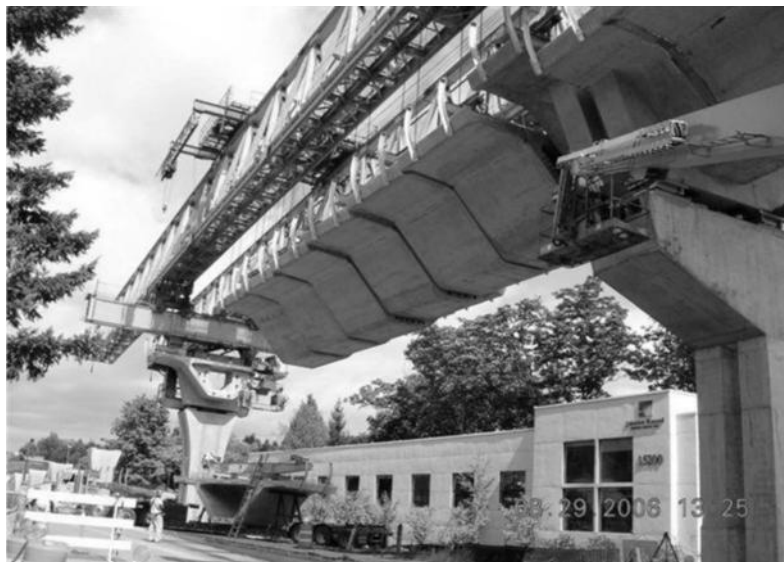
FIGURE 3.24 Span-by-span segment erection using overhead gantry.
