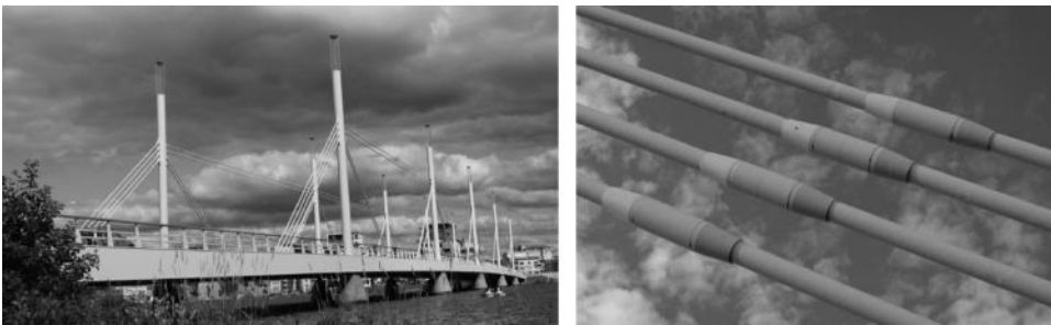
FIGURE 10.31 Munksjön Bridge in Sweden, completed in 2006. The central pylons are stabilized by horizontal top stays. The stay cables are fabricated from solid bars in high strength steel joined by couplers into the required length (refer to detail to the right). (Courtesy of COWI A/S [H. E. Jensen].)
