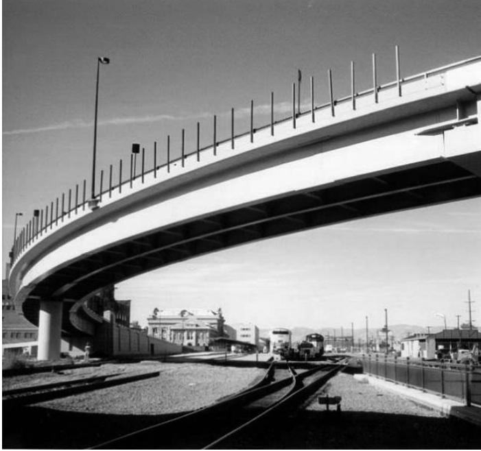
FIGURE 6.3 Curved I-girder bridge with integral bent cap.
