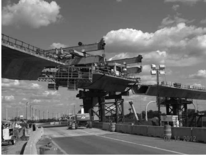
FIGURE 3.20 Segment erection with segment lifter.
