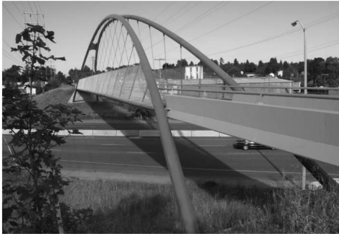
FIGURE 12.55 McLoughlin Bridge, OR.
