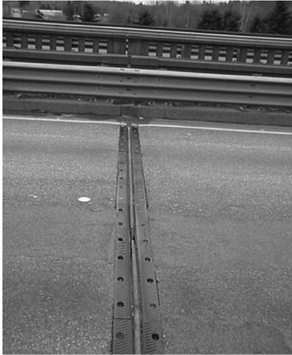
FIGURE 18.11 Bolt-down panel application.
