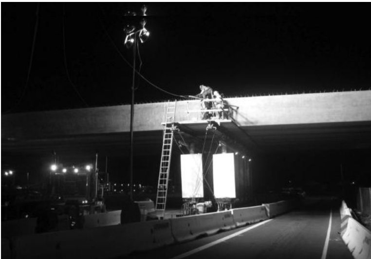
FIGURE 1.10 Precast bathtub girder segments spliced near midspan using temporary supports at Harbor Blvd. OC in California.
