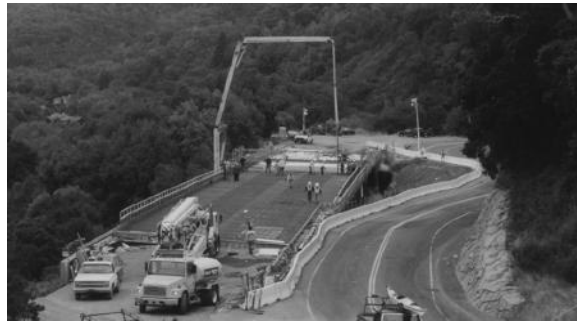
FIGURE 15.2 A cast-in-place concrete deck under construction.
