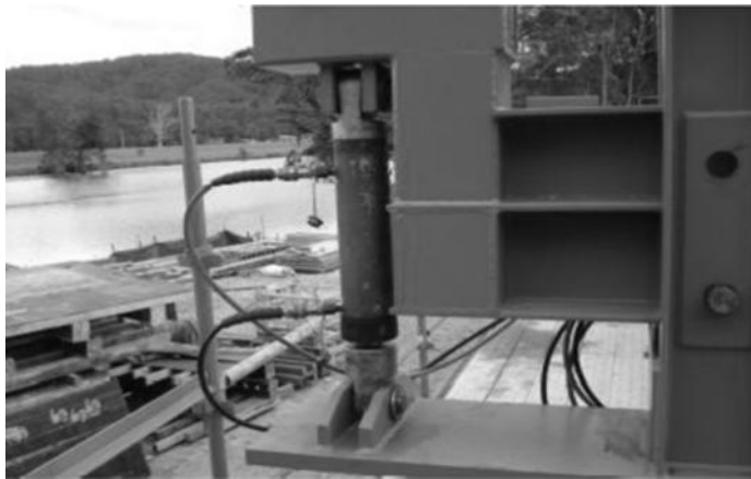
FIGURE 3.27 Hydraulic jack at launching nose's tip. (Courtesy of C2HC Alliance, Australia.)
