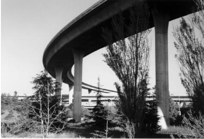
FIGURE 2.6 Prestressed box girder bridge (I-280/110 Interchange, California).
