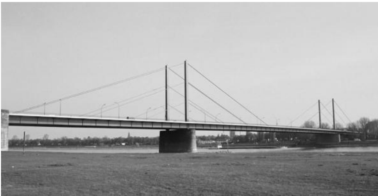
FIGURE 10.3 The Theodor Heuss Bridge across the Rhine River in Düsseldorf, Germany (also known as the North Bridge). Completed in 1957, the bridge has a main span of 260 m (853 ft) and the stay cables are arranged in a harp system. (Courtesy of www.structurae.de [N. Janberg].)
