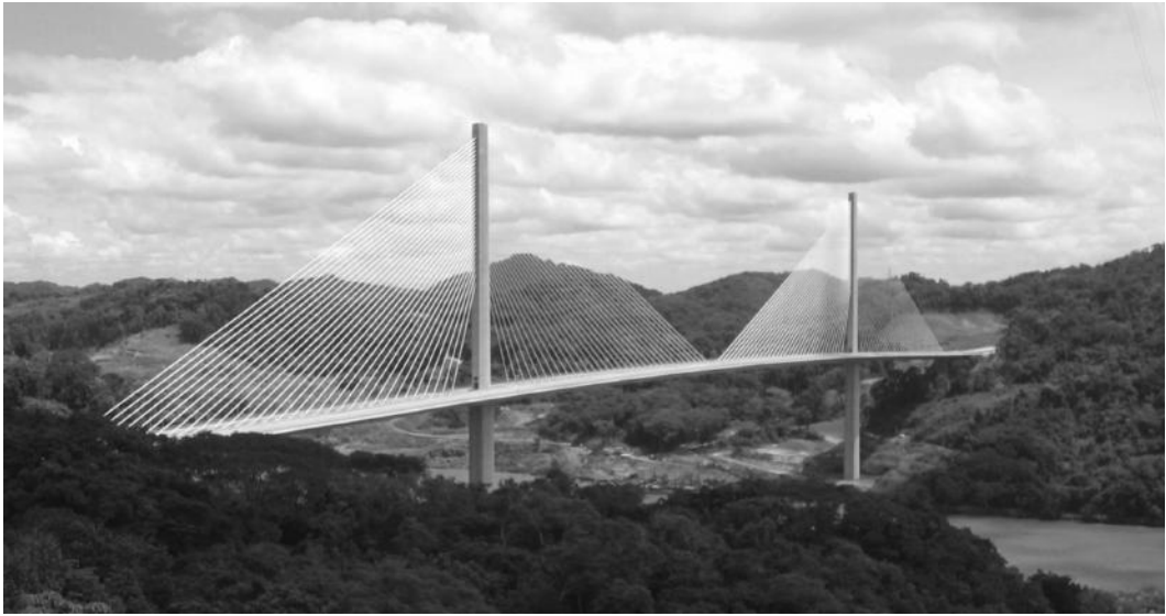
FIGURE 10.17 Second Bridge across the Panama Canal (Puente Centenario), completed 2004. The main span is 420 m (1378 ft). (Courtesy of COWI A/S [K. Fuglsang].)
