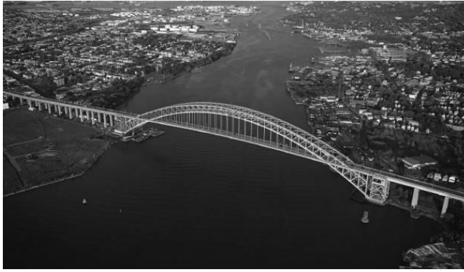
FIGURE 8.6 Bayonne Bridge, New York/New Jersey. (Copyright Keith Pholpott. Photo courtesy of HDR.)
