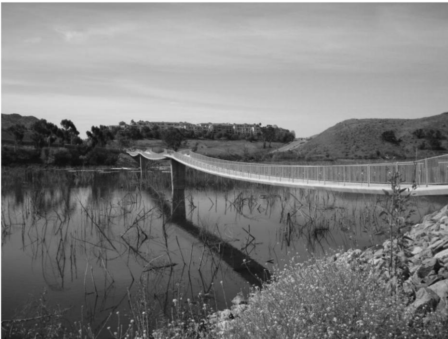
FIGURE 12.43 Lake Hodges Bridge, CA.
