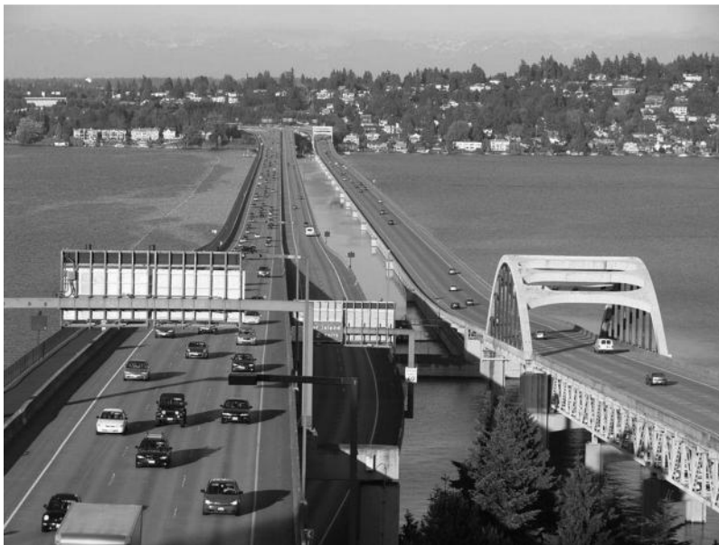
FIGURE 14.19 Floating bridges on Lake Washington. (Courtesy of Washington State DOT.)
