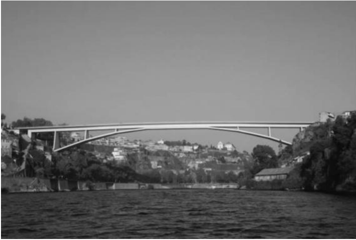
FIGURE 8.59 Infante Dom Henrique Bridge in Porto, Portugal.
