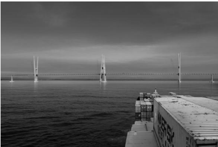
FIGURE 10.34 Proposed bridge solution for the Fehmern Belt Fixed Link: Multi-span cable-stayed bridge with two main spans of 724 m (2375 ft) carrying two tracks of railway on the lower deck and four lanes of road traffic on the upper deck. (Visualization by Dissing + Weitling, courtesy of Femern Bælt A/S.)
