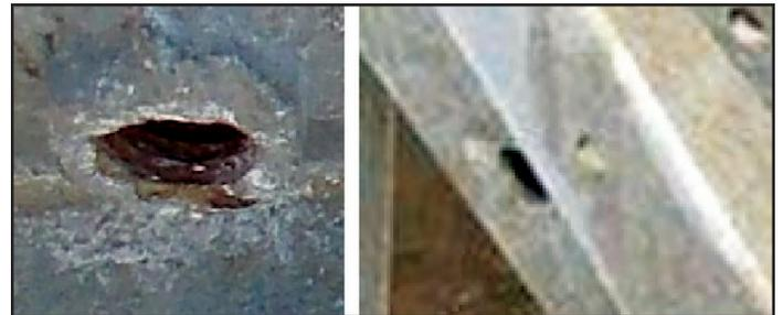
Figure 3: Damaged Bolt Holes Of Pinned Connections
