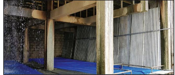
Picture Set 1.7: Placement of corrugated galvanized sheets along the cell boundary
