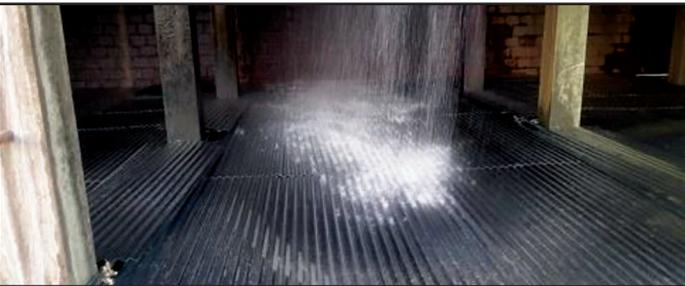
Picture Set 1.4: Placement of corrugated galvanized sheets
