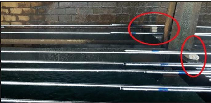
Picture Set 1.3: Use of bricks to create inclination
