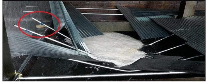
Picture Set - 2.3: Deficient number of pipes
