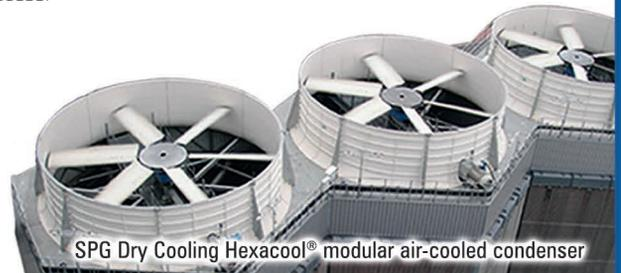
SPG Dry Cooling Hexacool<sup>®</sup> modular air-cooled condenser
