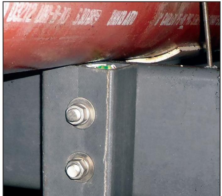
Figure 1: Excessive Compression On Unsupported Frp Structural Tubing
