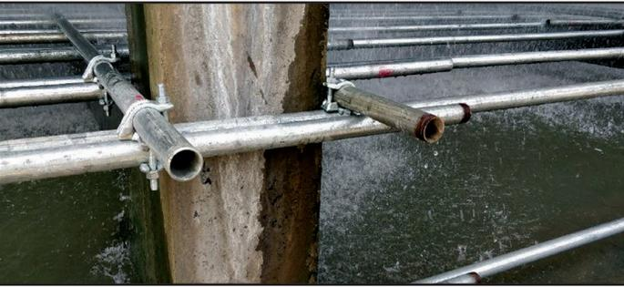
Picture Set 1.2: Connection between two pipes using galvanized clamps
