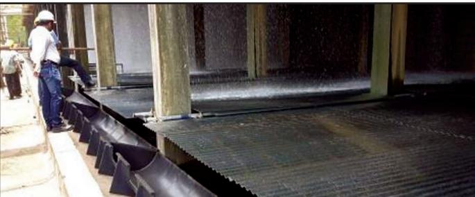
Picture Set 1.5: Placement of water collection troughs
