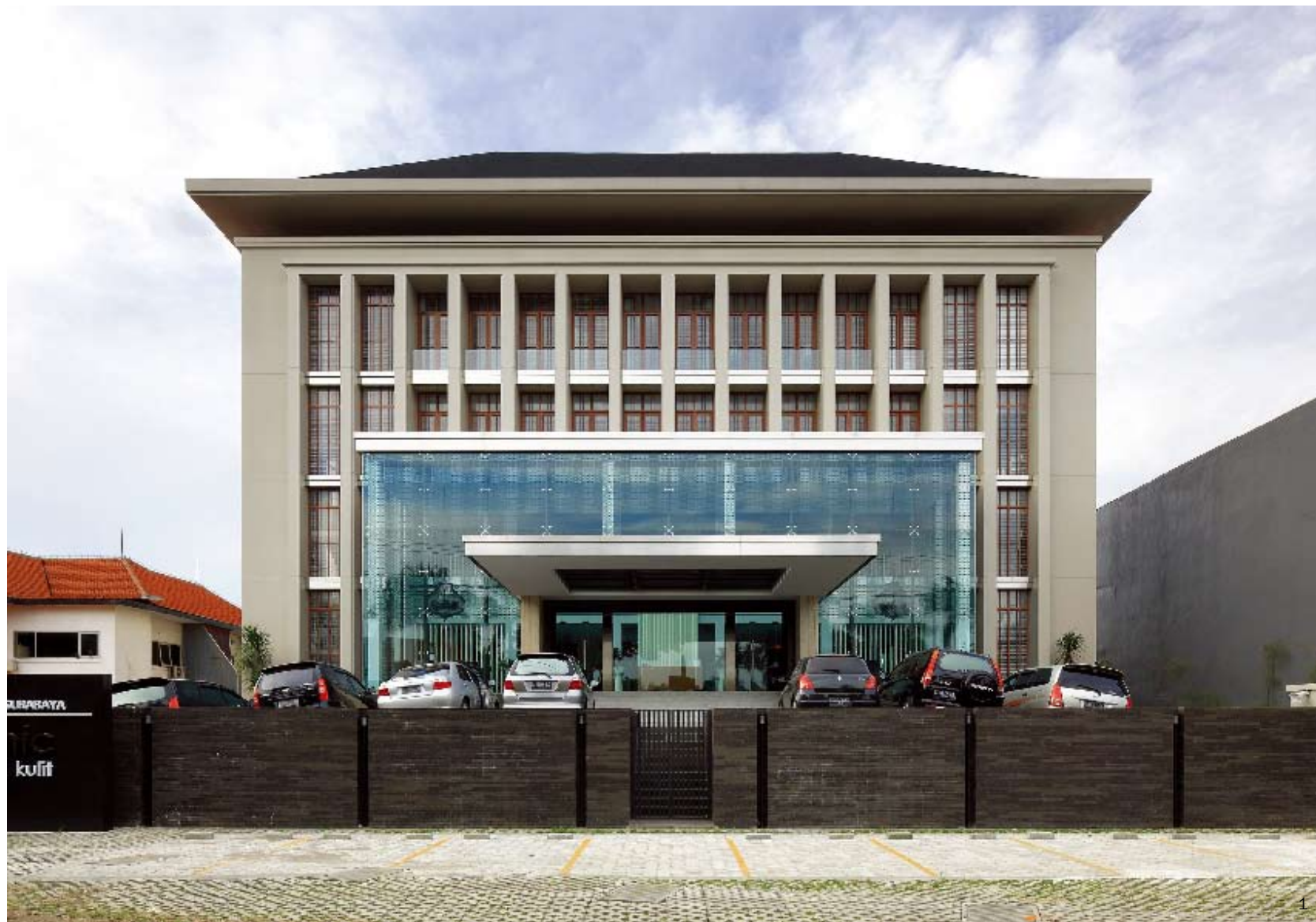
1. The building is quite symmetrical 2. The elegant and luxurious interior design
