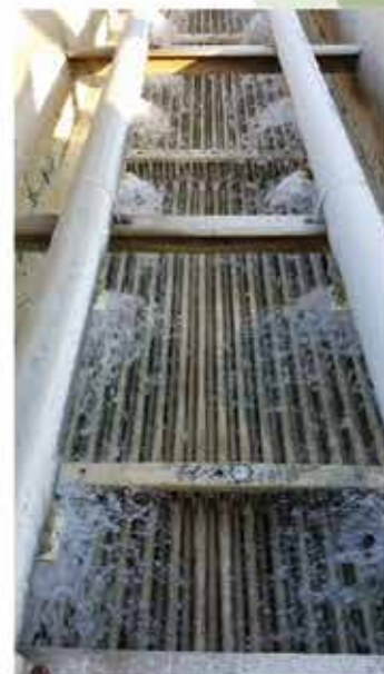
Poor Water Distribution
