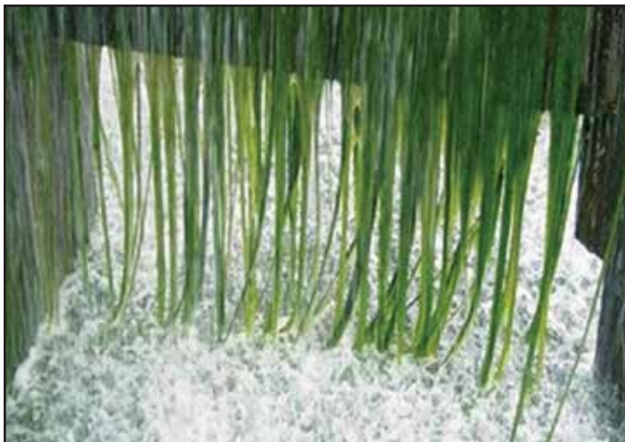
Figure 3: Algae hanging from cooling tower fill
