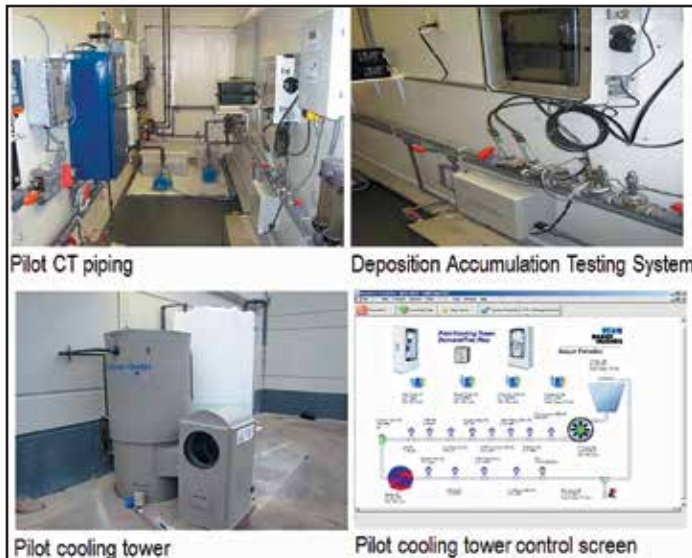
Fig. 2: Pilot test unit including the piping, deposition accumulation test system (DATS), pilot cooling tower and pilot cooling tower control screen.
