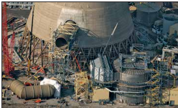
Fig 11 FGD Construction
