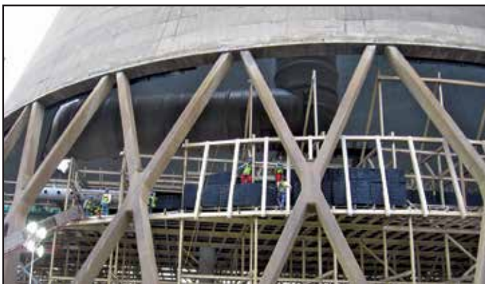
Fig 10 Counterflow Conversion Work in Progress
