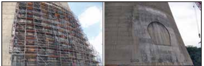
Fig 6 Concrete Shell Flue Duct Opening Reinforcement
