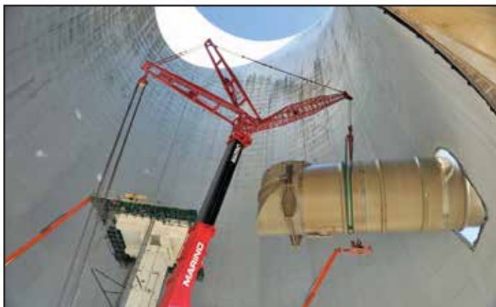
Fig 9 Installing Fiberglass Flue Duct
