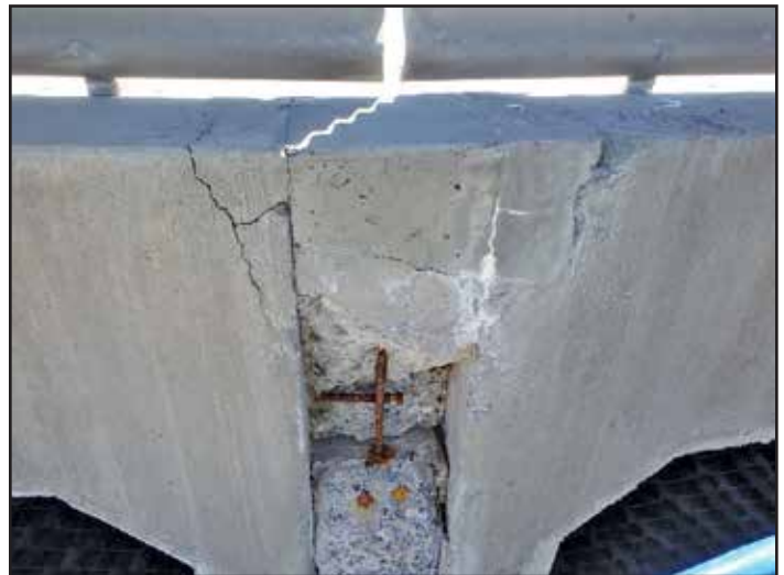
Figure 6: Spalled Concrete in Cooling Tower
