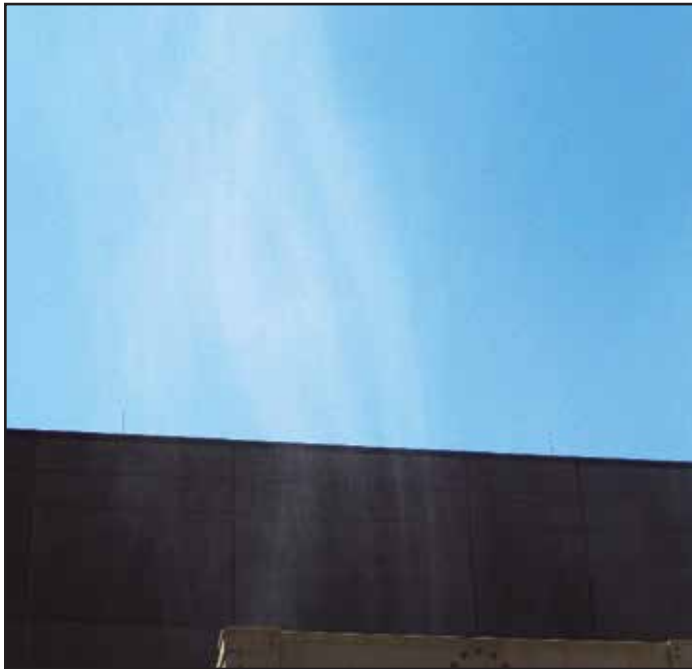
Figure 2: Picture of a drift issue with DE being within their operating limits.
