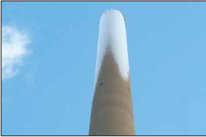
Fig 13 Old Stack Icing
