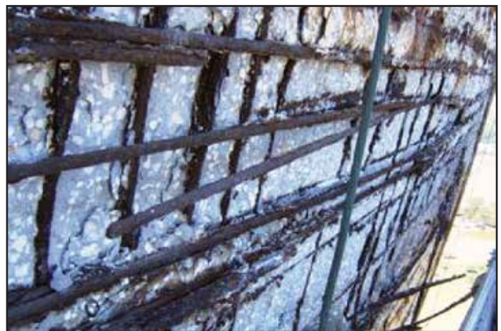
7: Cooling Tower Shell - Extensive Spalling Caused Delamination of Concrete with Exposed Corroded Reinforcing Bars
