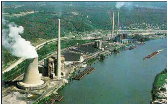
Fig 1. Cardinal Plant Prior to FGD Retrofit
