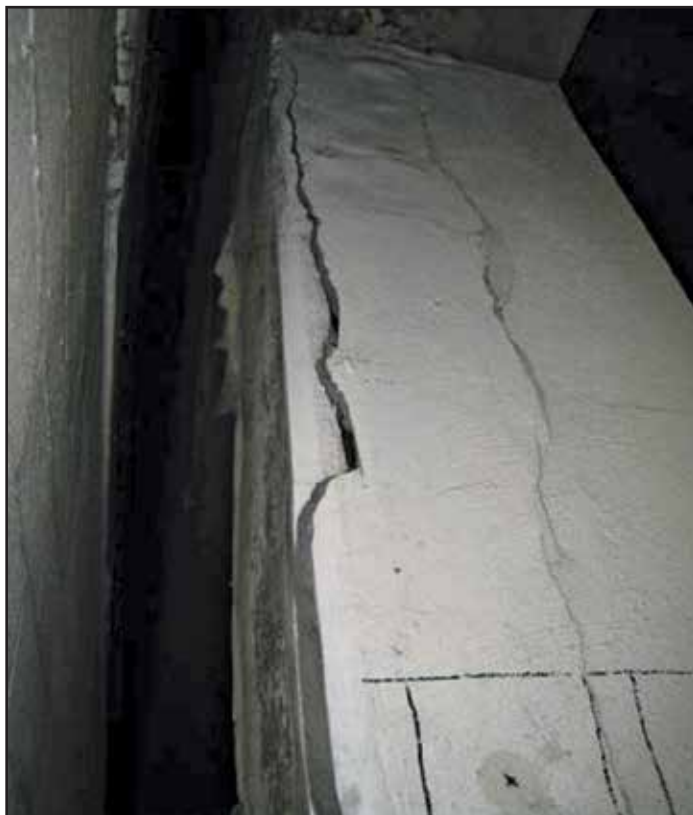
Figure 4: Cracking of Concrete due to Corrosion
