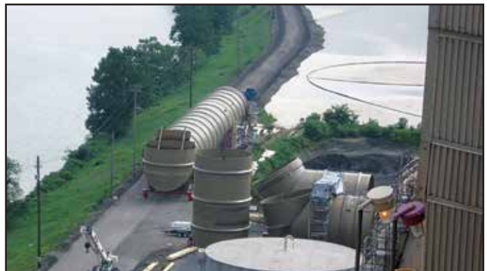
Fig 7 FGD Duct Pre Outage Work
