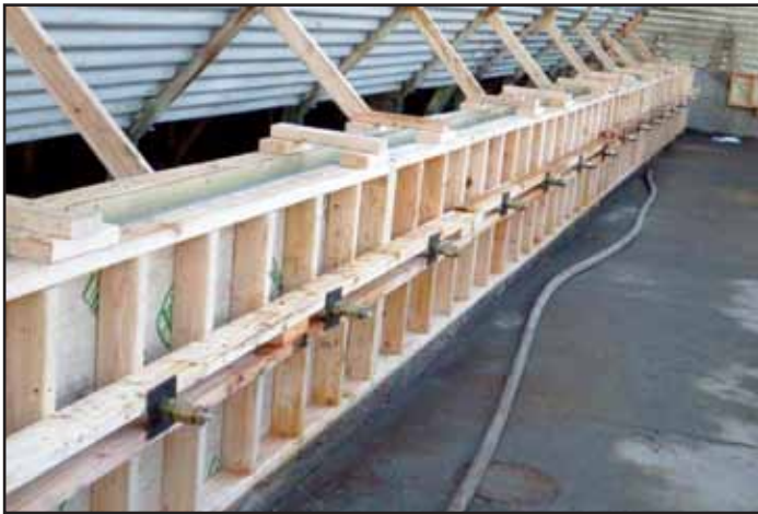
Figure No. 11 Excavation of deteriorated Basin Wall concrete materials.
