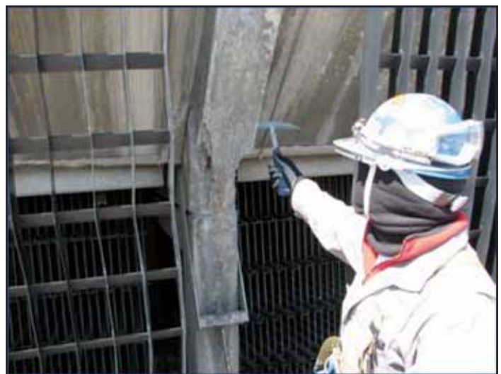
Figure No. 2 Hammer sounding of concrete member repairs.
