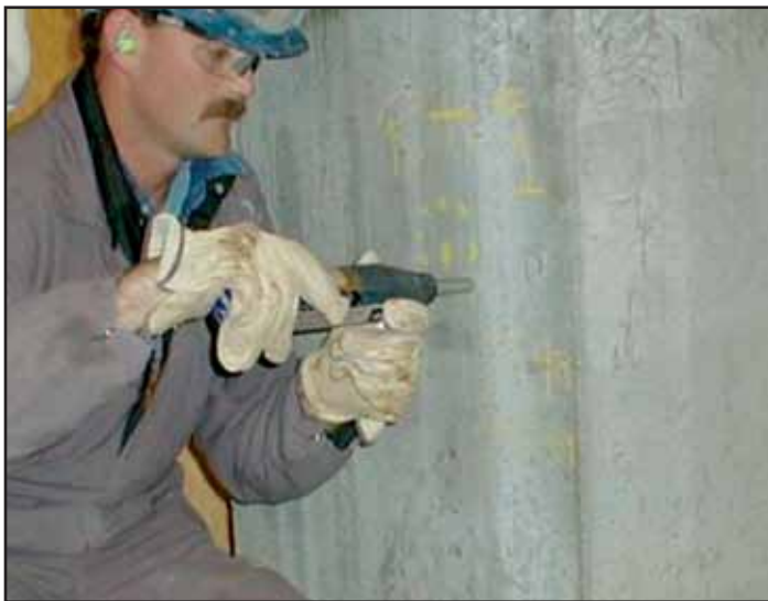
Figure No. 3 Rebound Hammer Testing for surface hardness assessment.
