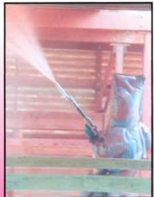
Spray Technician applying red dye colored preservative.
