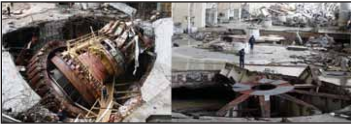
Figure 4A & 4B: Severe damage at the at the Power Station [4, 5]
