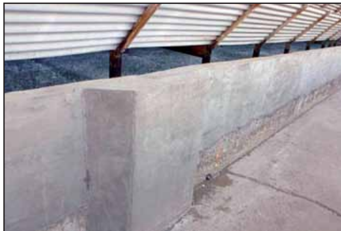
Figure No. 12 Basin Wall Formwork incorporating corrosion-resistant form-tie hardware.
