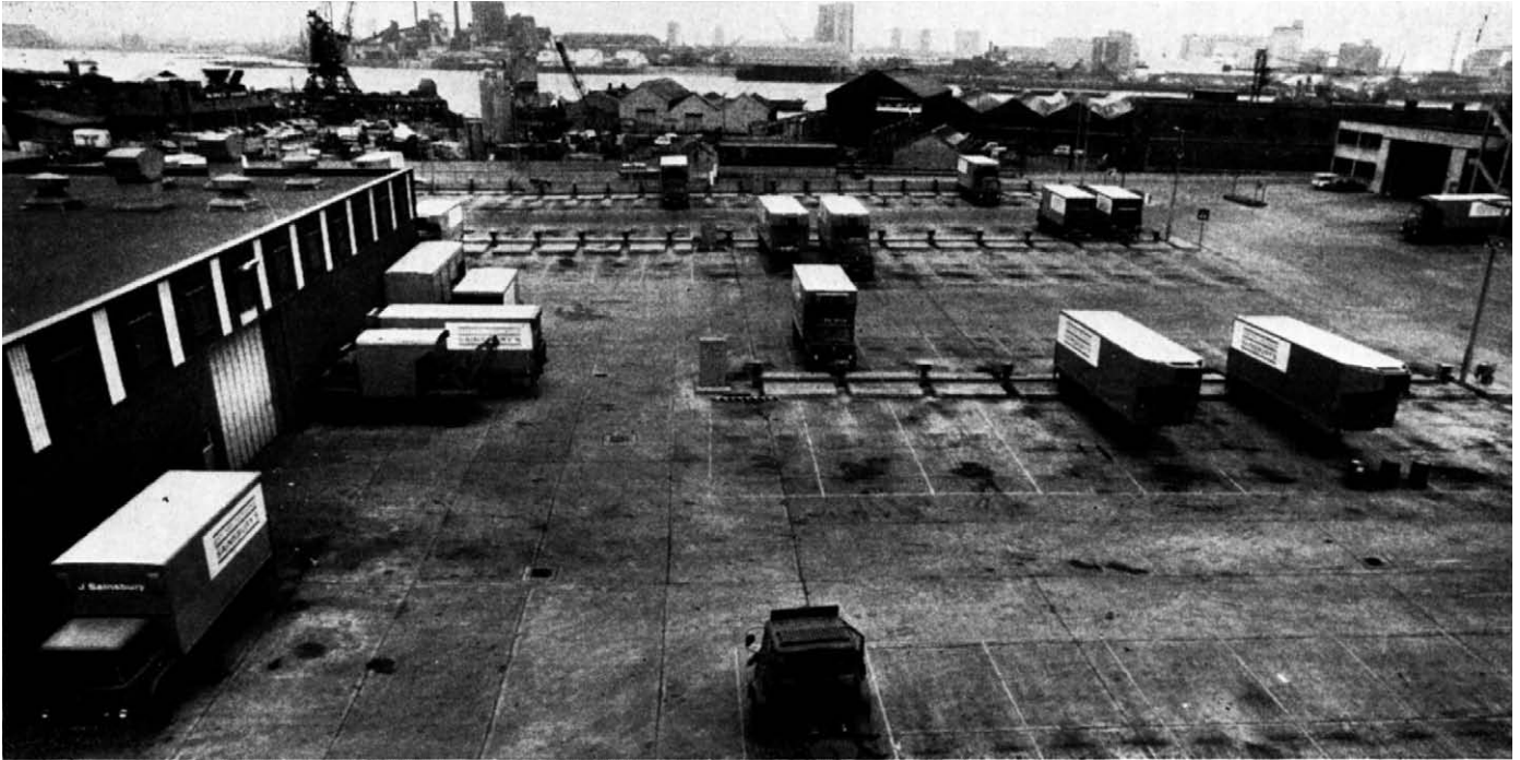
Figure 3.5 Well-planned truck park for refrigeration lorries, with plug-in positions for integral refrigeration units, clearly identified bays, and raised area to protect the plug points and allow safe personnel movement.
