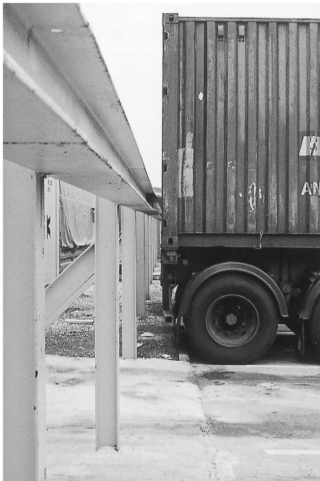
Figure 3.8 Robust barrier in parking area.
