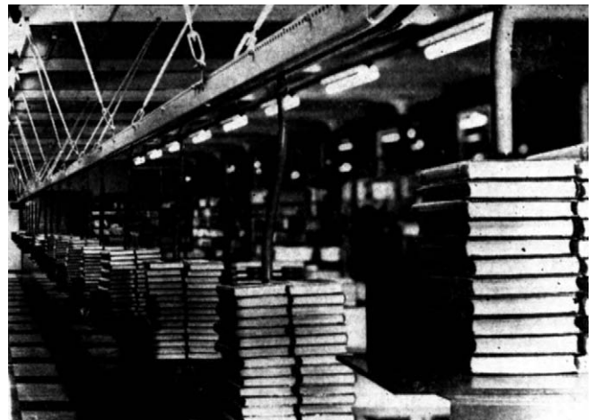
Figure 4.33 Lightweight overhead track conveyor used in book store.
