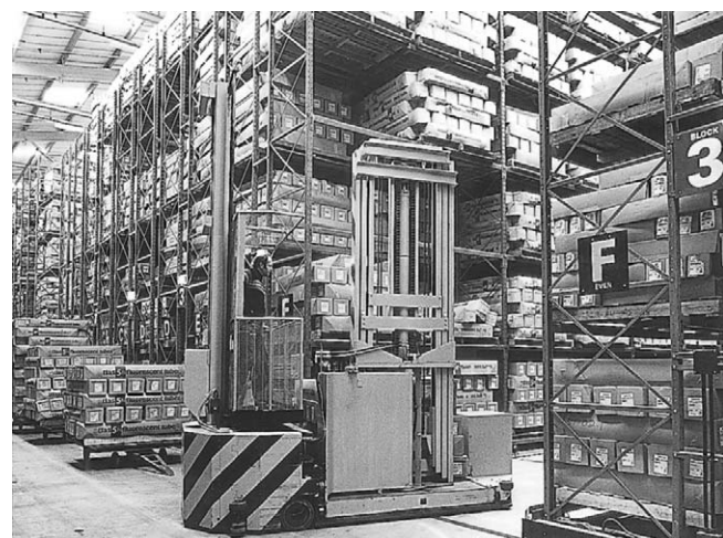
Figure 4.109 Note density of storage with mobile racking: here 1600 m 2 handles 10,000 products.
