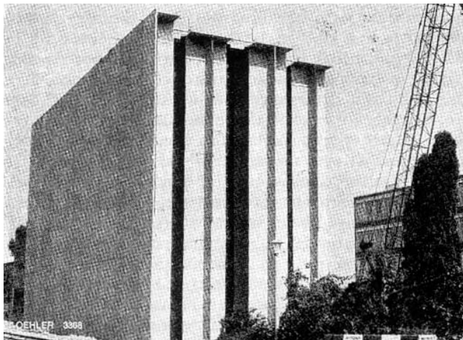
Figure 5.2 Dr Maag pharmaceutical warehouse, built from pre-cast concrete 'T' members.
