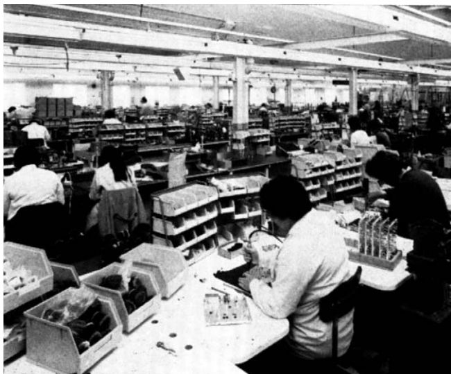
Figure 4.74 Supplies of parts in tote boxes, used in electronics industry.
