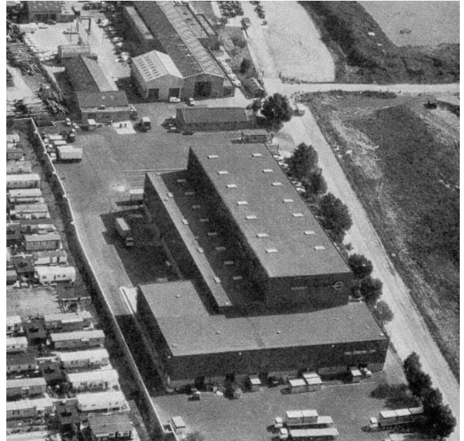
Figure 5.38 Low-rise peripheral building round high-bay pallet silo.
