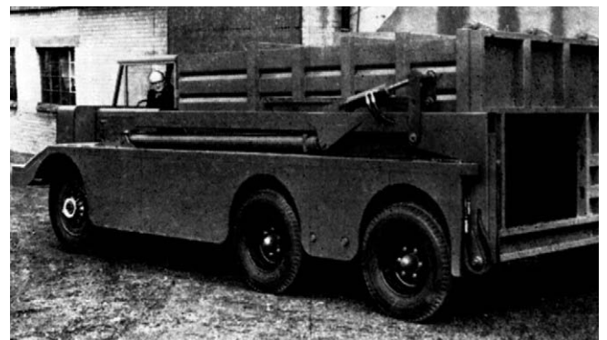
Figure 2.51 Skip collection vehicle for areas with low headroom, 3.6 m.
