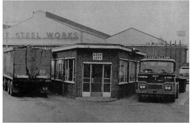
Figure 7.14 Dual weighbridge (one incoming, one dispatch) with digital read out for rapid throughput. Cycles of one minute per vehicle are possible. Note strategic siting on circulation route.
