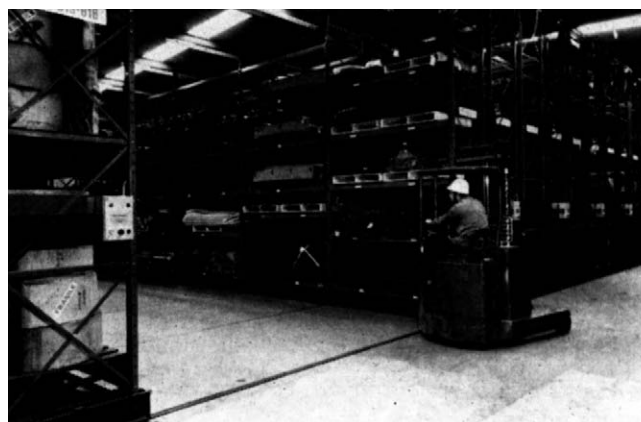
Figure 4.111 Rack opening mechanism has been operated, causing racks to open.
