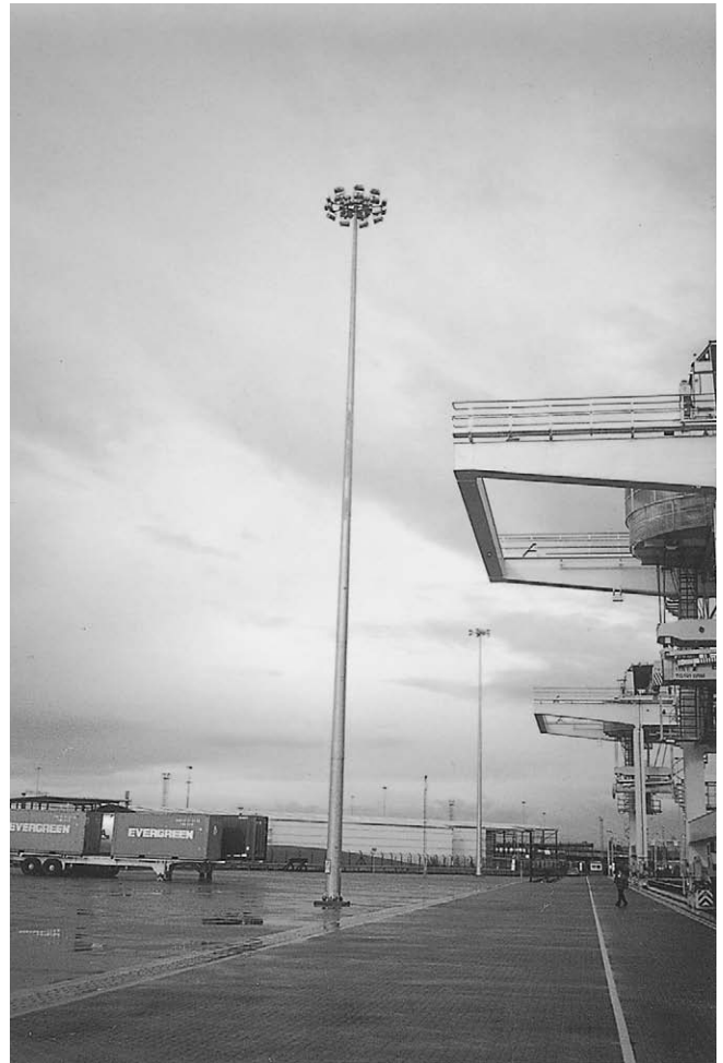
Figure 3.11 Large light tower: note also large areas required for container handling. Behind are two container cranes.
