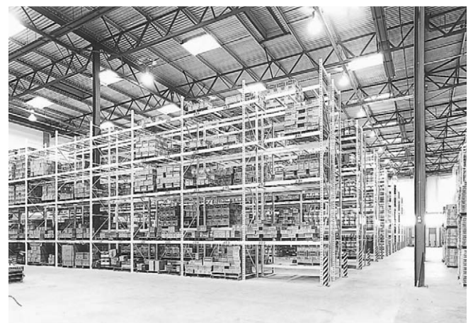
Figure 4.91 Adjustable pallet racking in use. Note clear labelling and protection bollards.
