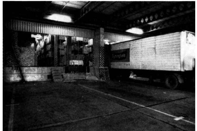
Figure 2.8 Totally enclosed loading bay. (Note structural clearances, the van at the dock is about 3.6 m high.) Note good light level without glare, clearly marked bay lines, well-painted columns to assist in reversing, extraction grill under stairs and retracted dock leveller. As usual there is a quantity of rubbish and broken pallets, as there is seldom provision in the loading area for its disposal.
