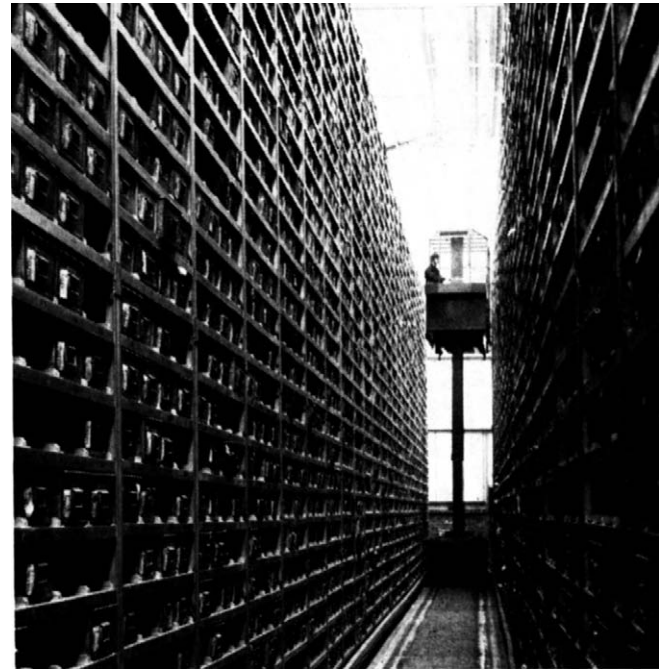
Figure 4.31 Free path order picker picking from tote boxes.
