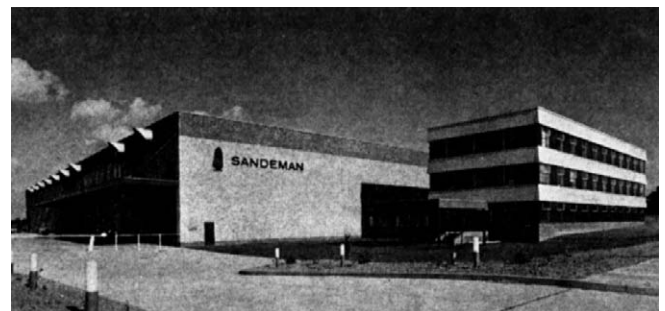
Figure 4.69 'Big box' warehouse showing adjoining office accommodation.
