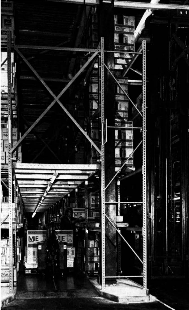
Figure 4.26 Stacking and order picking aisles arranged alternately at a warehouse in Holland, with turret truck and pallet transporter working in combination. Note how flat trusses allow maximum cube stacking, and the racking on a plinth which guides the turret truck's wheels.
