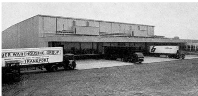
Figure 6.9 Dual-purpose loading dock in a cold store.
