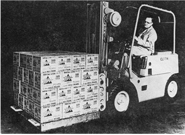
Figure 4.131 Turning fork attachment with arms set in palletized load carrying position.
