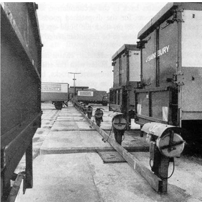
Figure 6.6 (a) A well-planned parking/plug-in area. (b) A row of double lead drum units, showing weather protection and drainage channels. The wide concrete apron with deep kerbs around the plugs prevents reversing damage.
