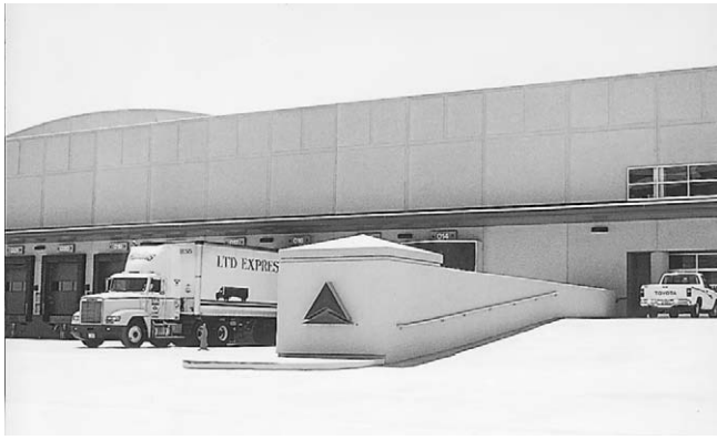
Figure 4.2 Raised loading bays with dock shelters: note ramp to warehouse floor level for small vehicles to the right.
