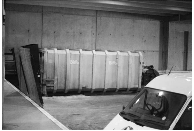
Figure 2.47 30 m skip in loading bay attached to clock-mounted static compactor.
