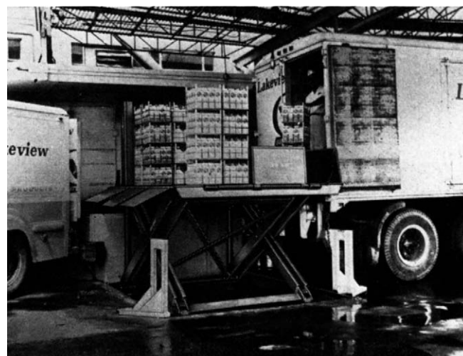
Figure 2.62 Elevating dock used where the old dock (left) is too low, and a dock leveller would reach too steep a gradient in the space available. Note raising lip to prevent wheeled dollies rolling off platform.
