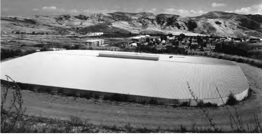
Figure 3.20 Column-supported aluminum roof with preformed sheathing, covering a water storage reservoir. (Courtesy of Temcor)
