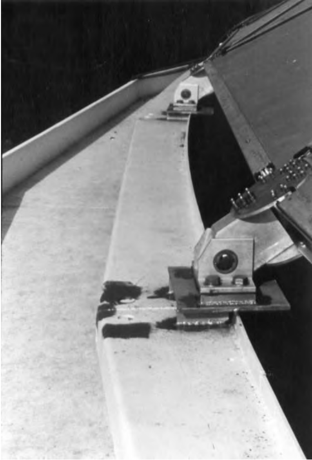
Figure 8.6 Pinned support for an aluminum dome. (Courtesy of Conservatek Industries, Inc.)
