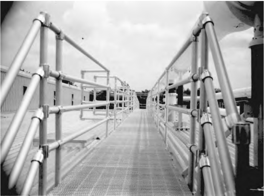
Figure 2.9 Aluminum walkway and handrail at a municipal wastewater treatment plant. (Courtesy of Conservatek Industries, Inc.)
