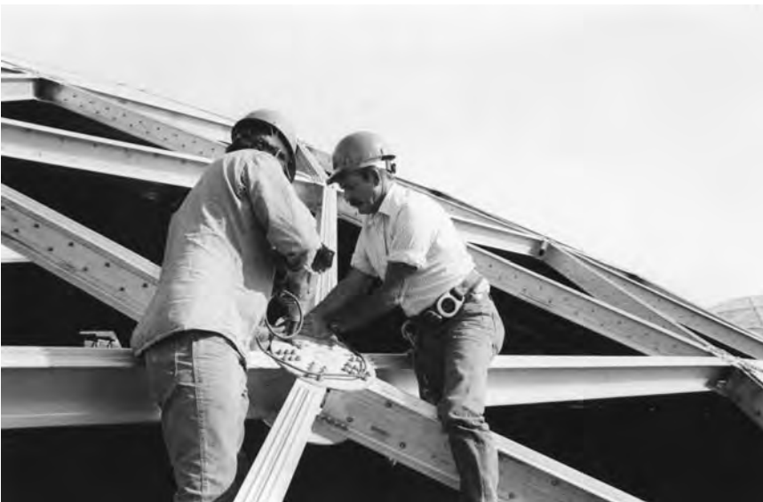
Figure 8.1 Aluminum frame with bolted connections. (Courtesy of Conservatek Industries, Inc.)
