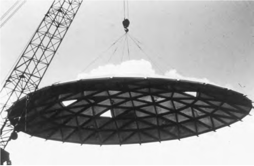
Figure 3.23 An aluminum dome being set in place with a crane. Aluminum domes as large as 190 ft [58 m] in diameter have been built alongside the structure to be covered, and then set in place in this manner. (Courtesy of Conservatek Industries, Inc.)
