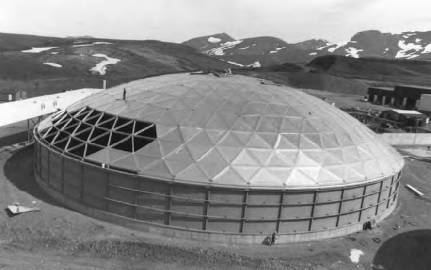
Figure 10.13 An aluminum dome under construction, partially sheeted. (Courtesy of Conservatek Industries, Inc.)
