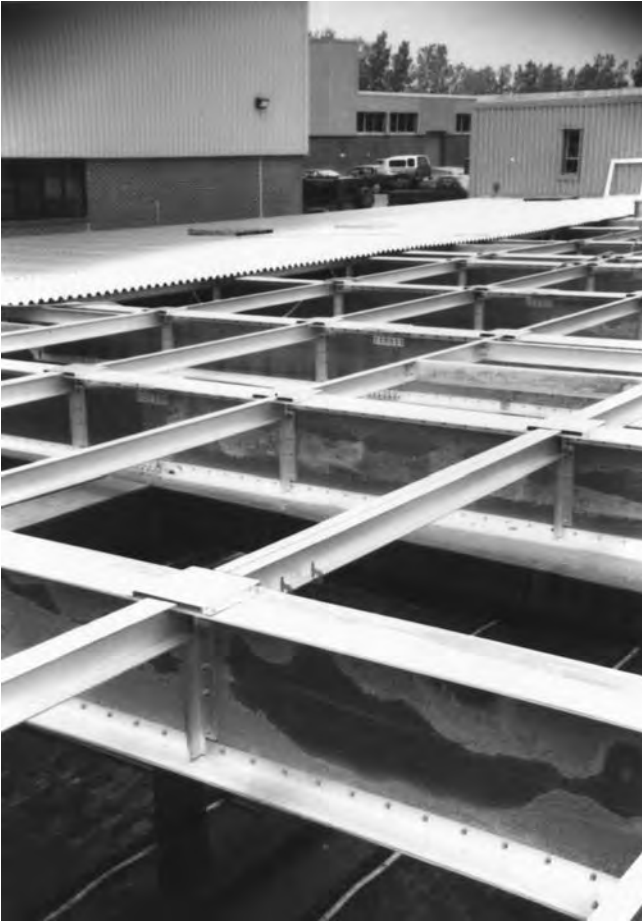
Figure 3.19 Water-stained beams in an aluminum cover. The beams will be covered by roofing panels, so the water stains pose no detriment to the structure, aesthetic or otherwise.
