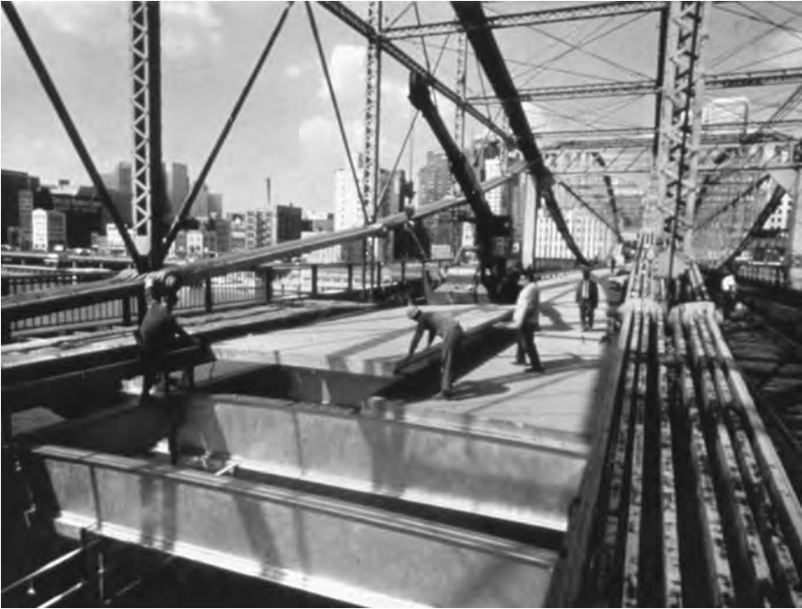
Figure 2.2 Installation of an aluminum deck on aluminum beams for the Smithfield Street Bridge in Pittsburgh, Pennsylvania. (Courtesy of Alcoa)
