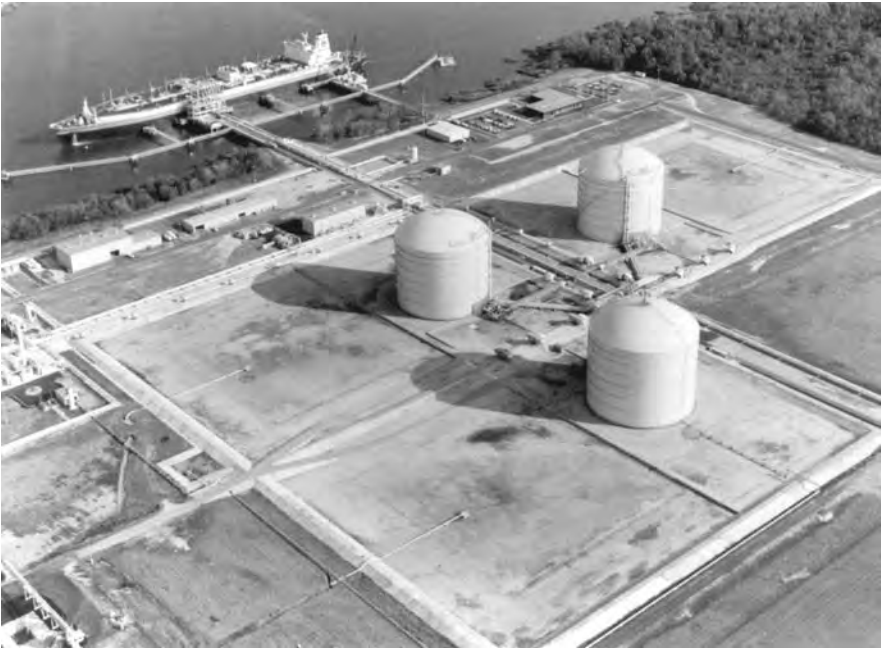
Figure 2.7 Double-wall cryogenic tanks storing liquified natural gas at -260^{\circ}\text{F} [ -160^{\circ}\text{C} ]. The inner tanks are aluminum. (Courtesy of Chicago Bridge & Iron)
