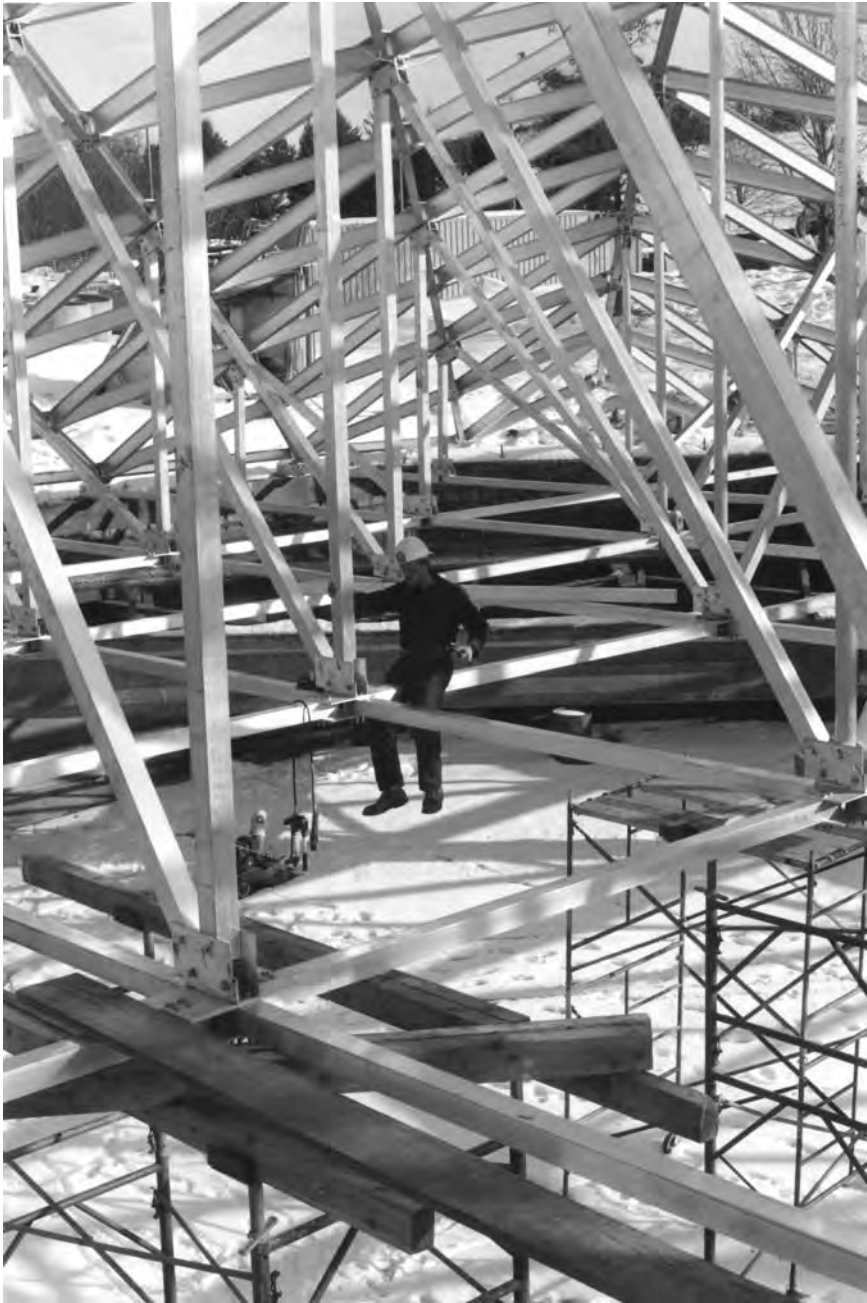
Double-layer aluminum space frame under construction. This is one of the two structures pictured in Figure 2.3. (Courtesy of Conservatek Industries, Inc.)
