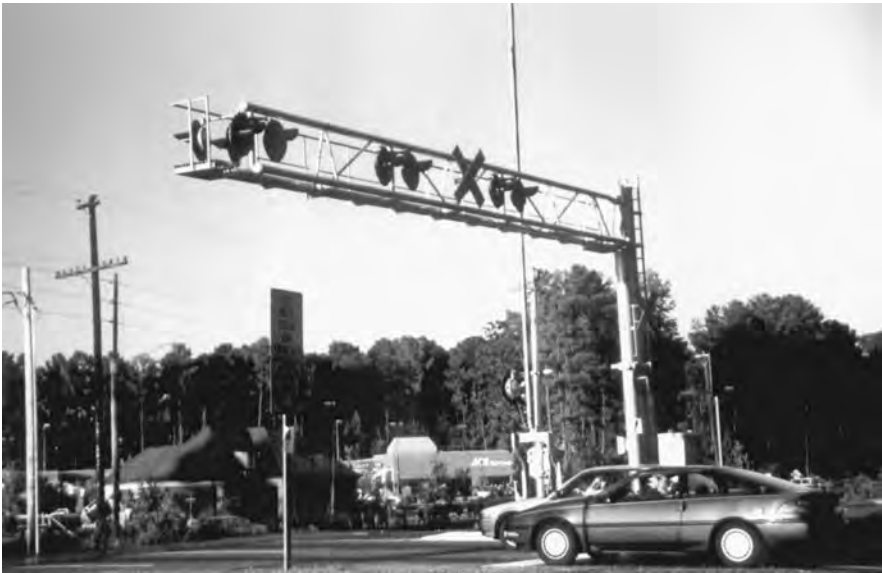
Figure 2.10 Aluminum structure supporting a highway sign at a railroad crossing.
