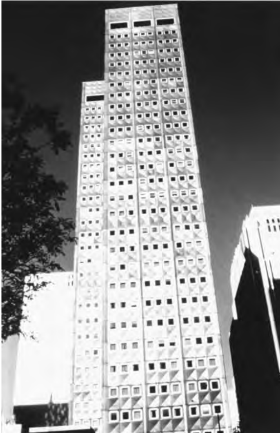
Figure 2.5 Aluminum curtain wall on the Alcoa Building. (Courtesy of Alcoa)
