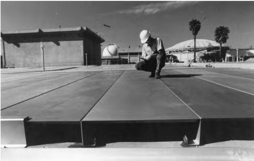
Figure 10.7 Cold-formed sheet beams. (Courtesy of Temcor)
