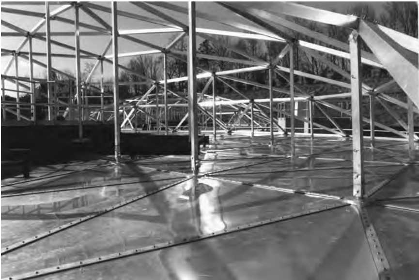
Aluminum space frame with a suspended aluminum deck. (Courtesy of Conservatek Industries, Inc.)
