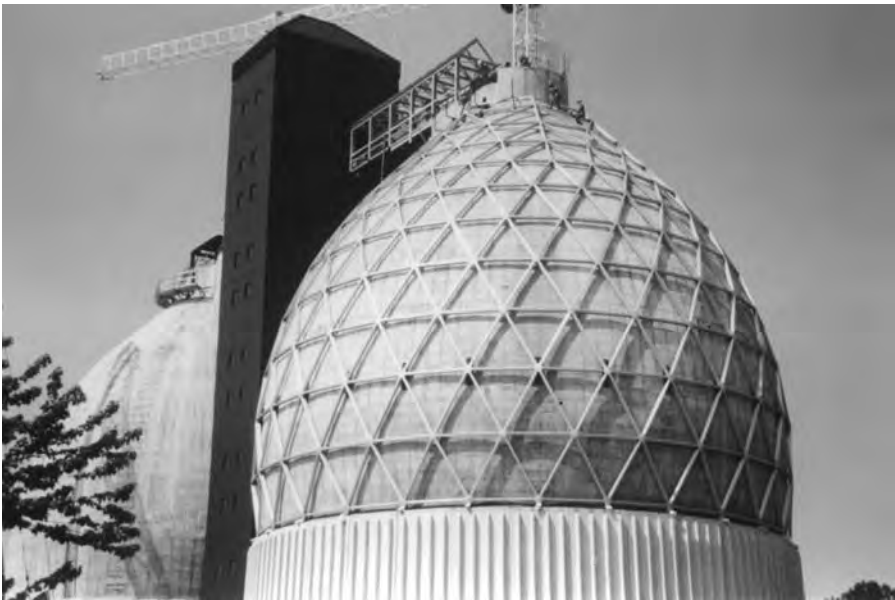
Figure 5.68 The framing for a custom, curved cladding system will undoubtedly be subject to combined shear, compression, and bending. (Courtesy of Temcor)
