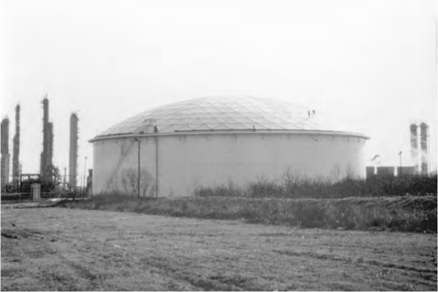
Figure 2.8 Clear-span aluminum dome covering a petroleum storage tank. (Courtesy of Conservatek Industries, Inc.)
