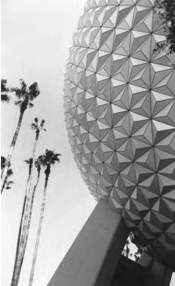
Figure 3.22 Aluminum-clad panels cover the sphere at the entrance to Walt Disney World's EPCOT Center in Florida.
