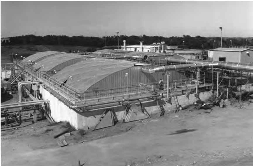
Aluminum barrel vault covers. (Courtesy of Koch Refining Co.)
