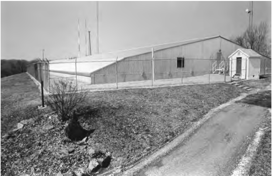
Truss-supported aluminum cover. (Courtesy of Conservatek Industries, Inc.)
