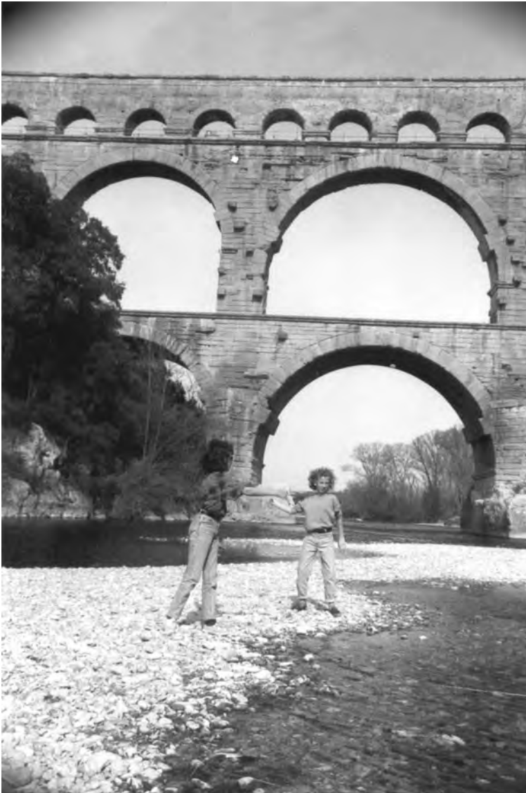
Figure 2.1 Pont du Gard in southern France. An aqueduct that the ancient Romans built by skillfully stacking stones.
