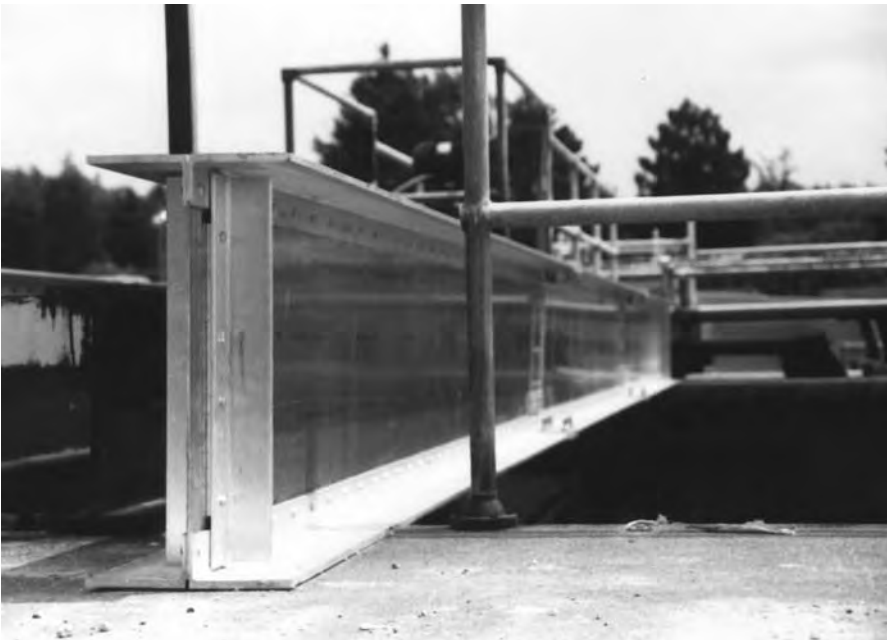
Figure 5.40 A built-up aluminum beam. (Courtesy of Conservatek Industries, Inc.)
