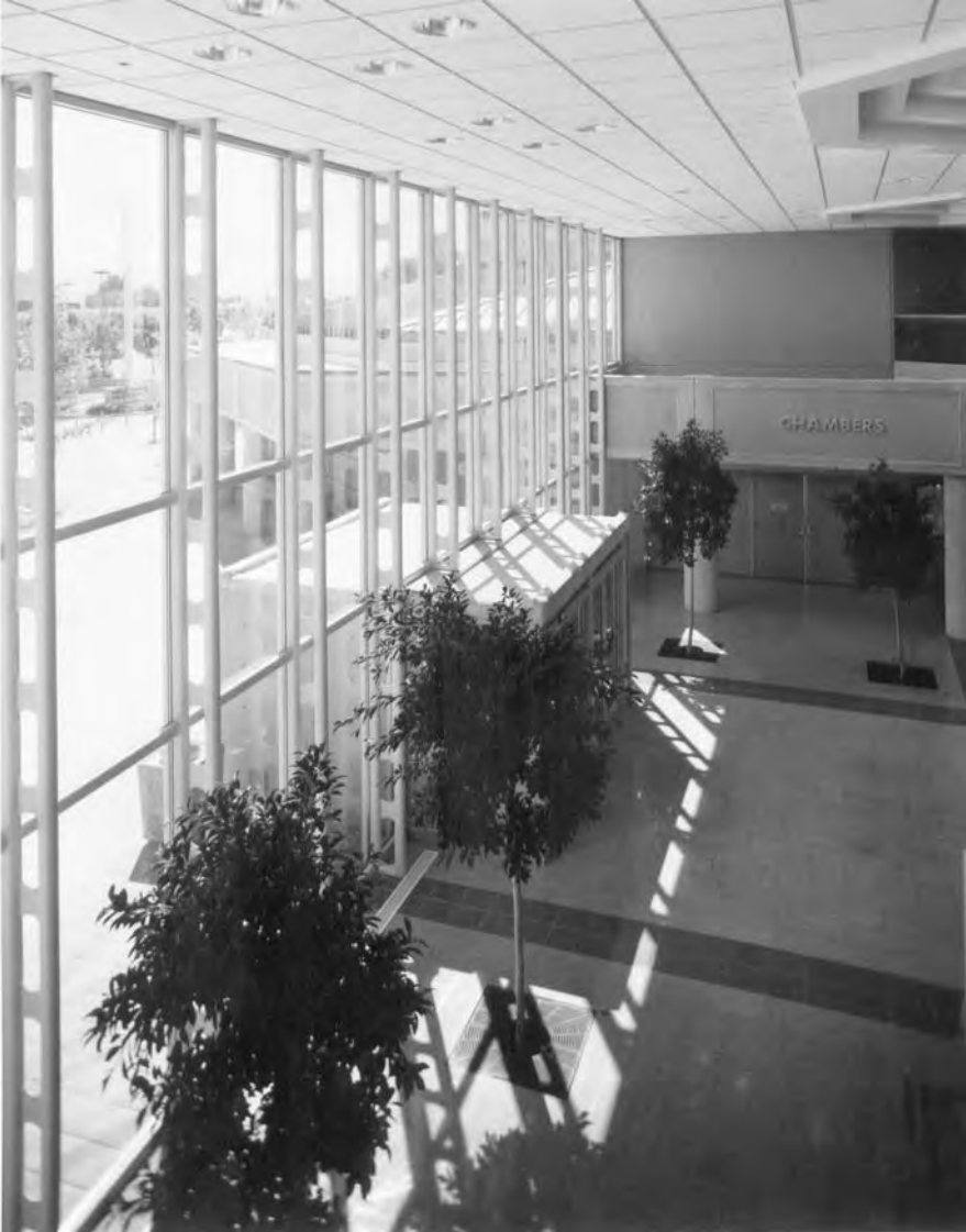
Figure 2.6 Custom-extruded aluminum framing supporting a glass wall. (Courtesy of Kawneer)
